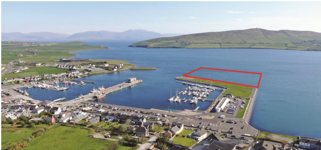
Figure 2. Looking south toward the proposed extension area (red) for the existing Dingle port and marina, Dingle Harbour, February 2021.
