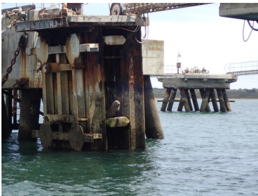
Figure 24, Seal at Crib Point Jetty 2019
