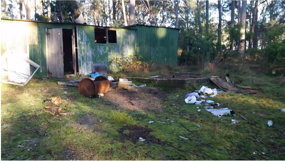
Plate 2: Corrugated iron structures and rubbish in the DAD in the south west of the study area
