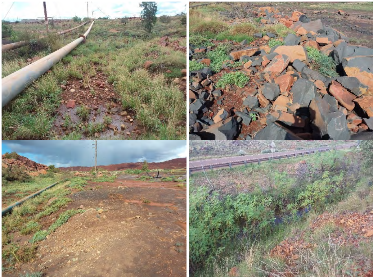
Plate 1 Evidence of disturbance from top right clockwise: pipeline, man-made rock wall, roadside drainage, earthworks
