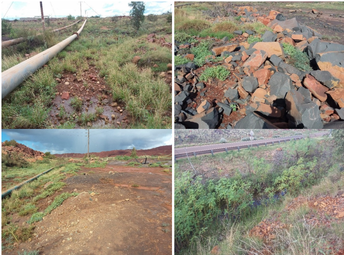
Plate 1 Evidence of disturbance from top right clockwise: pipeline, man-made rock wall, roadside drainage, earthworks
