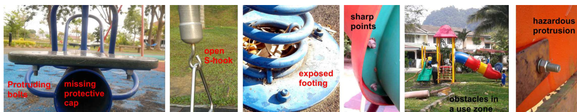
Figure 4. Examples of observations detecting general hazards
