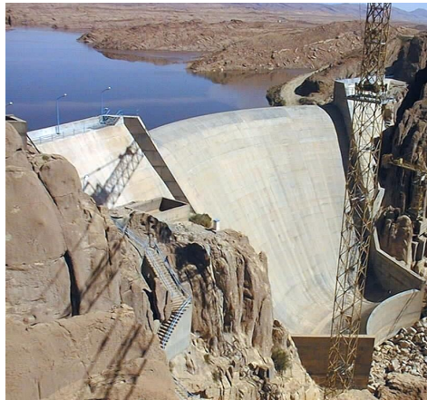
Figure 1. Brezina concrete arch dam
