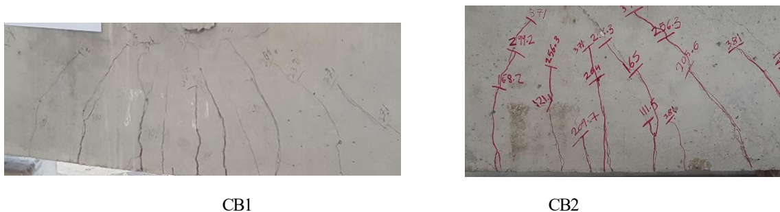
Figure 6. Pure Flexural Failure of CB1 and CB2 at Ultimate Load Capacity
