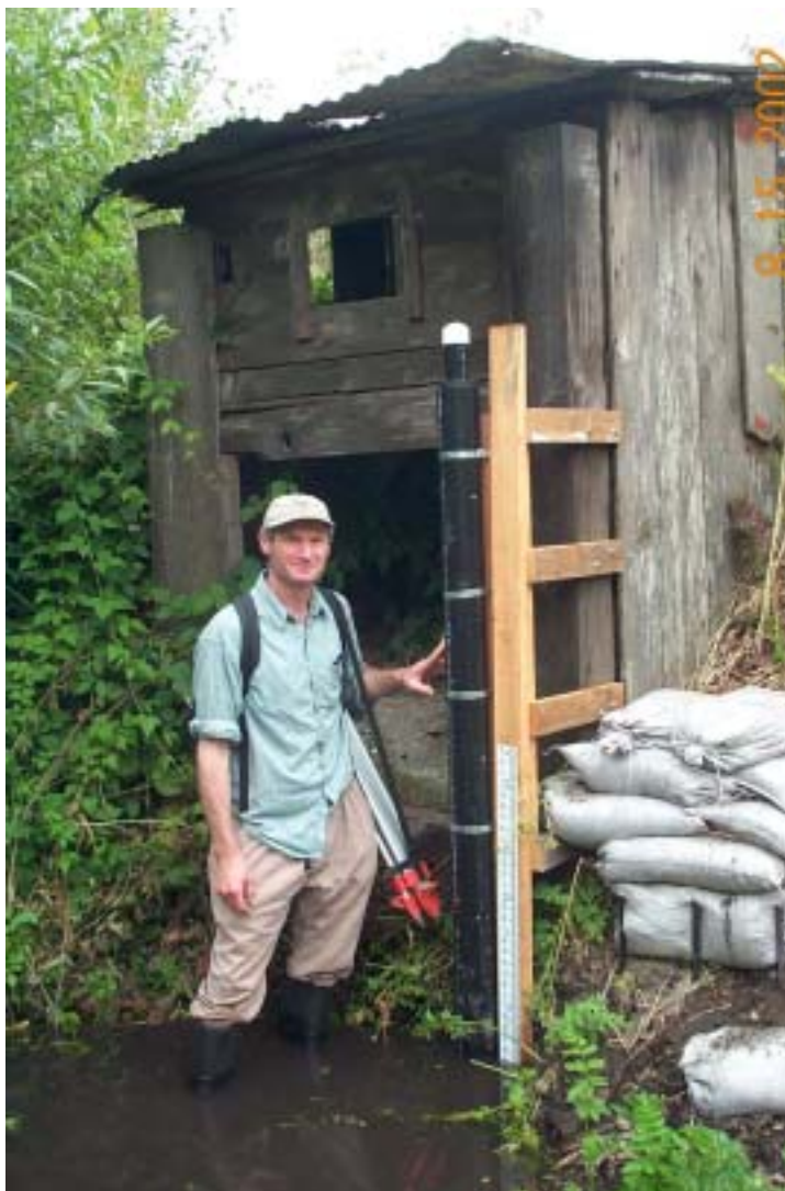
Figure 4. The Ferrari Creek staff gauge and stilling well are located to the west of Highway 1 in the location of the recently removed dam.
