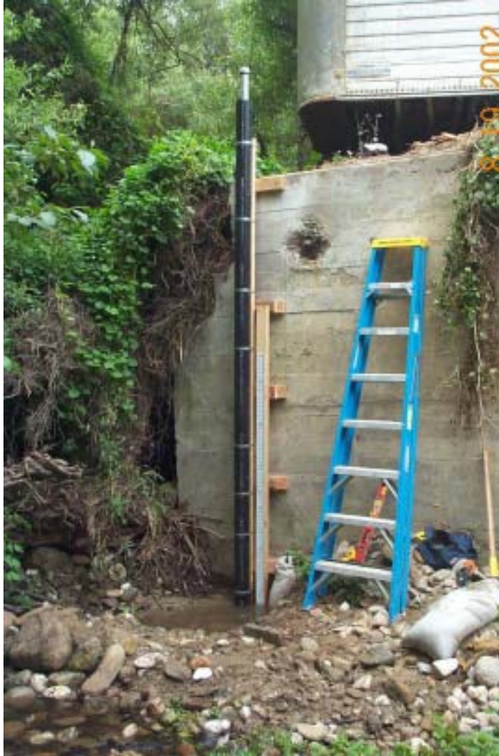
Figure 6. The San Vicente stilling well and staff gauge are located about 100 feet downstream of the diversion.
