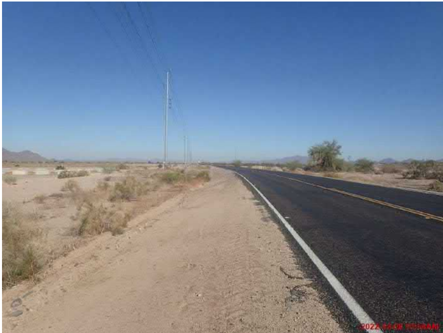
View from the southern portion of the project limits looking north along Old US 80. Note existing transmission lines.
