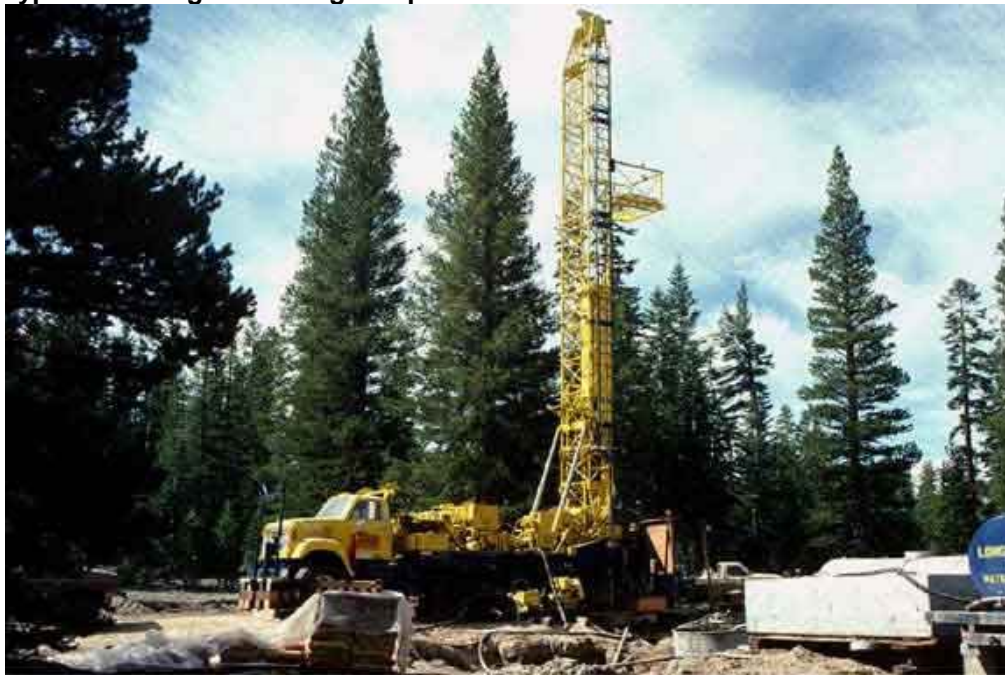
Figure 1. Typical Drill Rig for Drilling Temperature Gradient Wells
