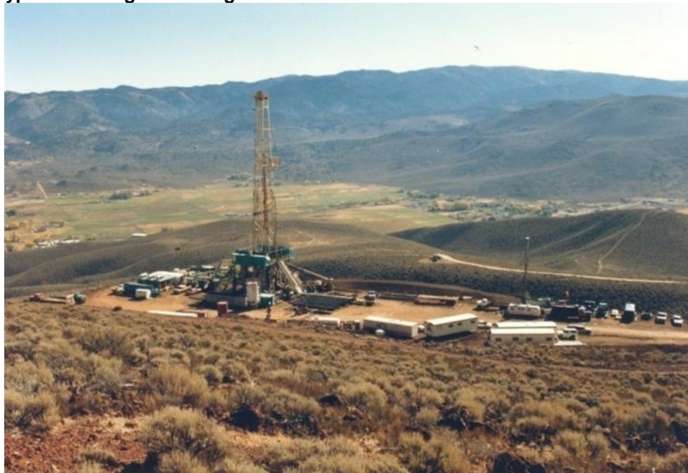
Figure 2. Typical Drill Rig for Drilling Production Wells
