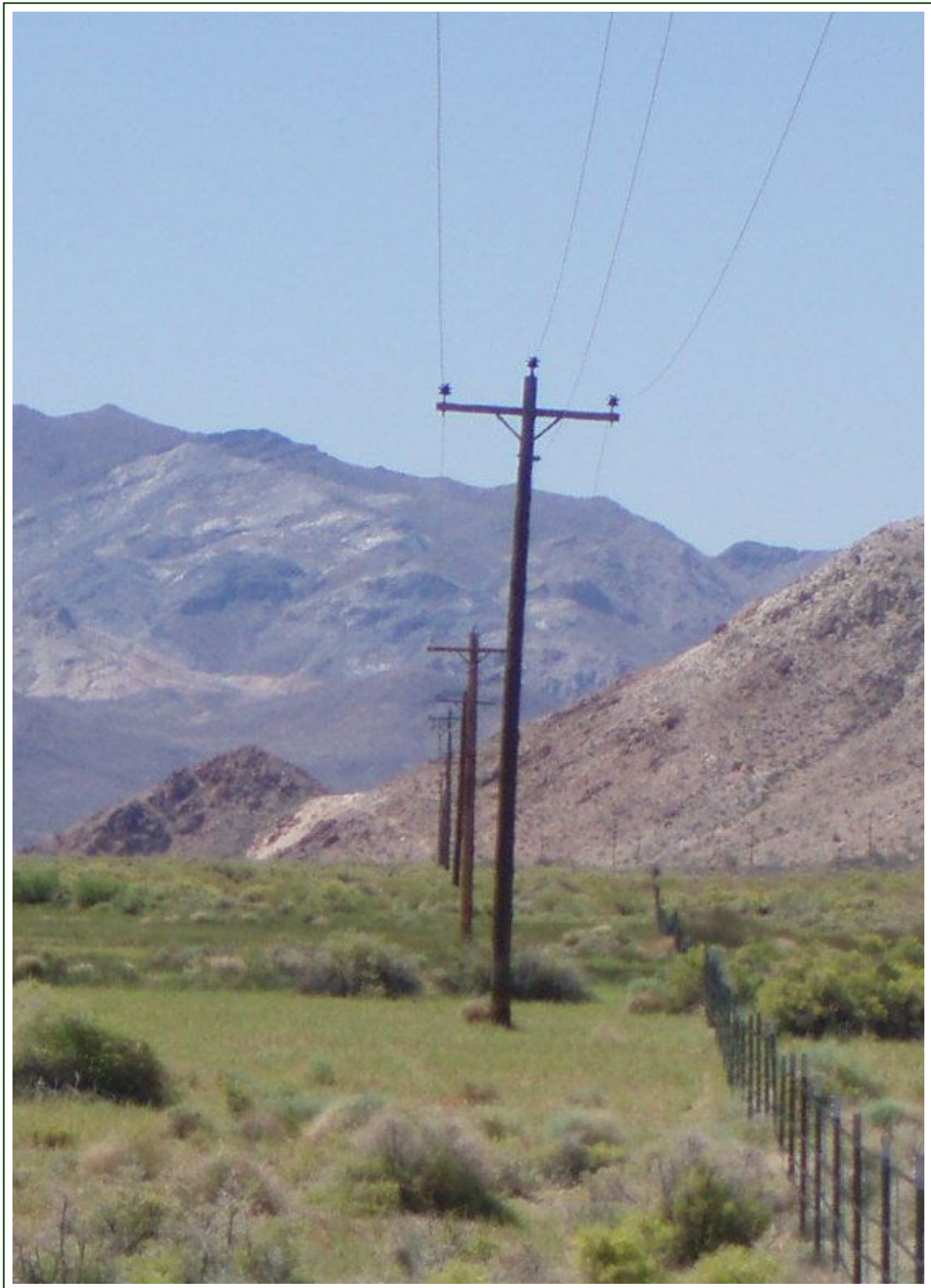
Photo 2. Typical single poles. These would be used from Beatty to Lida Junction.
