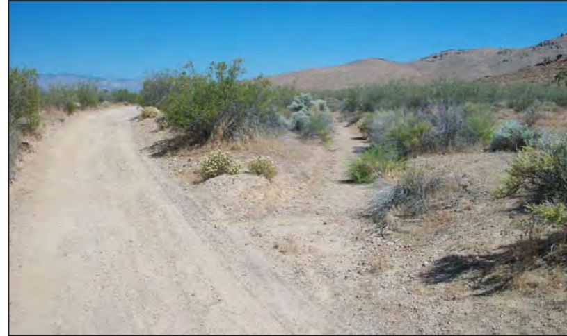
Photo 2 - View of drainage facing northeast. Feature exits natural channel and enters road at this location.
