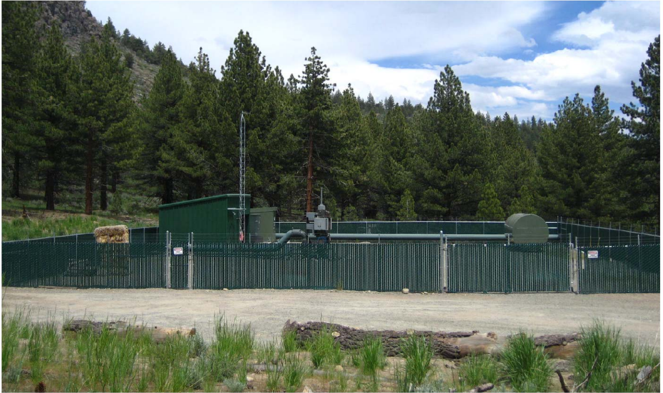
Photo 3: View of well facility 66-25 looking north from Pole Line Road.
