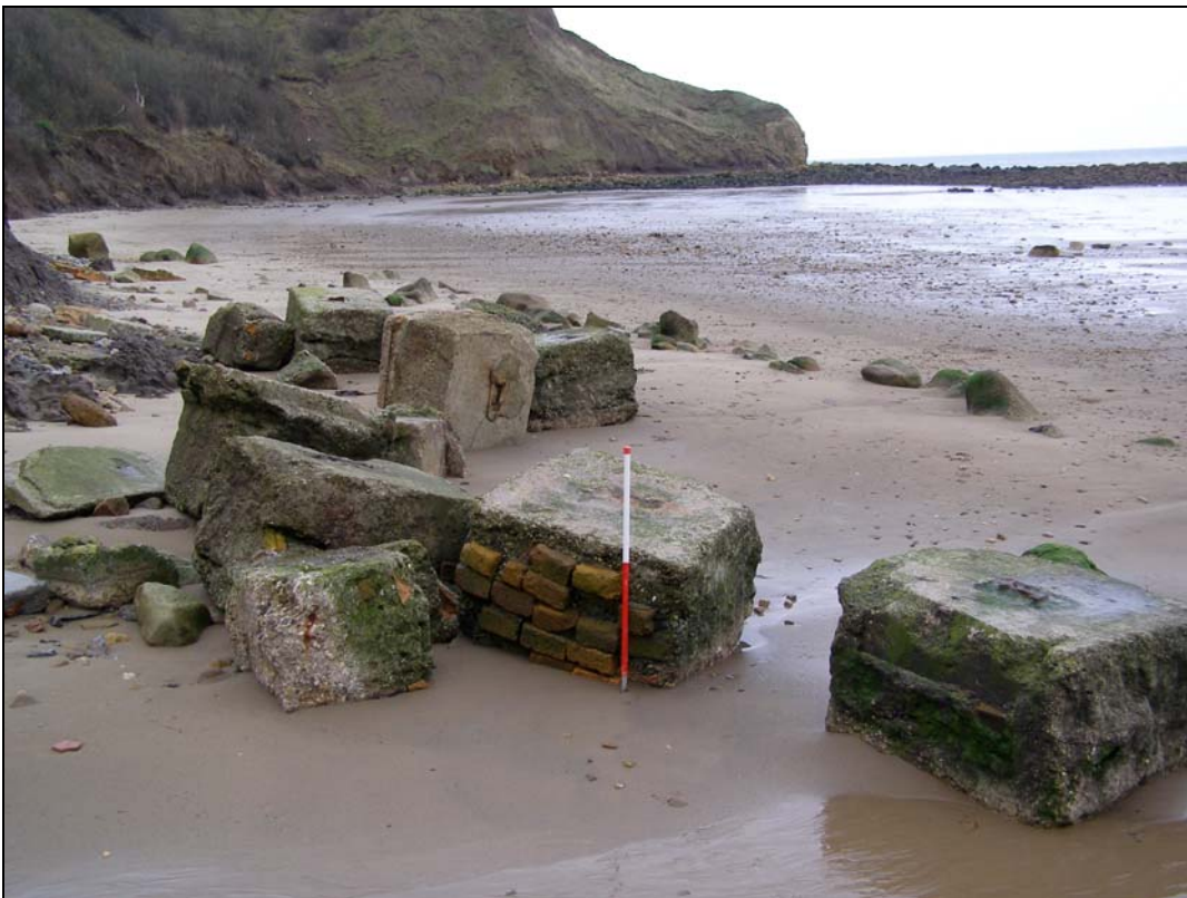
Plate 41: The surviving Second World War defensive concrete blocks on Cayton Bay Beach (OAN 160/266)
