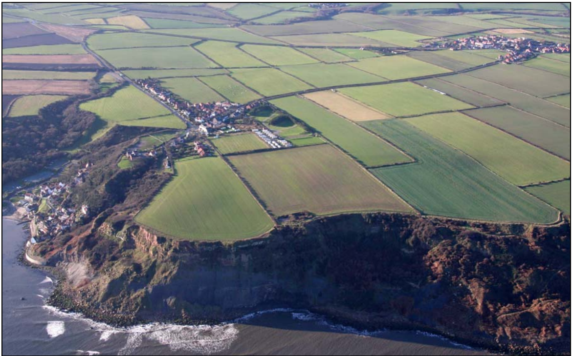
Plate 22: View of the Post-Landslip Ground Conditions at Victoria Ironstone Mine, Runswick Bay (OAN 78)
