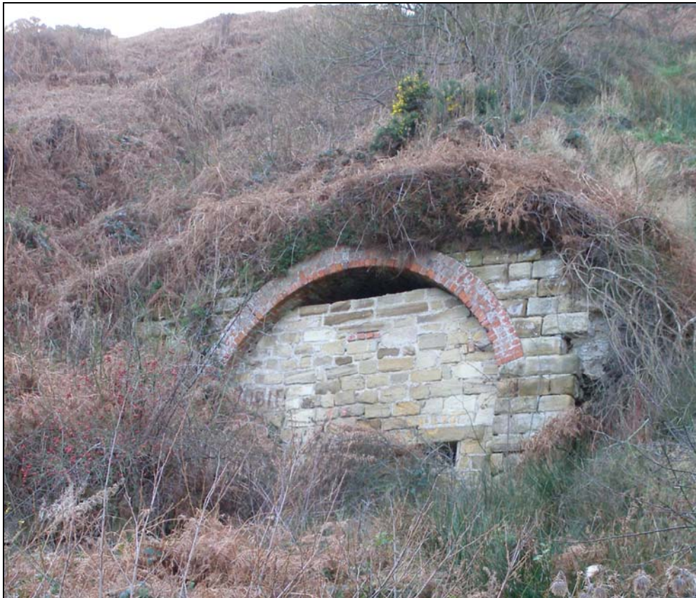
Plate 20: The Surviving Remains of the Tunnel Mouth at Port Mulgrave (OAN 194)
