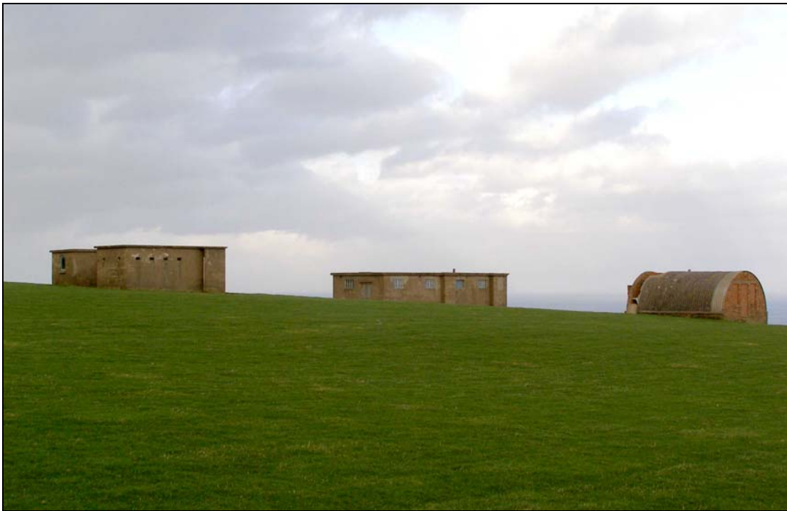
Plate 37: Part of the surviving remains of Bent Rigg Radar Station, Staintondale (OAN 6)
