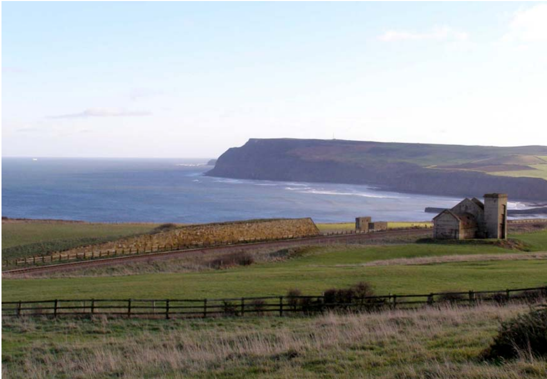
Plate 9: View of the Surviving Surface Remains at Huntcliff Ironstone Mine, Warsett Hill (OAN 54)
