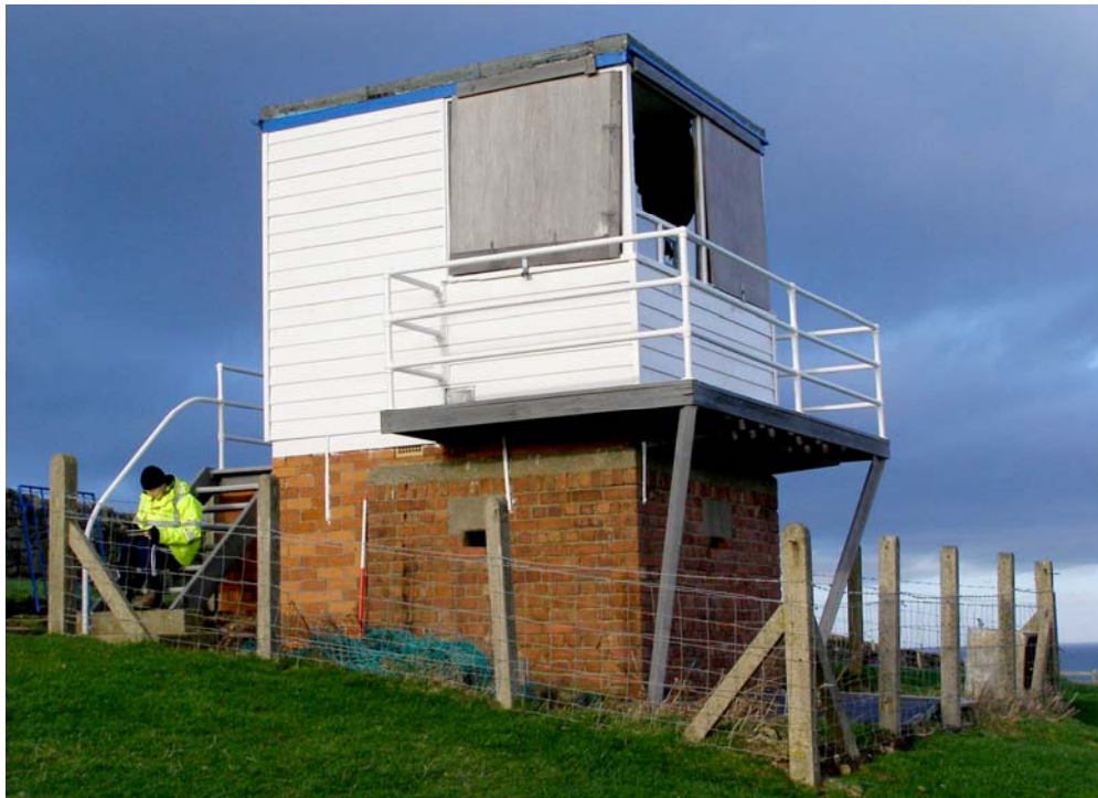
Plate 28: View of the Coastguard Lookout Point at Robin Hood's Bay (OAN 185)
