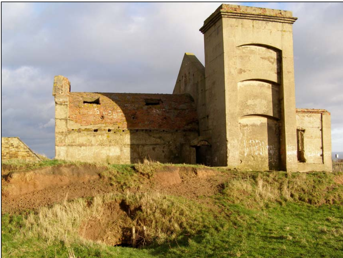
Plate 10: Erosion to the Tunnel Vaulting and General Survival of the Guibal Fanhouse at Huntcliff Ironstone Mine, Warsett Hill (OAN 152)
