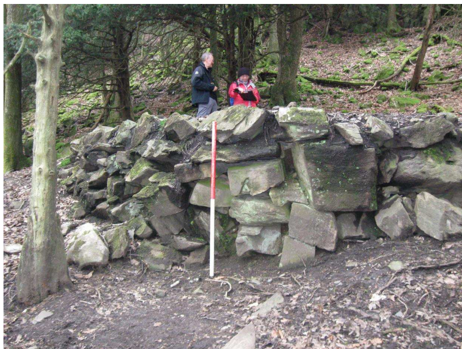
Plate 19: Detail of the large-scale stone revetment that retained a charcoal-burning platform at Summer House Knott (SMK 1003)
