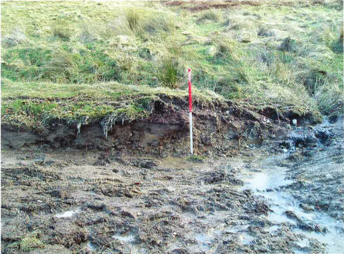
Plate 9: Typical damage to the edges of the Askham Fell Bridle Way
