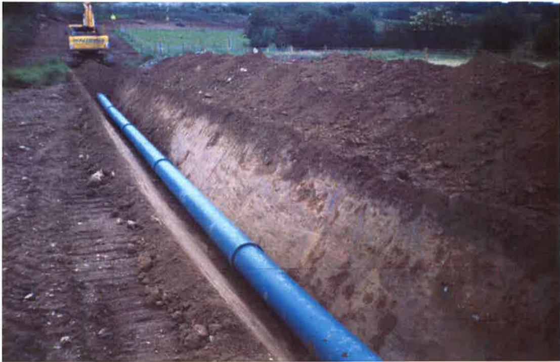
Plate 5: Laying of pipe in Watching Brief Area D
