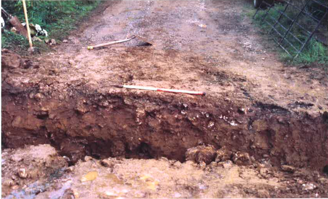
Plate 7: Excavation through trackway on the line of the putative Roman road, Area F
