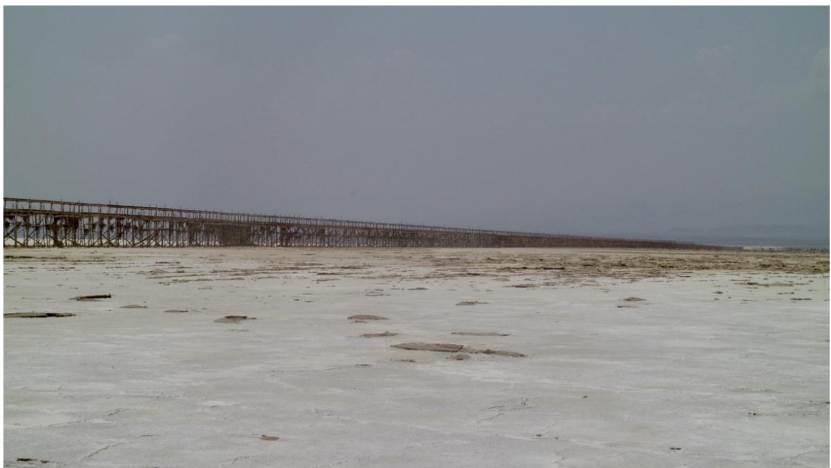
Image 20: Wooden aqueduct like construction to bring fresh water onto the salt flats (photo: TJFT, August 2018)
