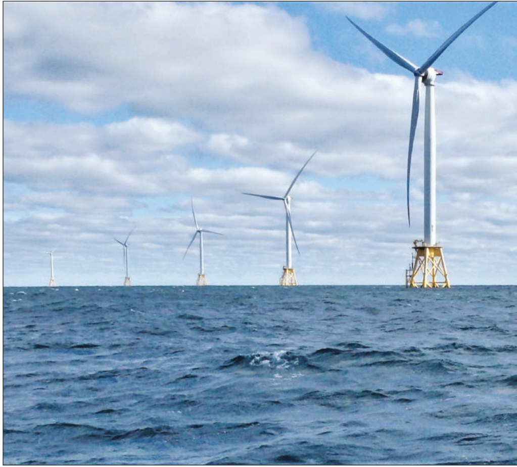
The Block Island Wind Farm.
