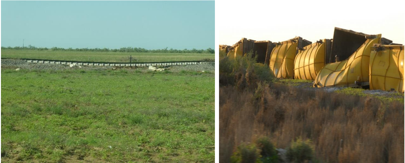
Figure 38a, 38b. Railway line damage near Julia Creek and a train carrying lead and zinc from Mt Isa to Townsville rolled over after erosion of the line ballast at Nelia.
