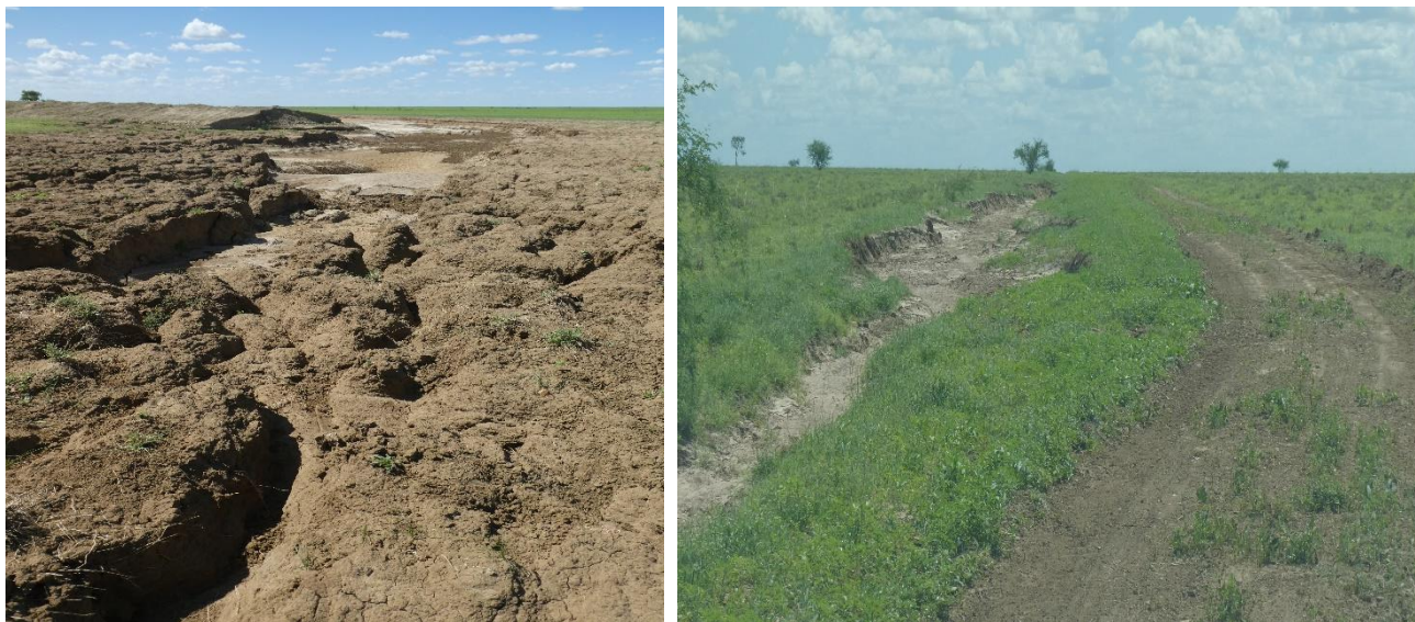
Figure 39a, 39b. (a) Dam bank and by-wash destroyed by flood waters, and (b) a property road washed out with a new adjacent track graded on the Downs south of Julia Creek.
