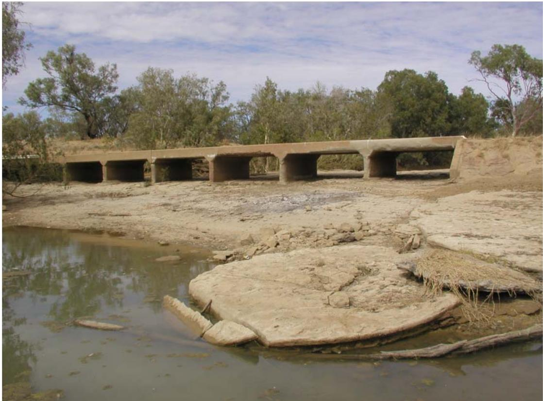
**Plate 13** Punchbowl crossing on the Flinders River has good-sized culverts that would not restrict fish passage.
