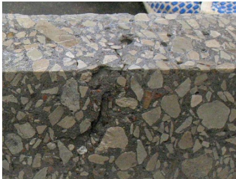
Figure 17. Eppley Core 3 after 70 cycles, showing a circumferential crack at least partially affected by subsurface voids. The arc-shaped damage feature in the lower center is a spall over a subsurface void that is fracturing off.
