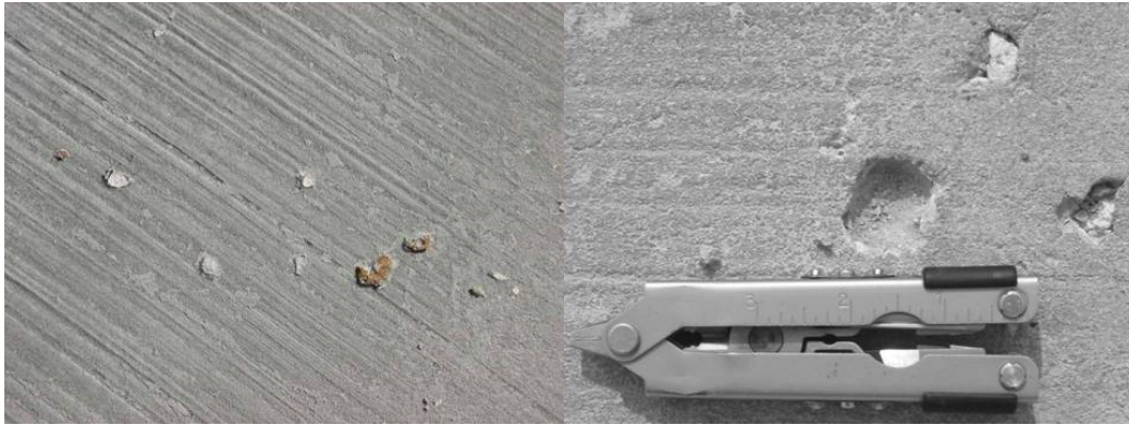
Figure 6. Examples of popouts: (left) Laughlin AFB, TX; (right) Middle Eastern airbase
