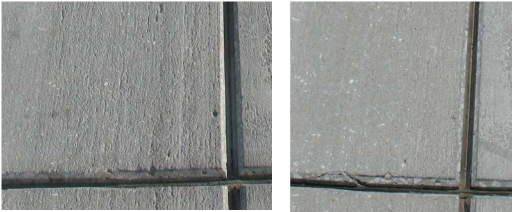
Figure 55. Loss of surface paste and formation of a new spall. Condition in December 2007 is on the left, and condition in June 2008 is on the right.
