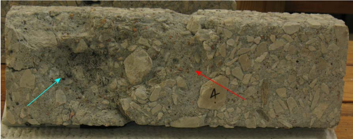
Figure 19. A specimen from Eppley Field after 230 cycles. The red arrow points to a zone of concrete that is deficient in coarse aggregate and probably also air. The blue arrow points to a deeply damaged zone that started as damage from a 10 mm entrapped air void and later enlarged, apparently due to paste damage. Note that the concrete, and specifically the paste, on the right-hand end of the specimen is in good condition.
