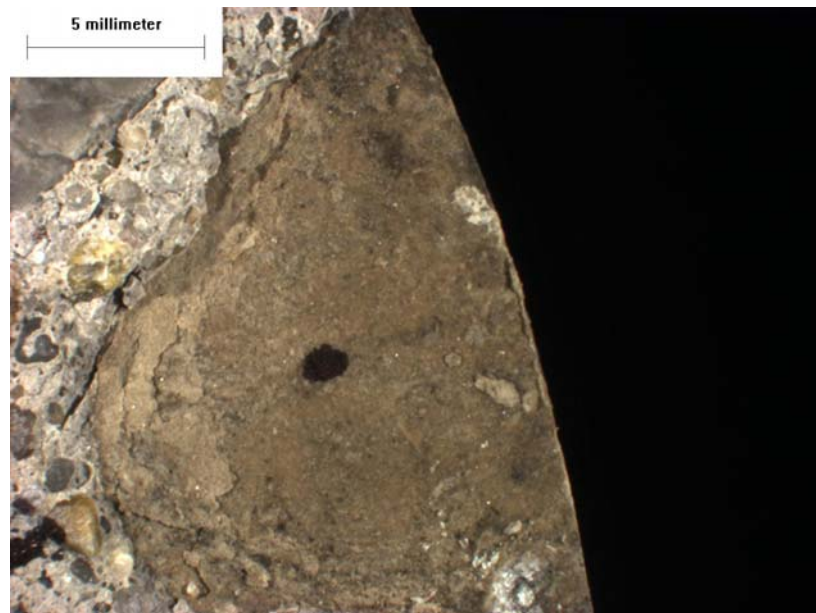
Figure 36. An example of paste etching and aggregate damage (along the left edge) after 19 cycles of freezing and thawing in water after exposure to potassium acetate.
