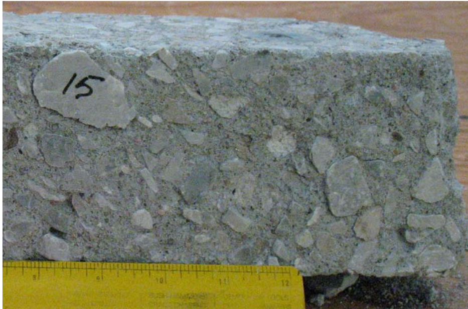
Figure 21. This photograph shows the same area of sample 15 shown in Figure 20, after 230 cycles. The paste is still largely intact, as indicated by the still relatively sharp edges, although the aggregate is clearly undercut due to loss of cement paste.
