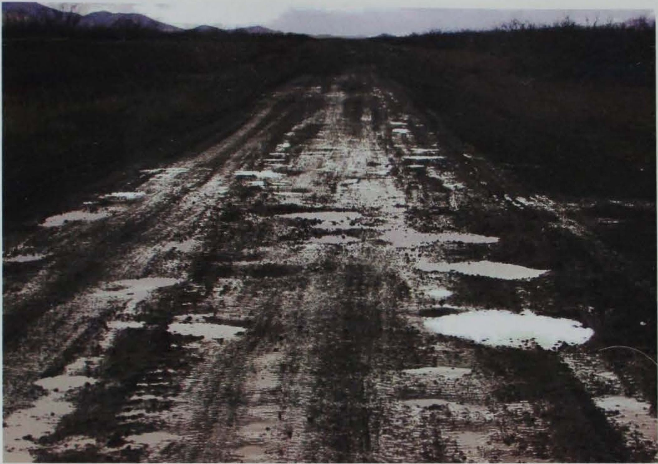
Photo 1. Initial road surface condition
