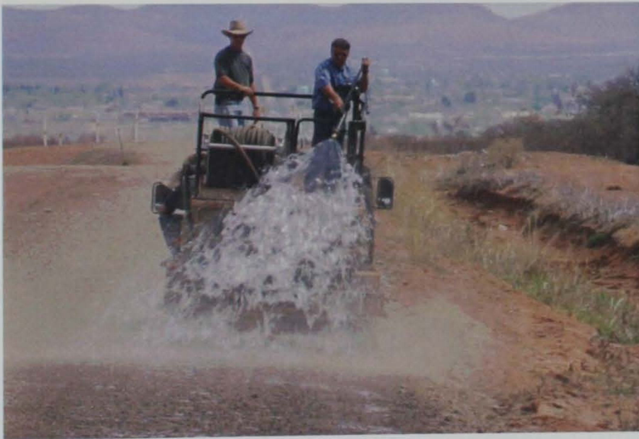
Photo 34. Spraying of high viscosity Blue Goo® solution with hand wand
