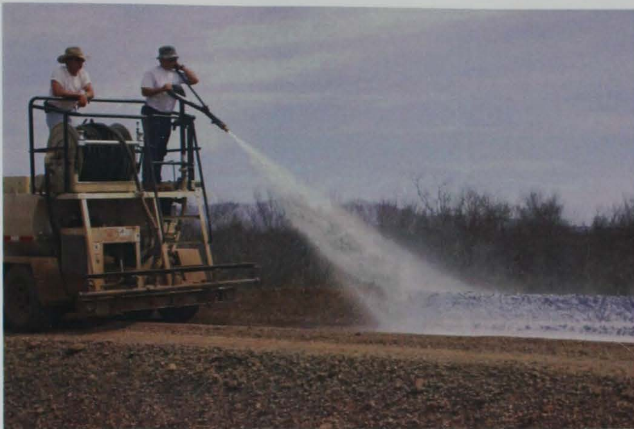
Photo 13. Spraying product on windrows using hand wand
