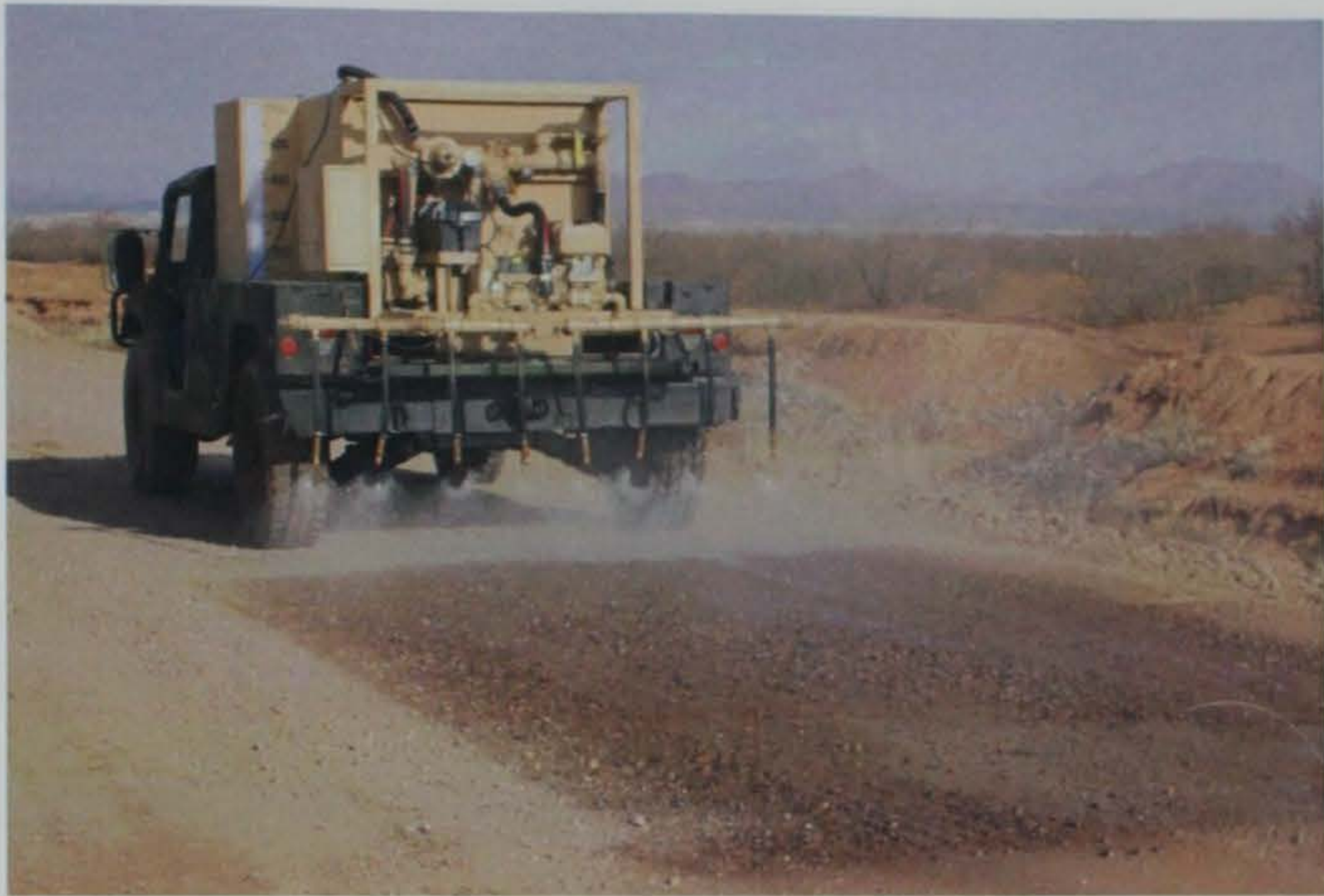
Photo 29. Applying Envirokleen® to transition areas with spray boom
