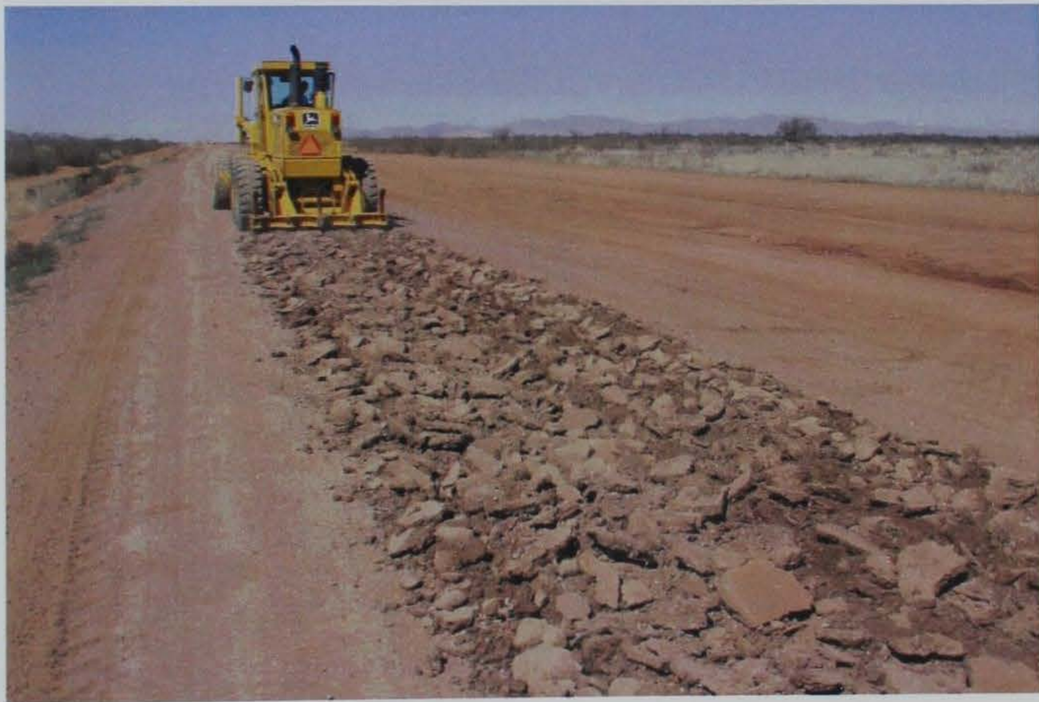
Photo 2. Breaking of surface and grading prior to test section construction
