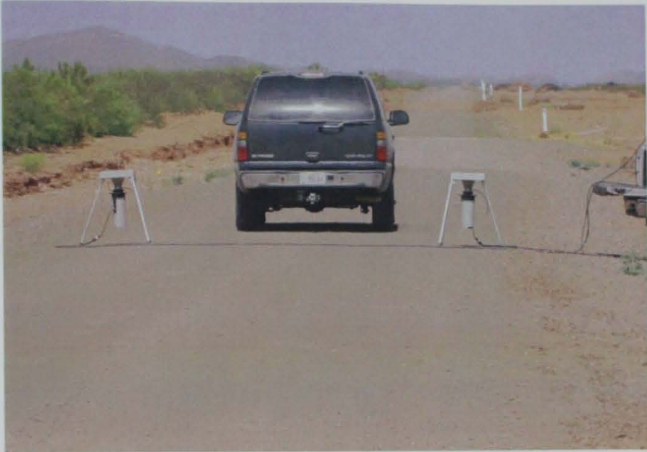
Photo 45. Excellent performance of Envirotac II® on Section 18
