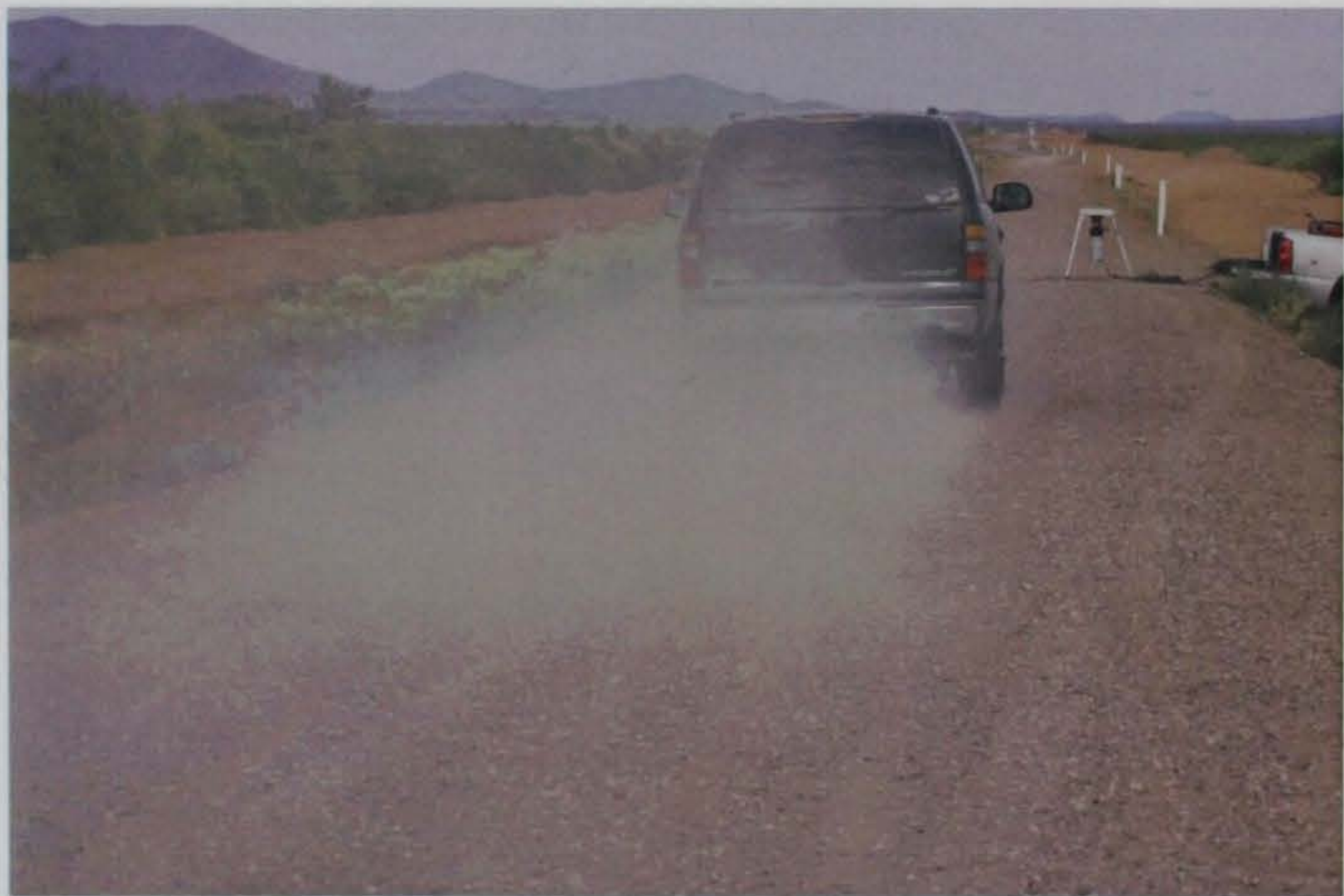
Photo 40. Dust collection on Section 12, Blue Goo®
