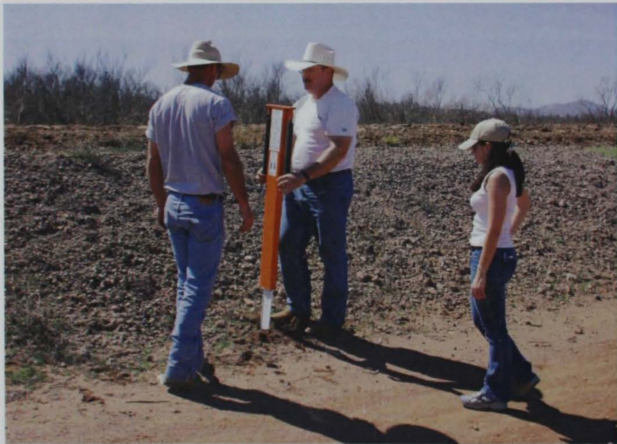
Photo 4. Placement of traffic delineators
