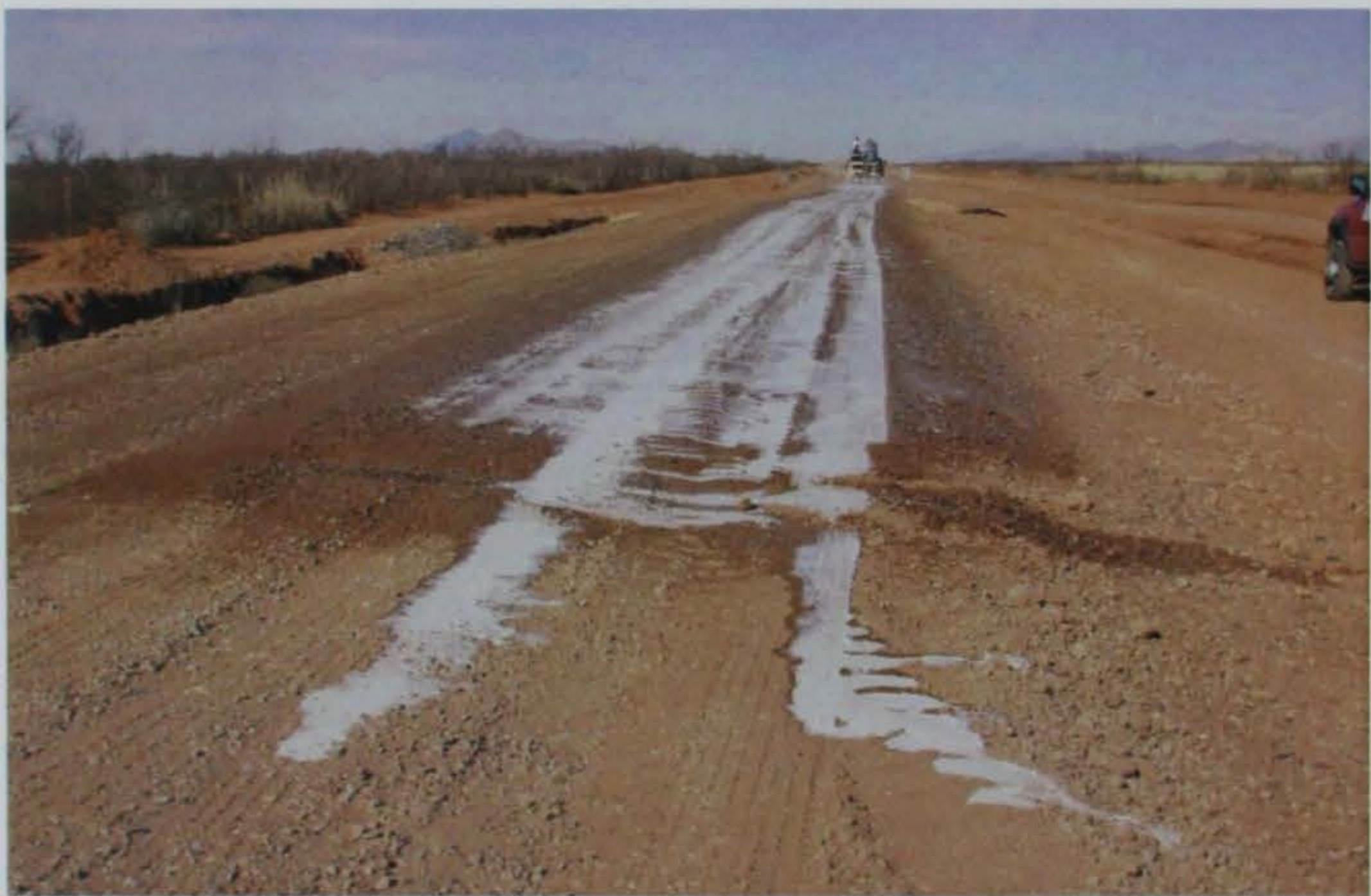
Photo 12. Delayed penetration and product runoff on section 2
