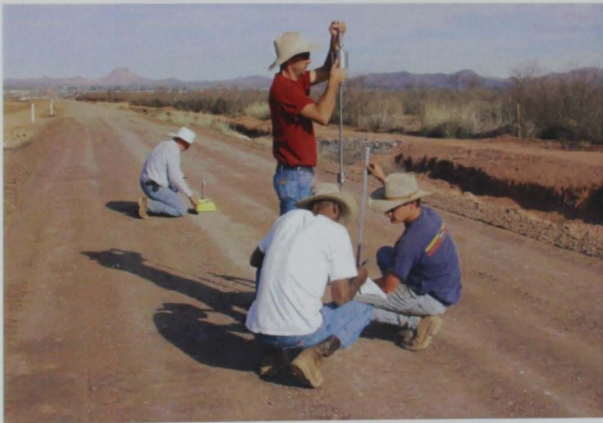
Photo 22. Data collection with DCP and nuclear gauge 1 day after construction
