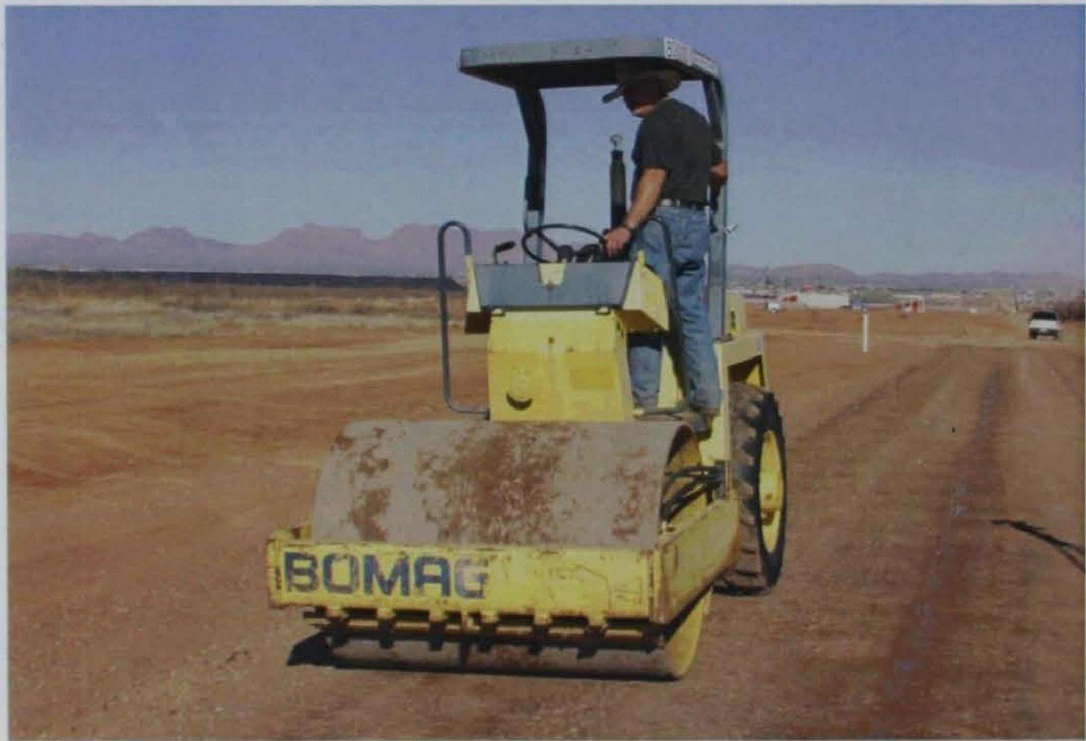
Photo 8. BOMAG 6-ton steel wheeled vibratory compactor
