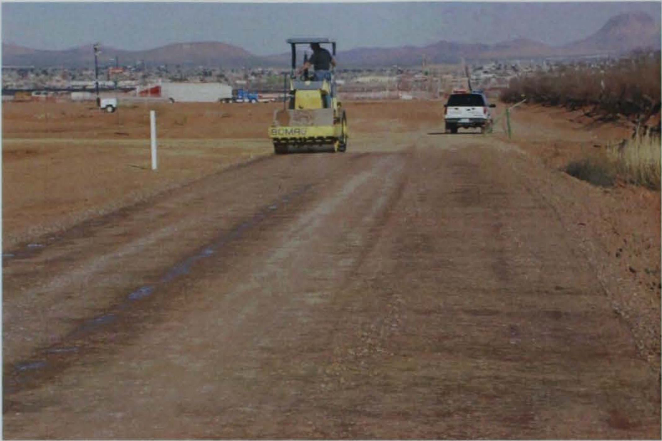
Photo 11. Section 1 after compaction
