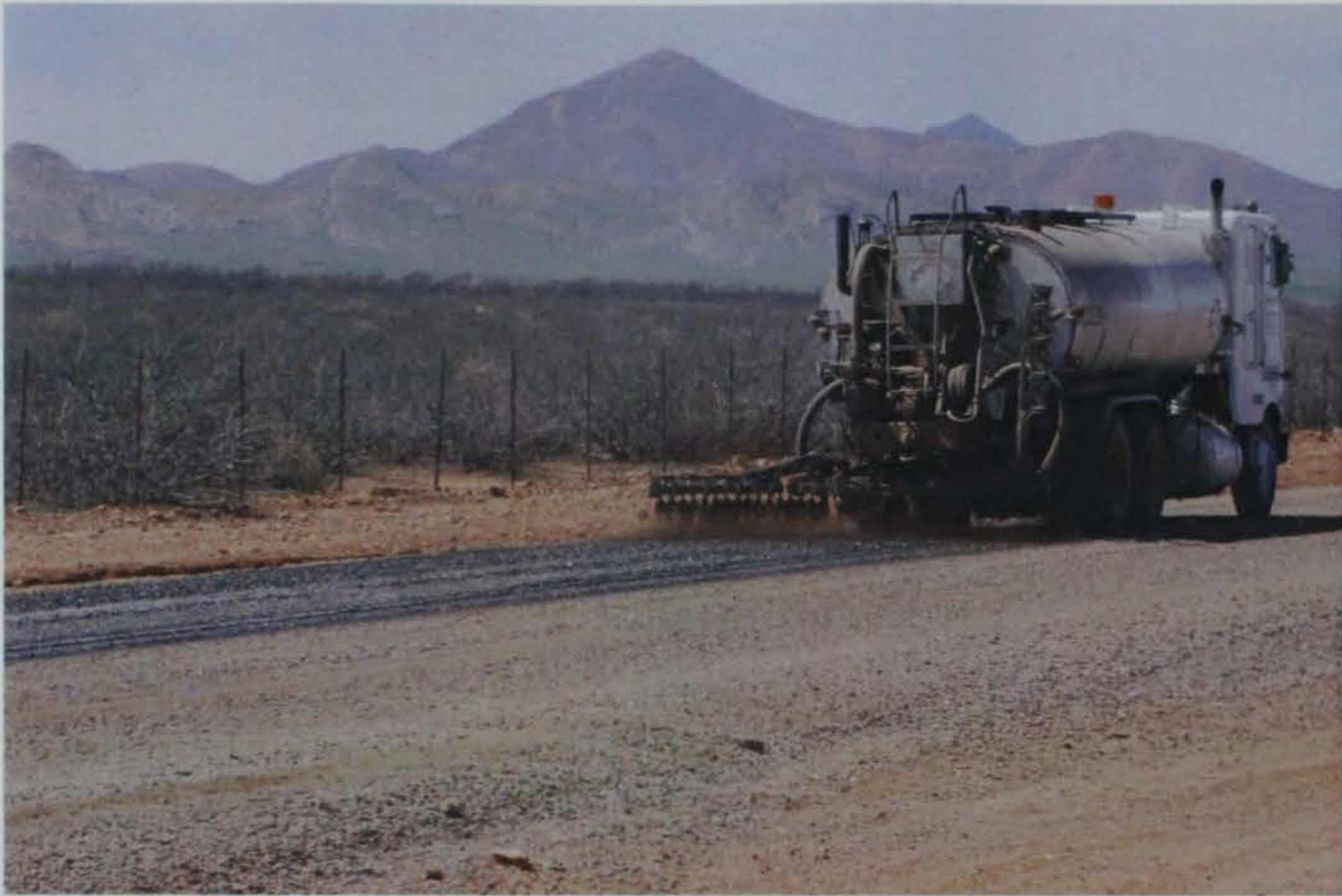
Photo 35. Application of asphalt emulsion by heated tanker with distribution bar
