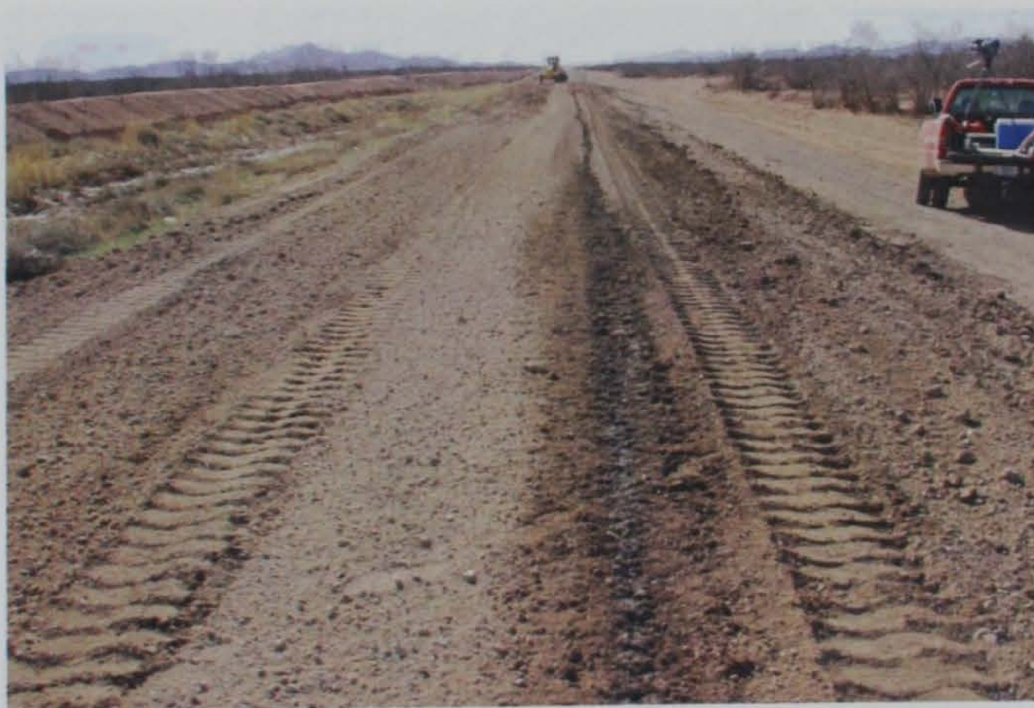
Photo 18. Dry center of test section and uneven product distribution after spreading of windrow on Section 5
