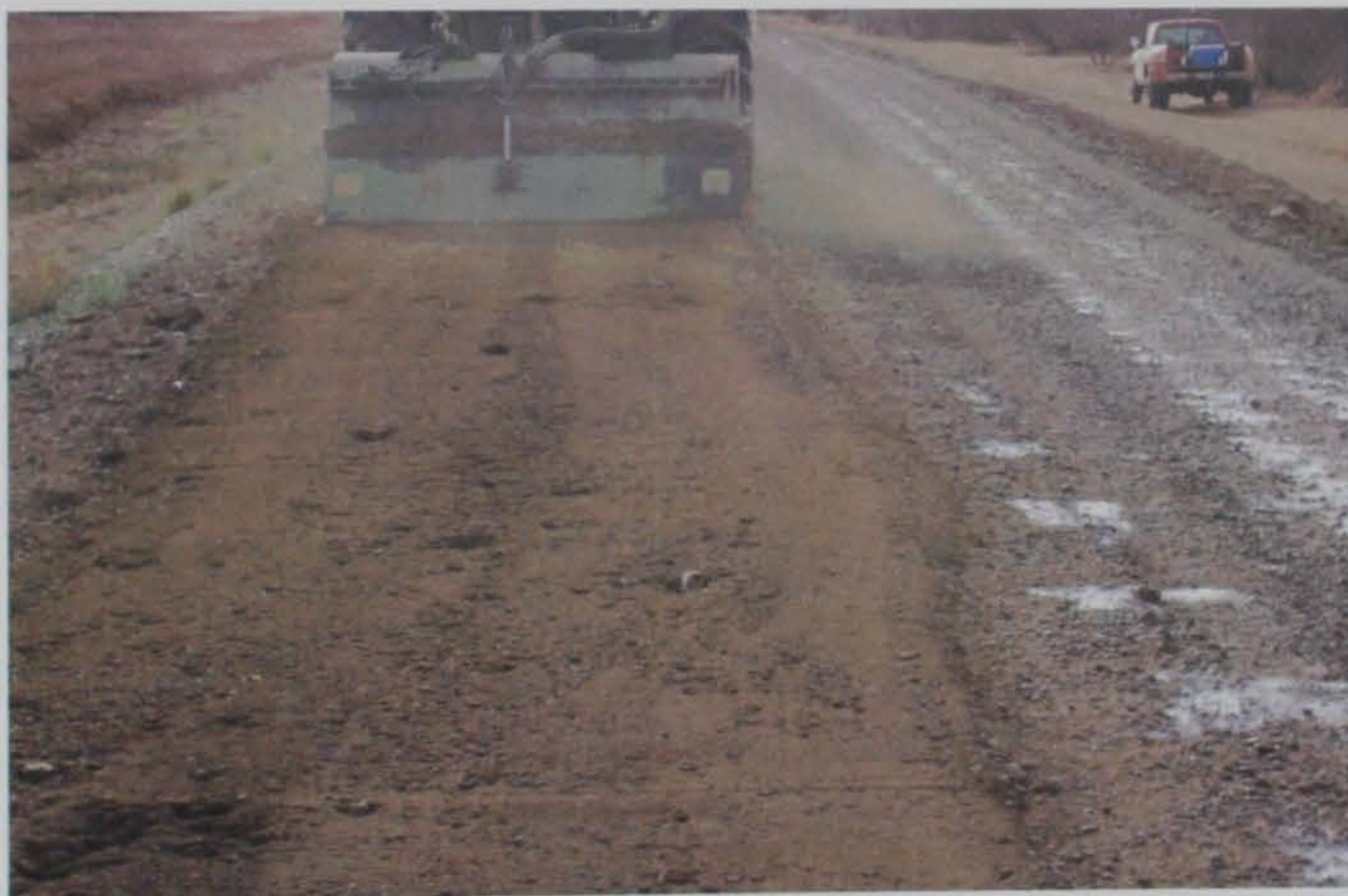
Photo 14. Tilling surface after spraying product to incorporate palliative into soil
