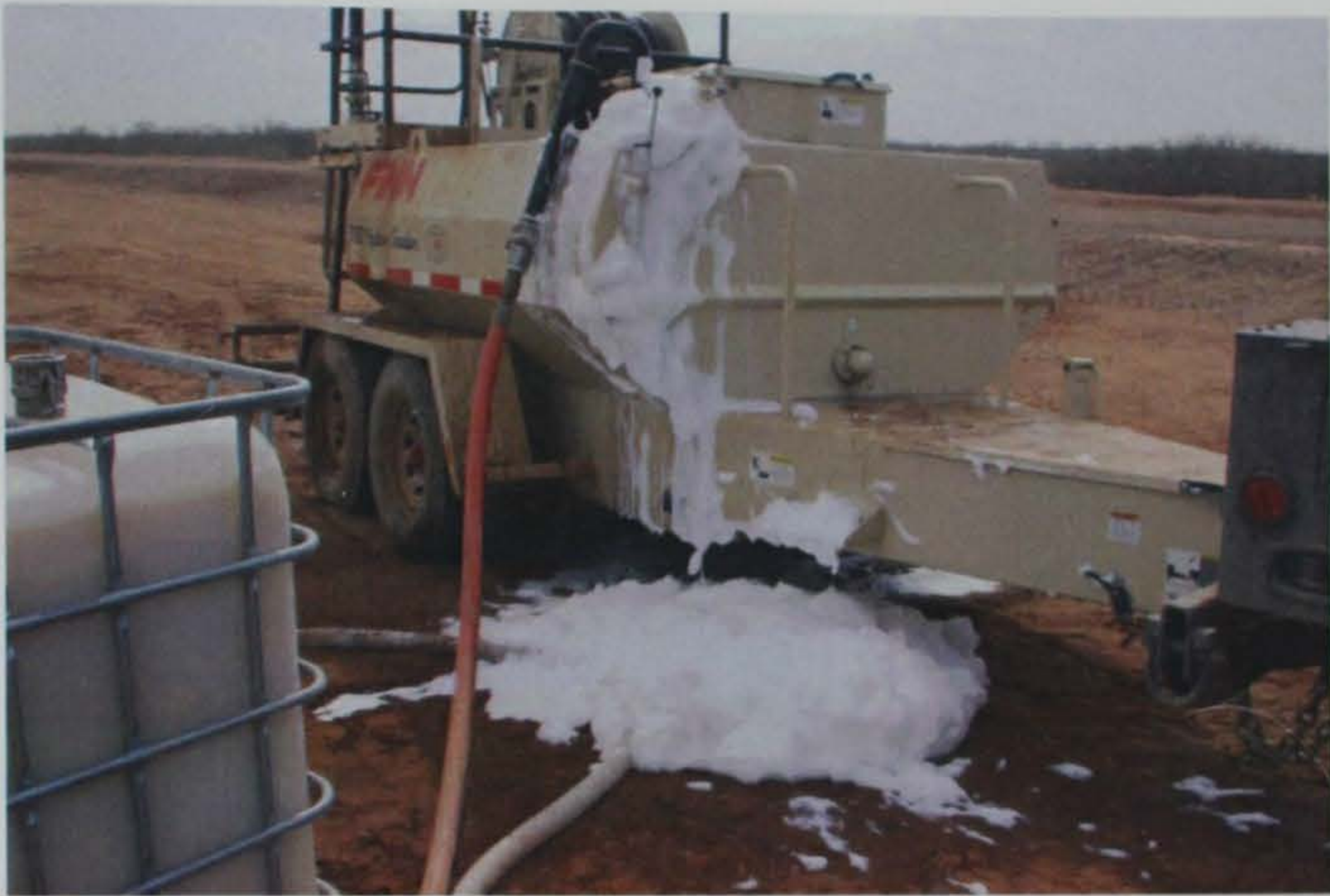
Photo 33. Foam overflowing hydroseeder while filling with Polytac®
