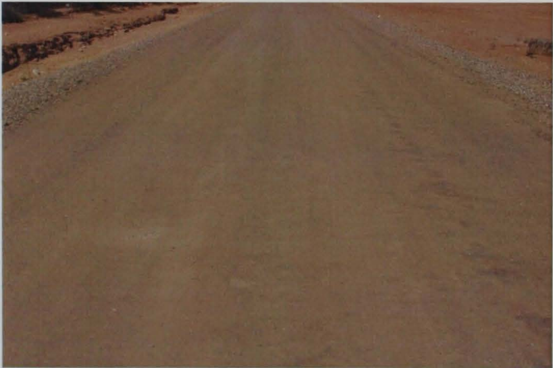
Photo 36. Undisturbed surface of Section 18 after 30 days
