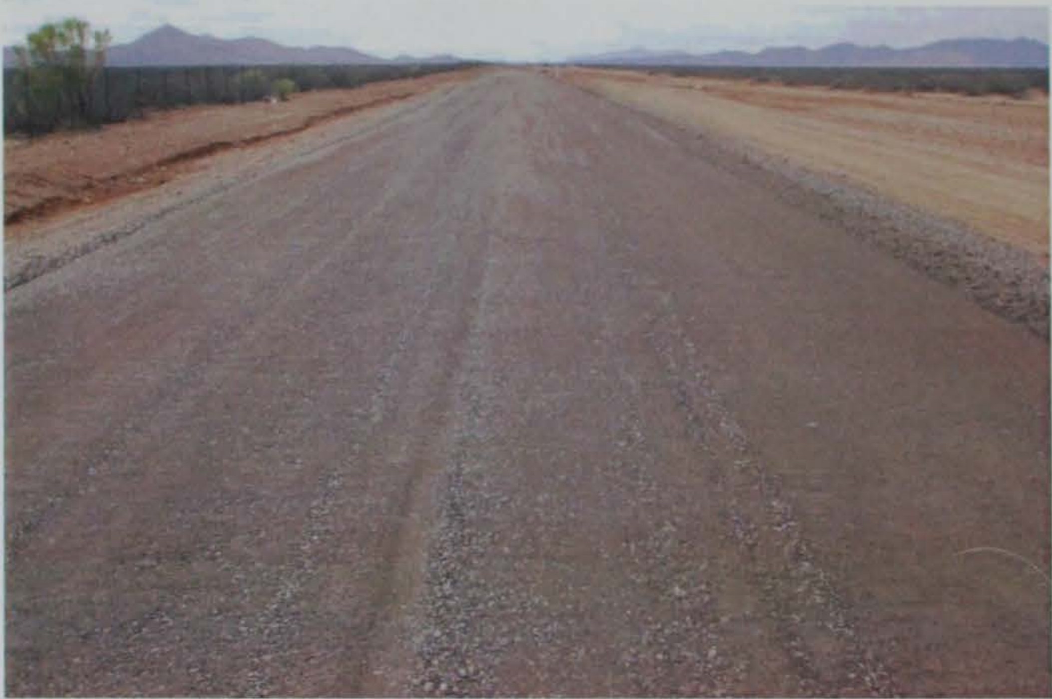
Photo 21. Final road surface after topical application
