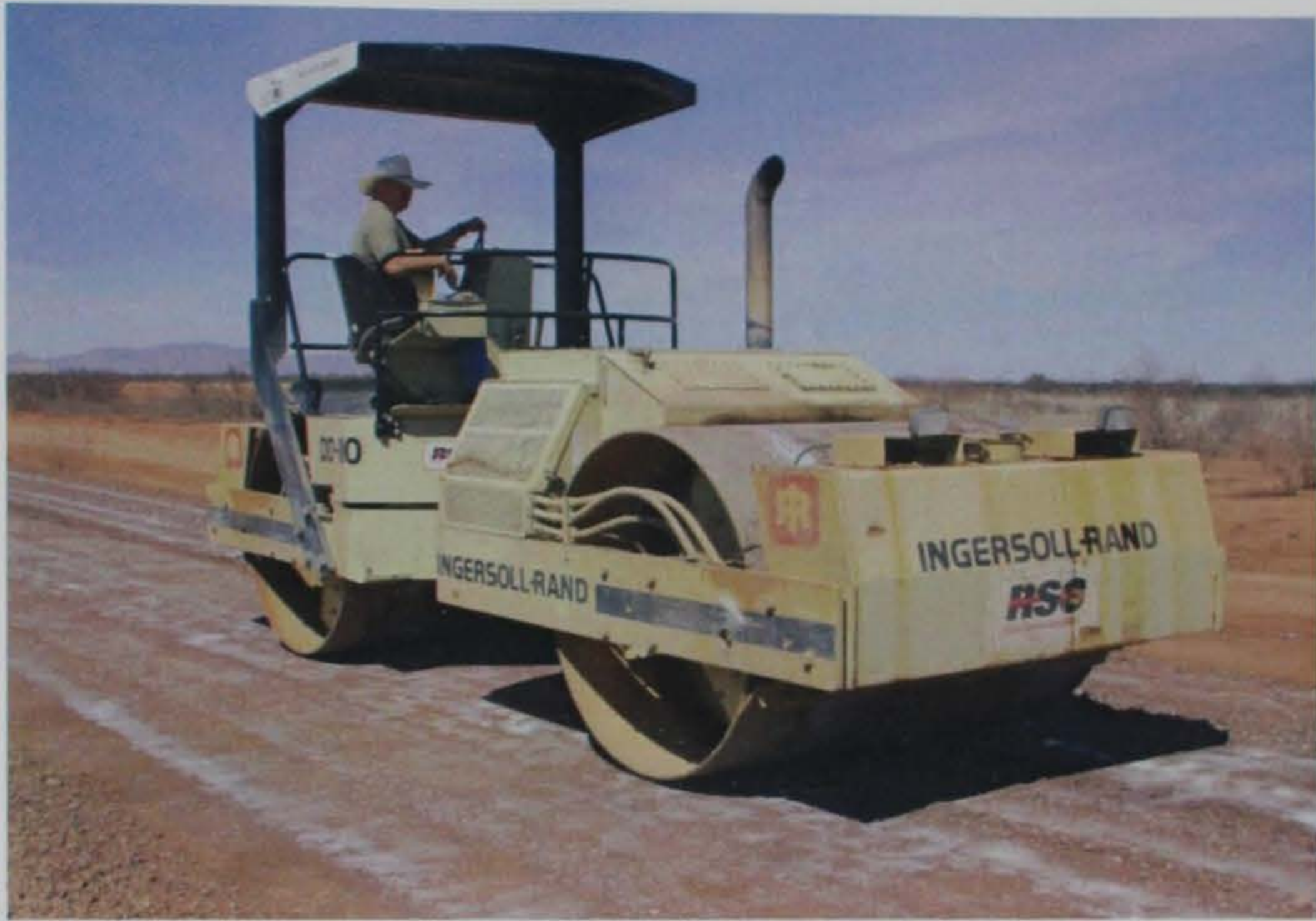
Photo 9. Ingersoll-Rand 12-ton vibratory compactor
