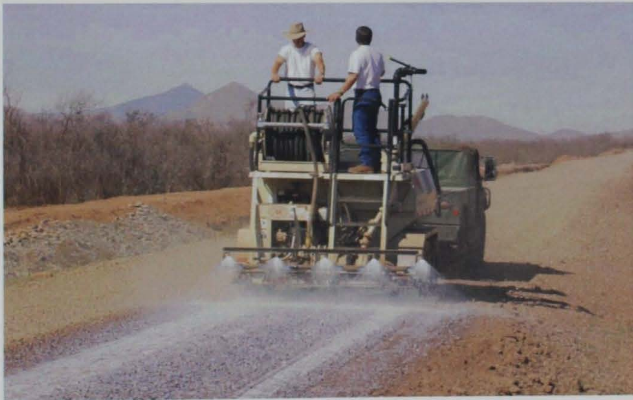
Photo 10. Spraying from distribution bar on hydroseeder
