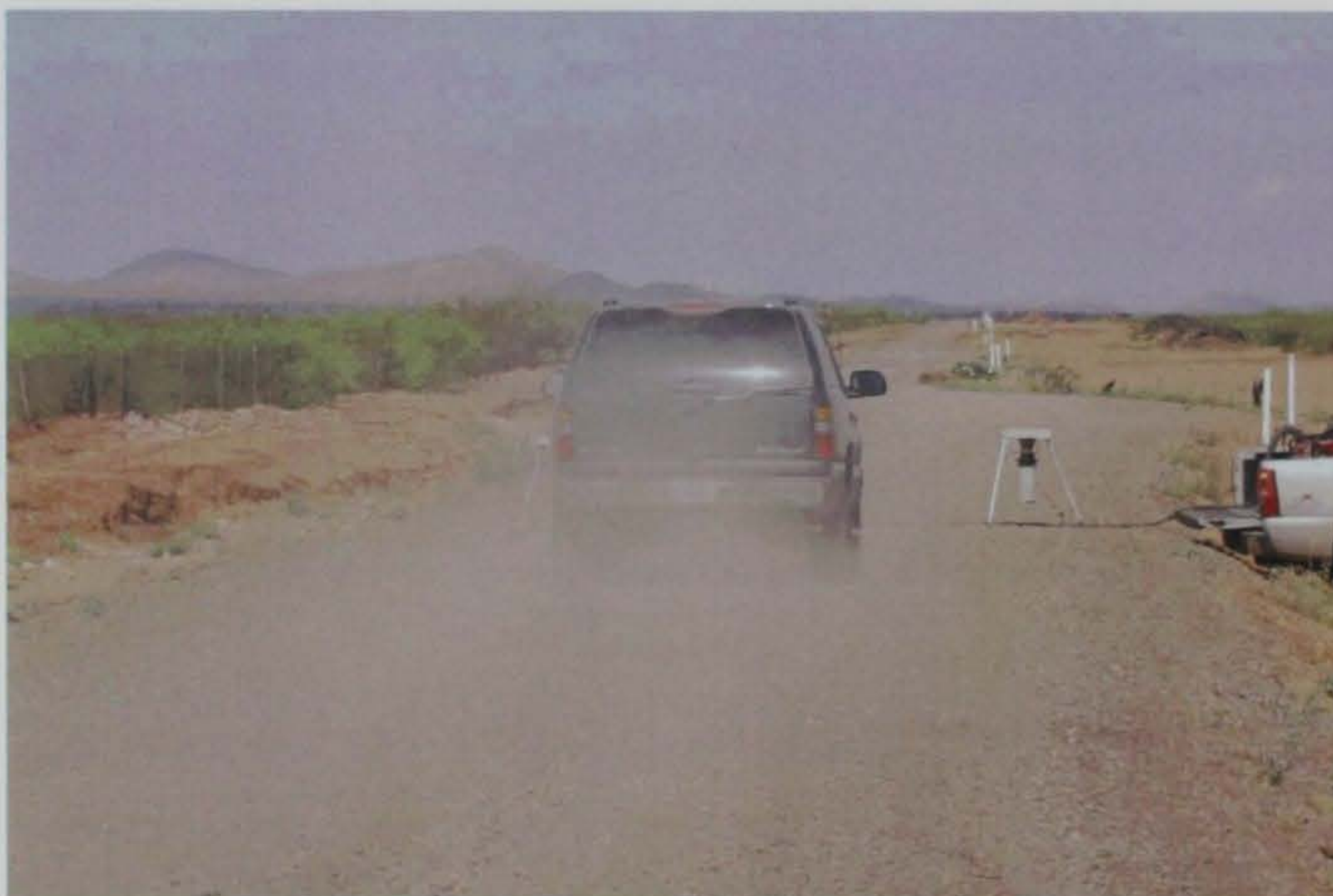
Photo 44. Data collection on test section treated with Dustex®
