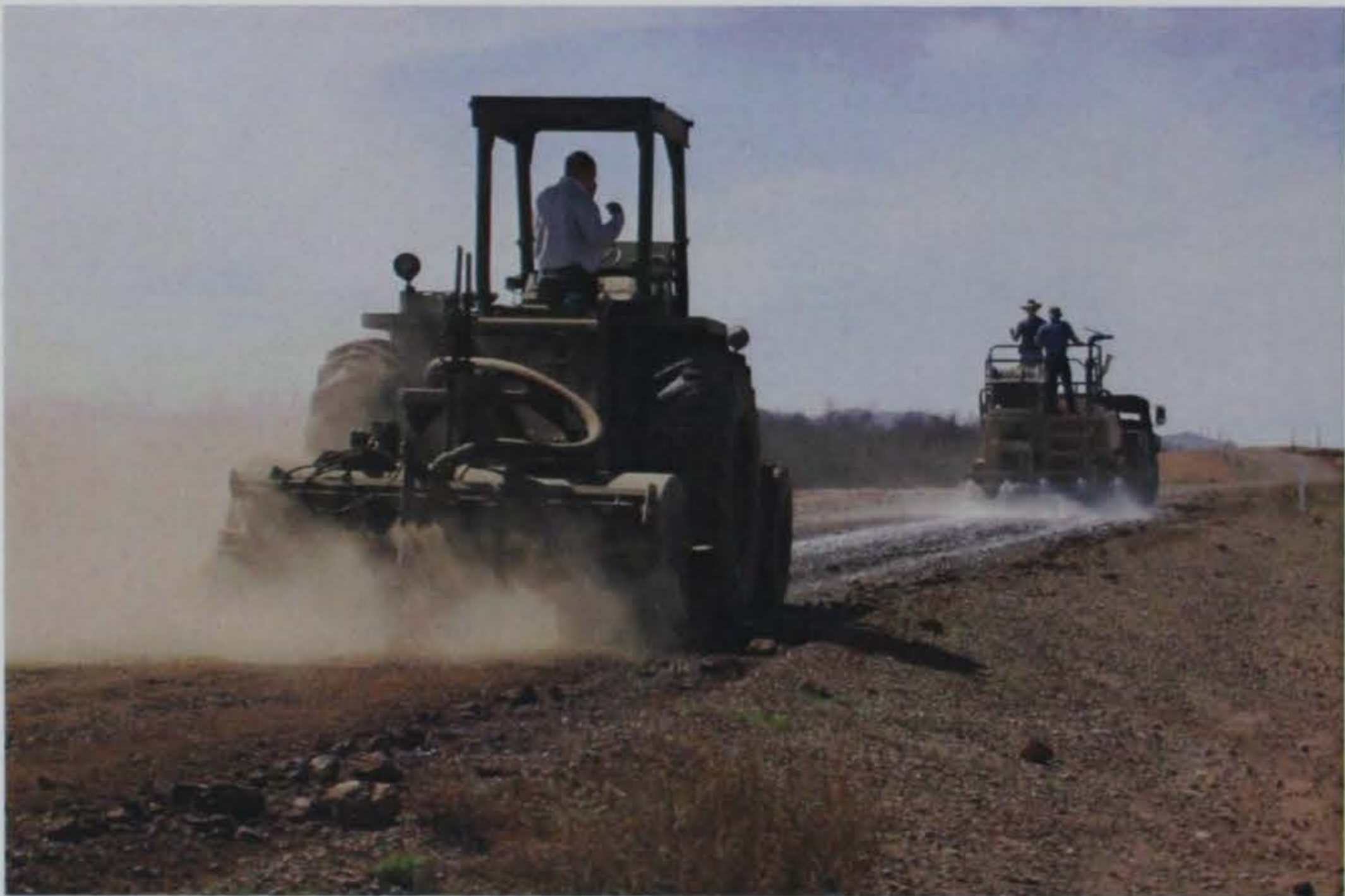
Photo 20. Immediate tilling of product after spraying onto surface
