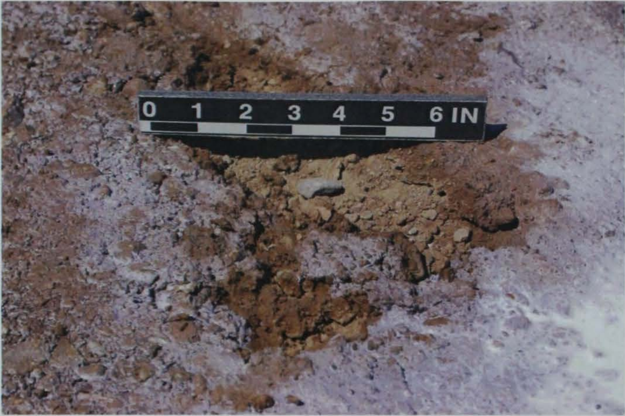
Photo 15. Removal of surface crust from product sticking to roller on compactor
