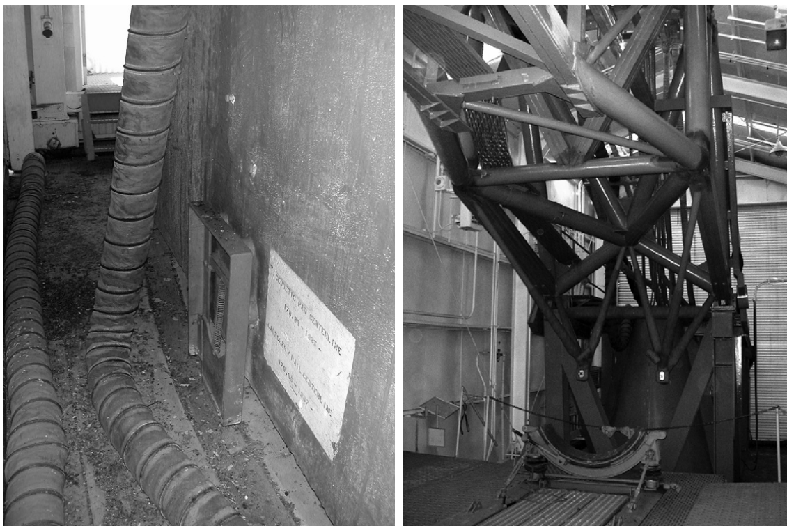
Figure 9. Launcher ballast (left) and lug assemblies (right), VAFB Facility #580, 2008 (ERDC-CERL).
