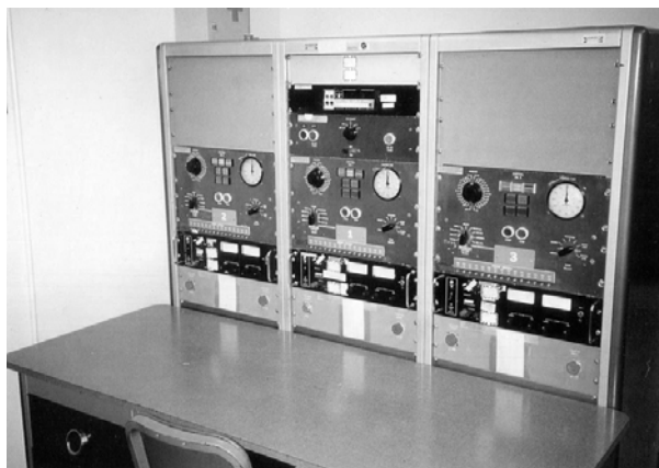
Figure 6. Battery-handling console in battery shop, VAFB Facility #582, circa 1990 (Collection of Jim Price).
