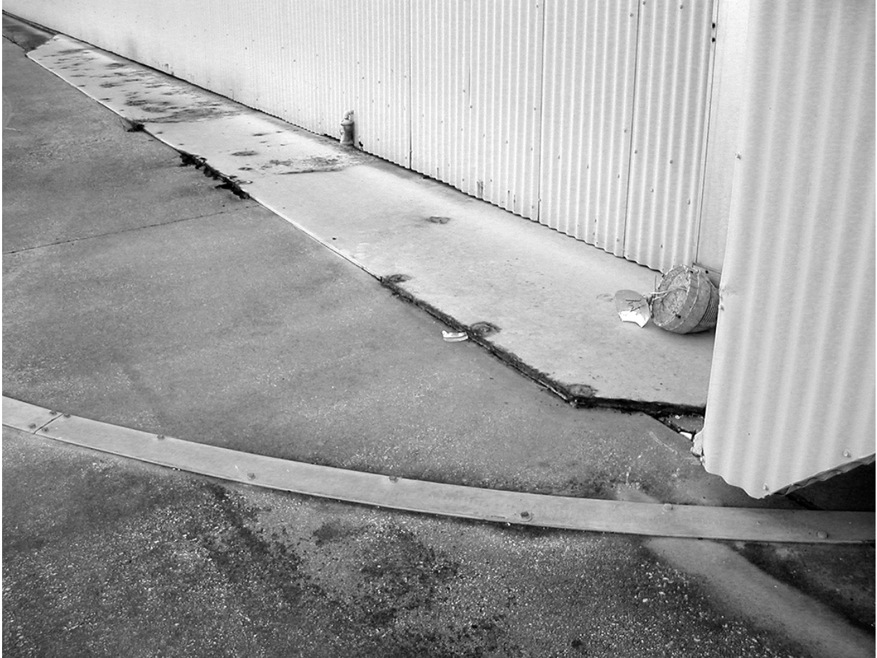
Figure 11. Portion of the azimuth ring and blast plates, 2008 (ERDC-CERL).
