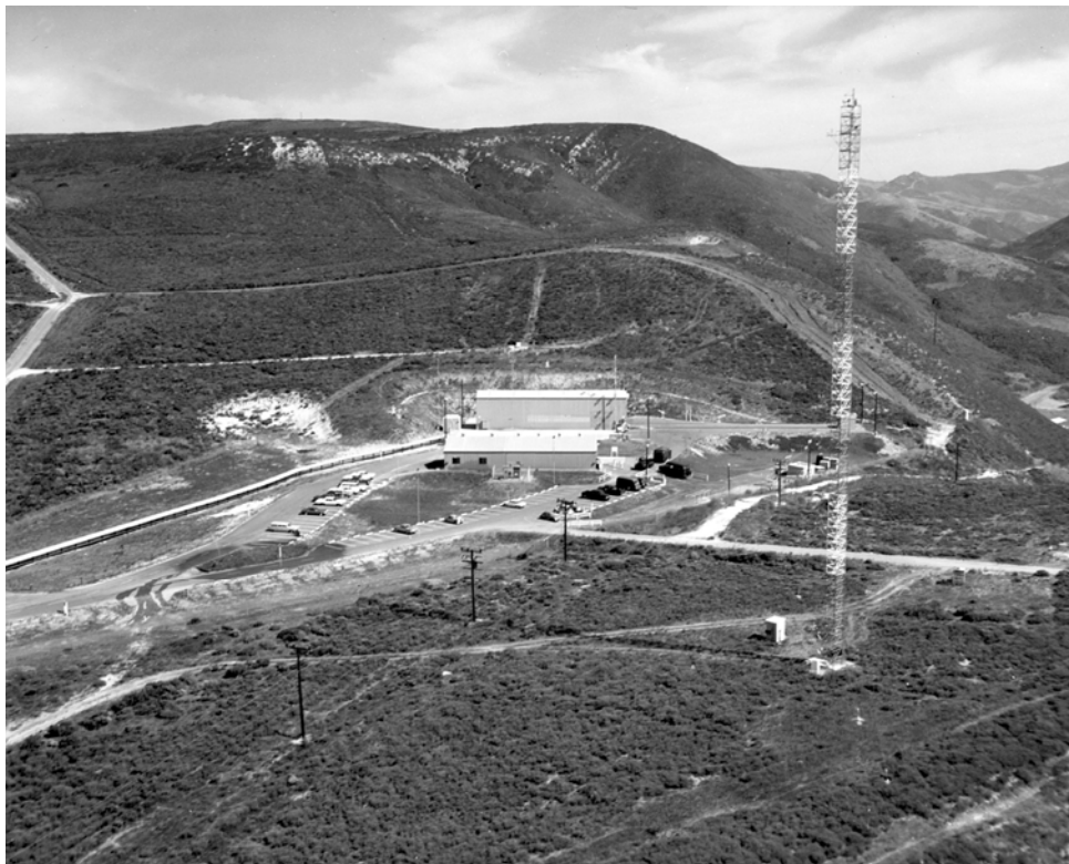
Figure 26. Aerial view of SLC-5, 1967 (Official USAF Photograph).
