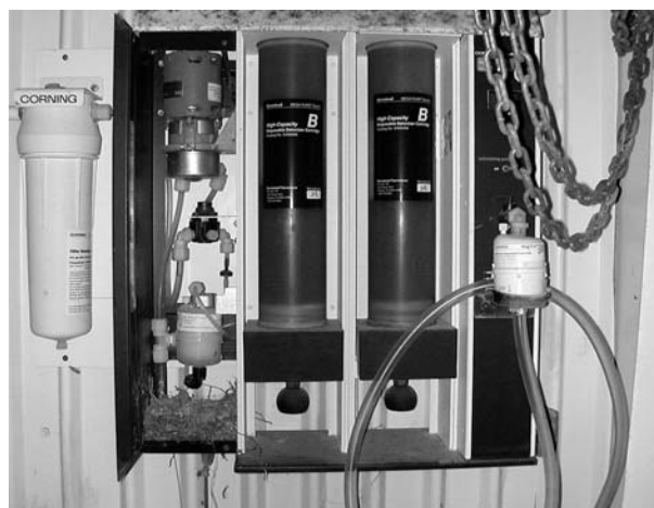
Figure 2. Fueling room deionization unit, VAFB Facility #582, 2008 (ERDC-CERL).
