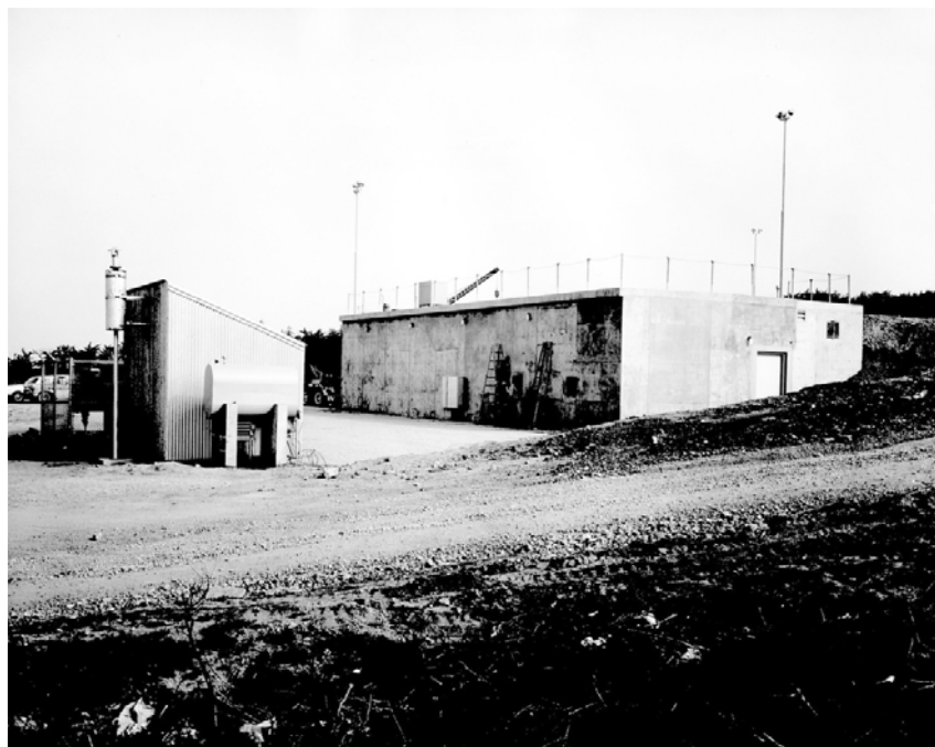
Figure 18. Probe blockhouse nearly completed, 5 February 1962 (U.S. Navy Seabee Museum, Port Hueneme, CA).
