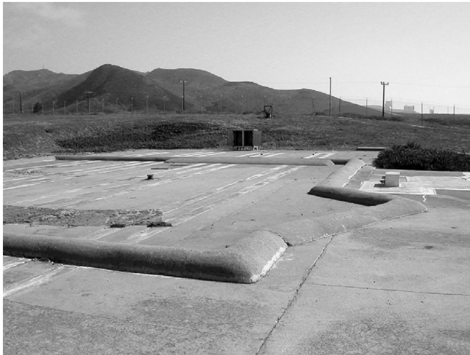
Figure 6. Concrete dike around Probe launch pad, 2008 (ERDC-CERL).
