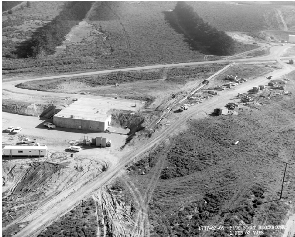
Figure 17. Blockhouse construction, 1 February 1962 (Official USAF photograph).
