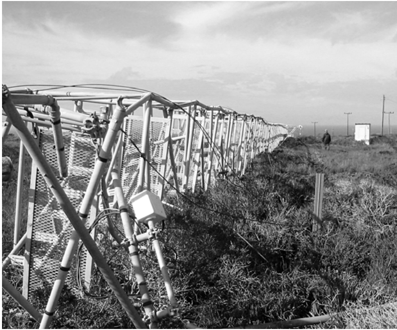
Figure 25. The meteorological tower was demolished 3 January 2003 (VAFB Cultural Resources Office).
