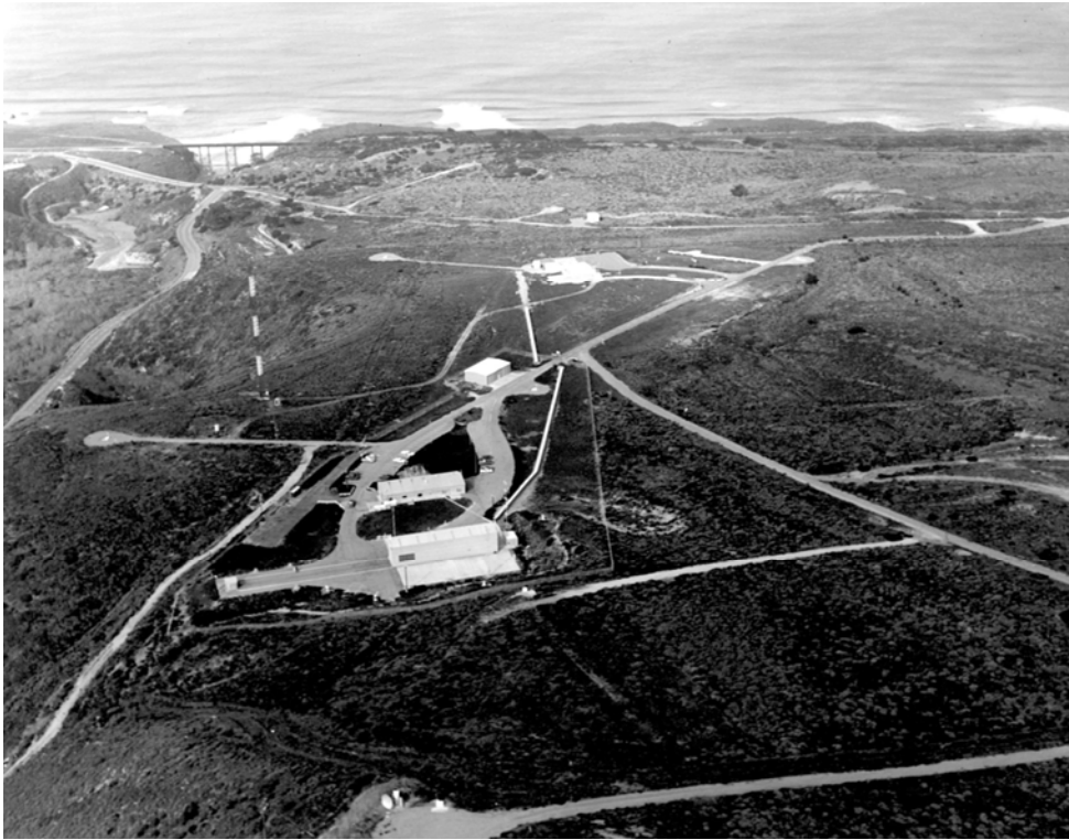
Figure 27. Aerial view of SLC-5, 1979 (NASA HQ History Office, Washington, D.C.).
