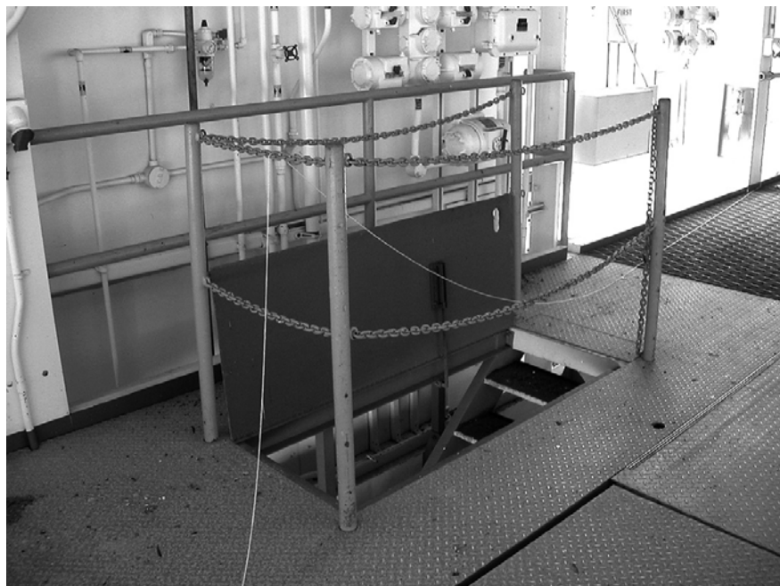
Figure 2. Work platform hatch in open position, VAFB Facility #580, 2008 (ERDC-CERL).
