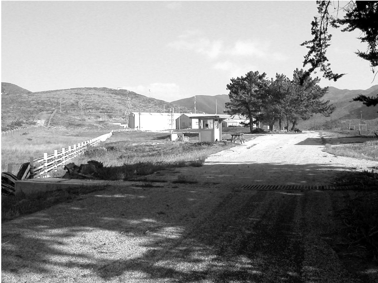
Figure 47. Access control point to uphill Scout facilities in 2008 (ERDC-CERL).
