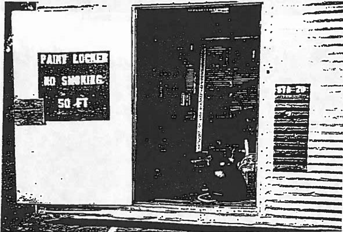
Paint Storage Area at U.S. Coast Guard Station I
