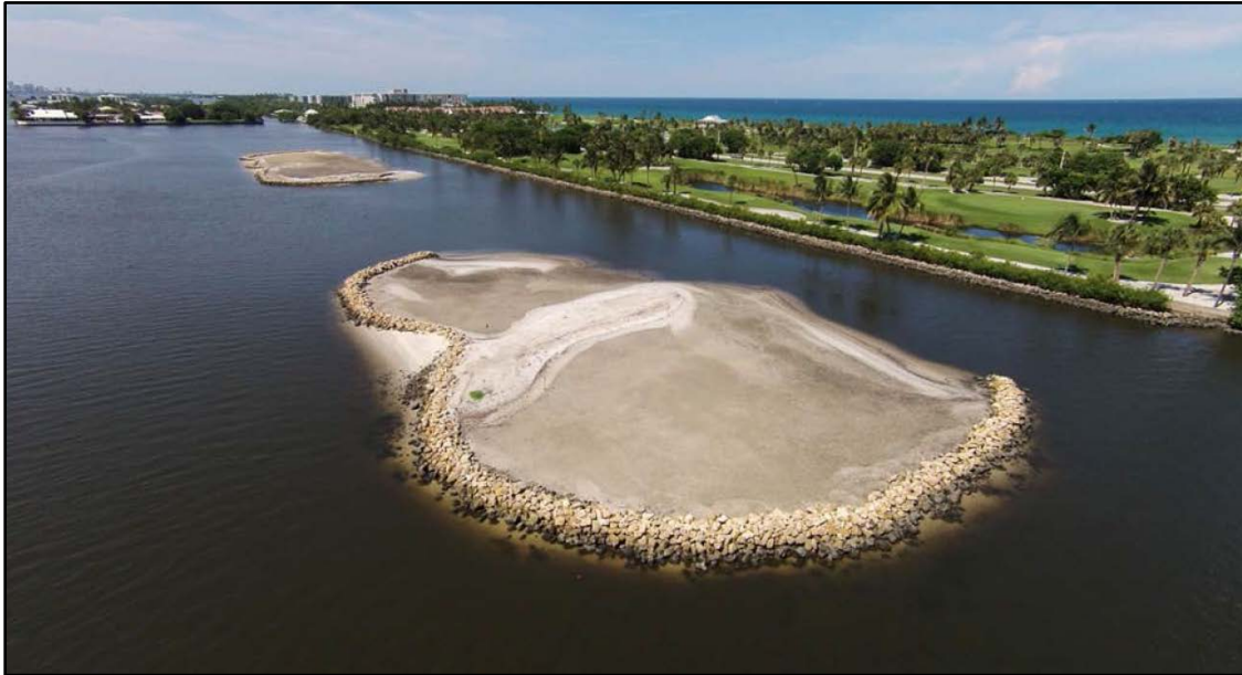
Figure 6. Image of a similar project site prior to planting, showing an example of the rip-rap shoreline used for island stabilization and protection (image supplied by USACE)
