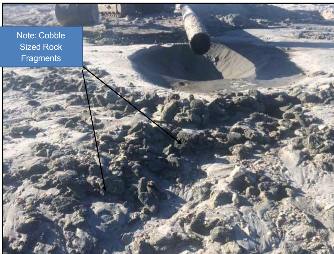
Photograph No. 5 – Dredge Material at Mouth of Dredge
