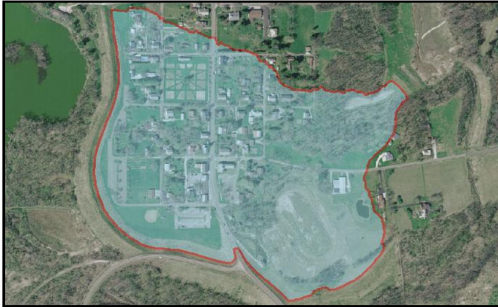
Figure 1-3 Aerial photograph showing portion of Zoar Village below El. 916 feet (highlighted in blue)
