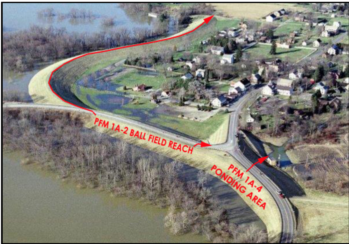
Figure 3-8 Oblique aerial from January 2005 Event showing locations on Zoar Levee associated with PFM 1A-2 & PFM 1A-4.
