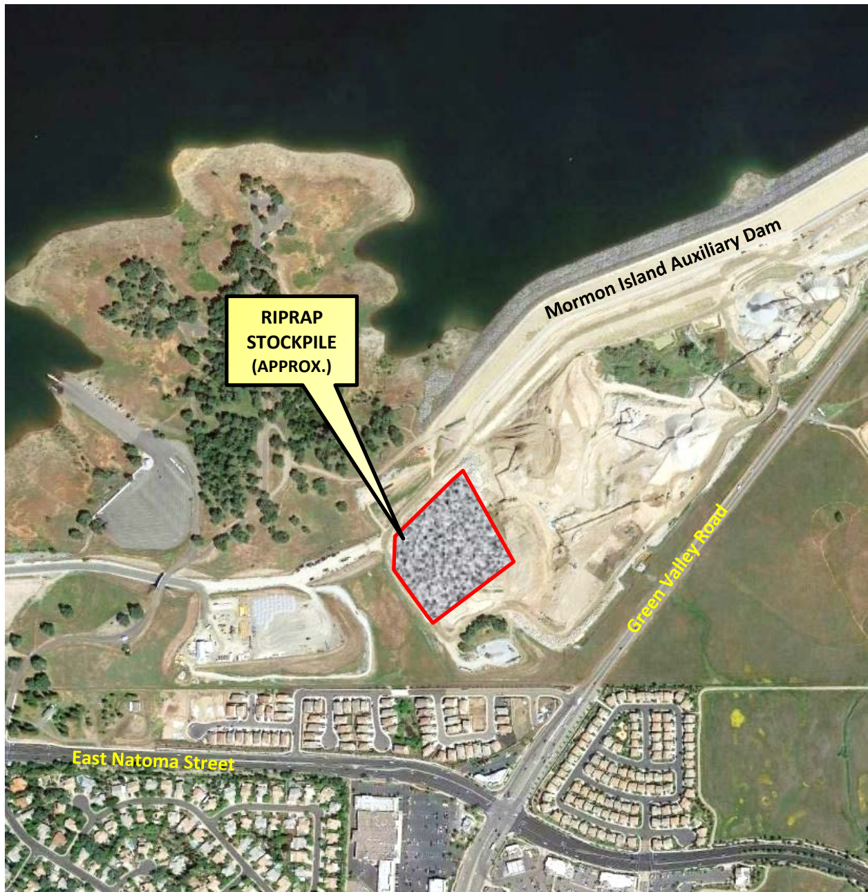
Figure 2-15. Approximate location of existing riprap stockpile within the MIAD East Area.
