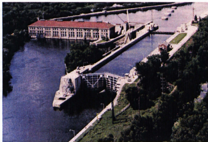
Figure D34. Lockport Lock and Dam, Illinois Waterway
