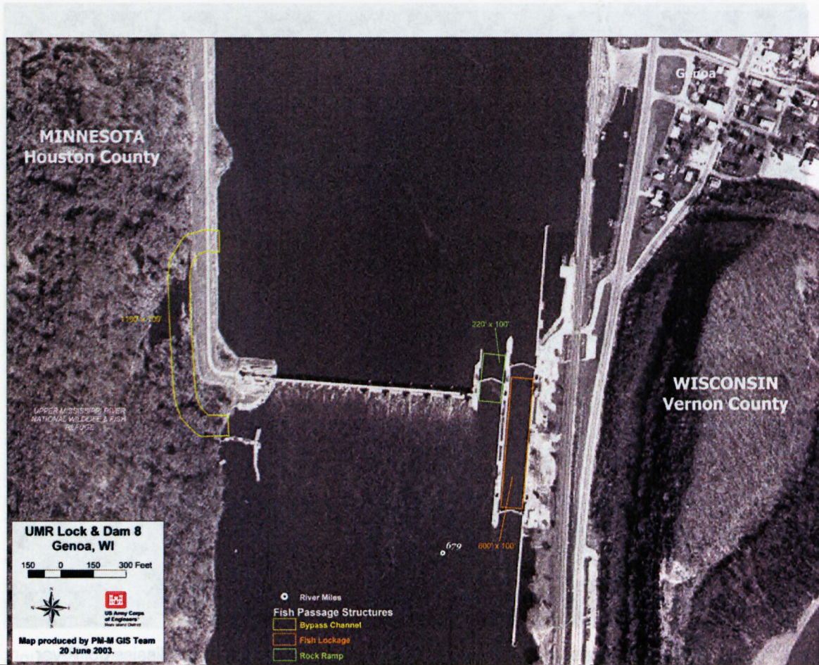
Figure D9. Potential fish passage improvements at Lock and Dam 8, Upper Mississippi River
