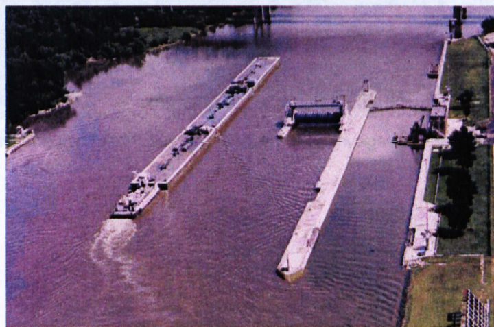
Figure D29. Peoria Lock and Dam, Illinois Waterway
