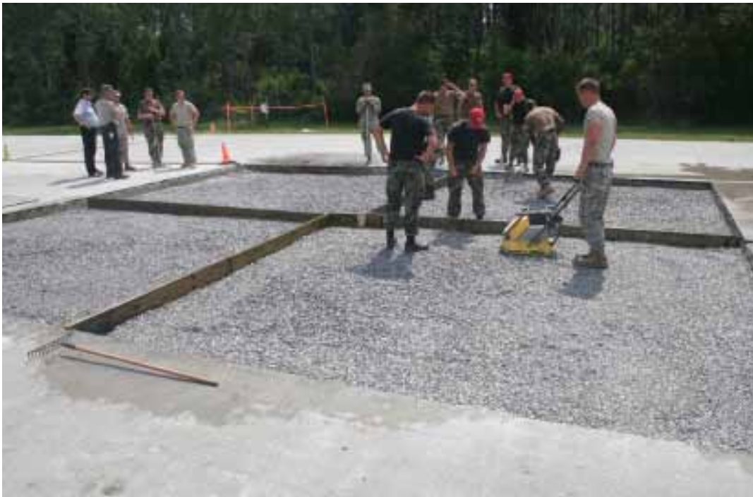
Figure 66. Crater 2 formed and layer of aggregate added.
