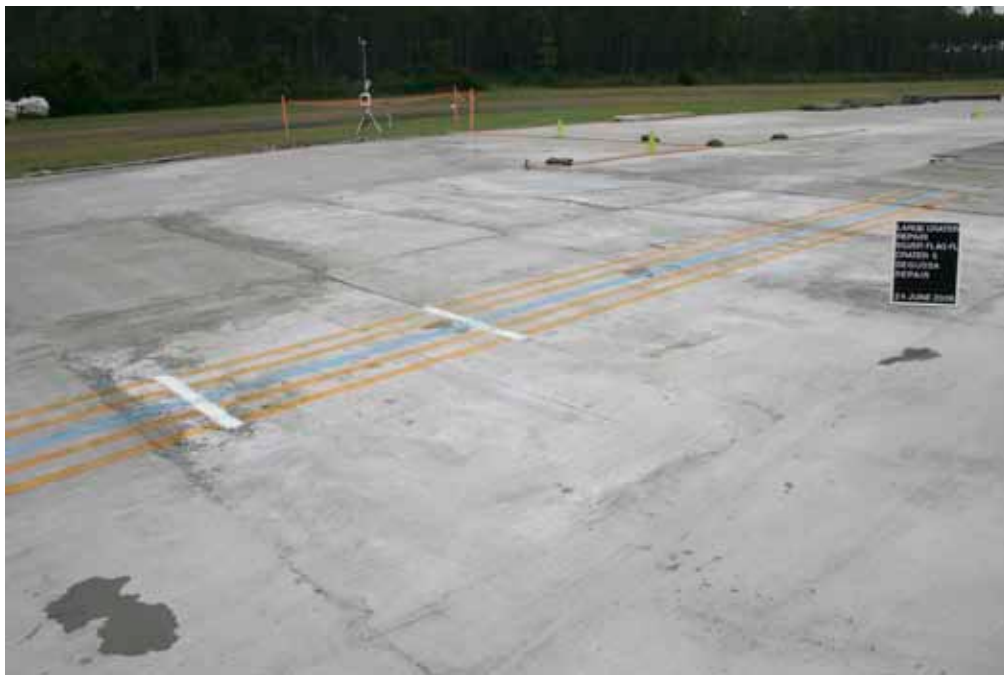
Figure 62. Final crater repair in Crater 5.
