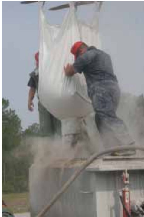
Figure 82. Adding Ultimax concrete to the mixer for Crater 4.
