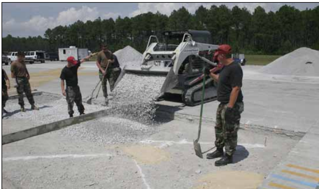
Figure 12. Installed instrumentation in test crater.
