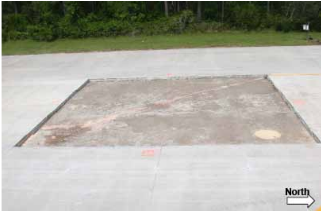
Figure 19. Crater 1 prior to cap placement.
