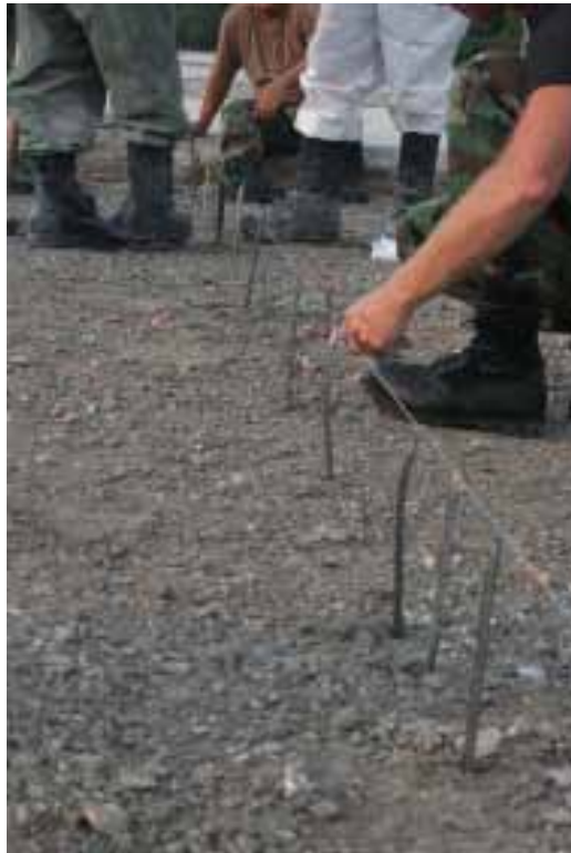
Figure 79. Bent aluminum stakes resulted from the use of hand tools during the installation of stay-in place forms in Crater 4.
