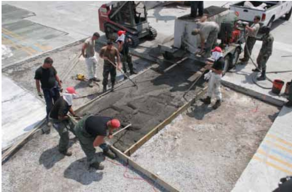
Figure 60. Repairing the traffic lane in the southeastern quadrant for Crater 5.
