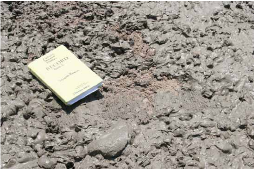
Figure 33. Adequate coating of grout around stone in Crater 1.
