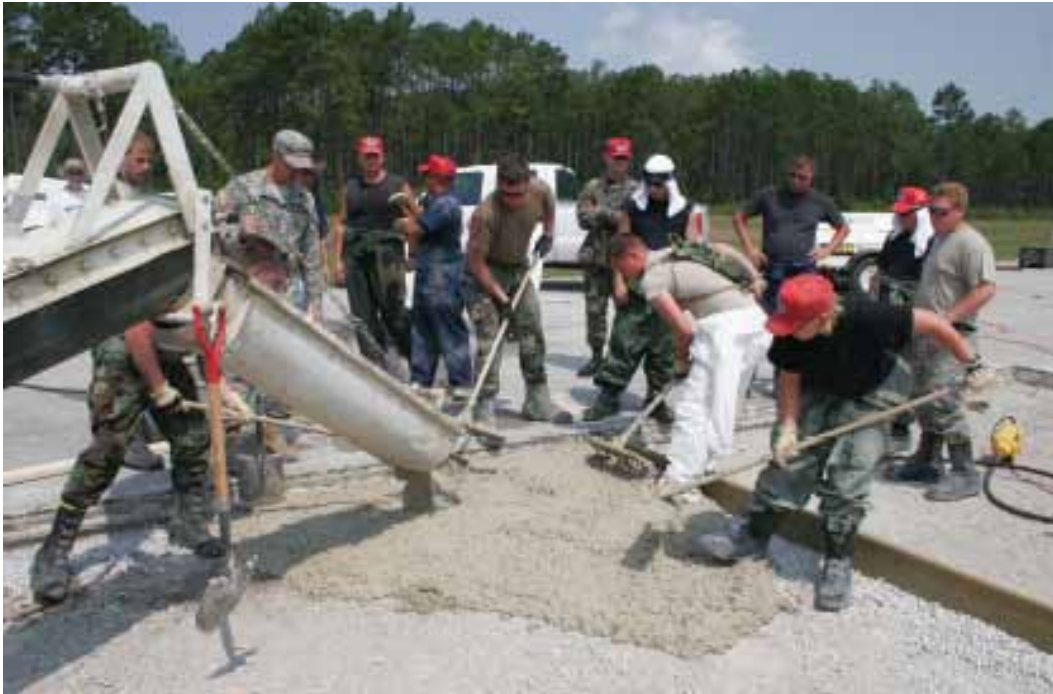
Figure 44. Pouring Rapid Set DOT concrete into the southwestern quadrant of Crater 6.
