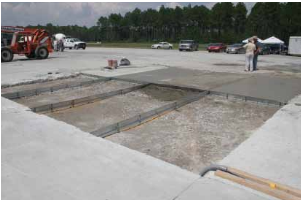
Figure 85. Completed Sections 1 through 4 of Crater 4.
