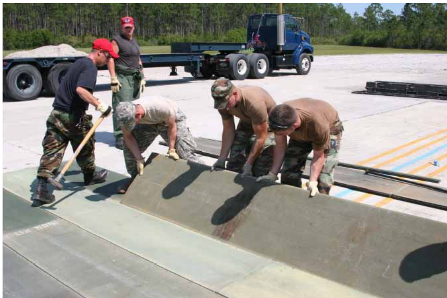
Figure 8. Placing AM2 matting in traffic area to protect existing pavement.
