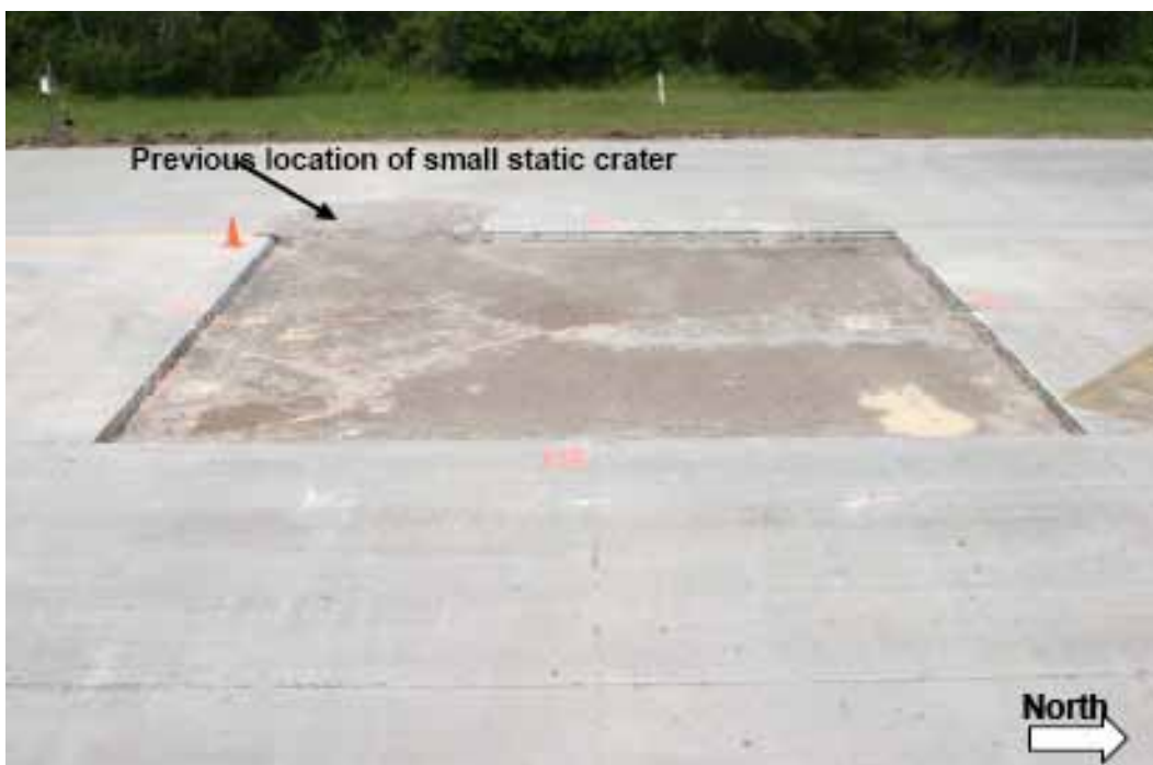
Figure 20. Crater 2 prior to cap placement.
