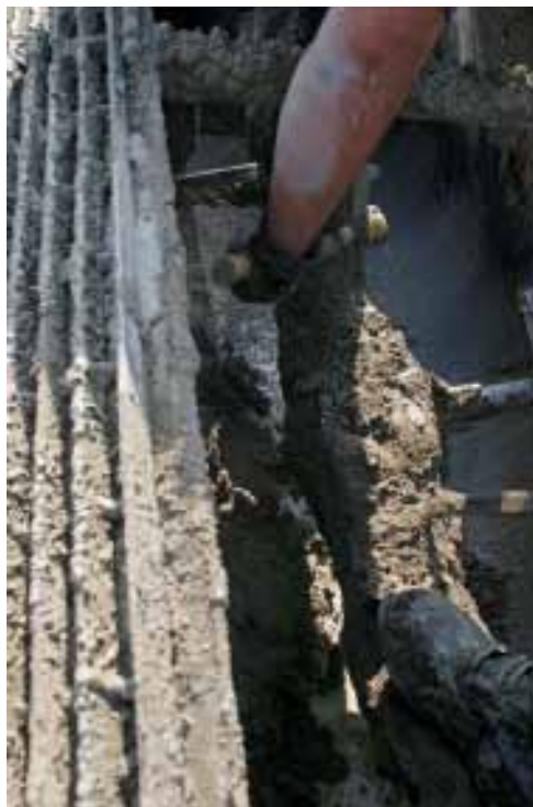
Figure 86. Breaking up large clumps of unmixed Ultimix concrete material building up on the center shaft with a ball-peen hammer.
