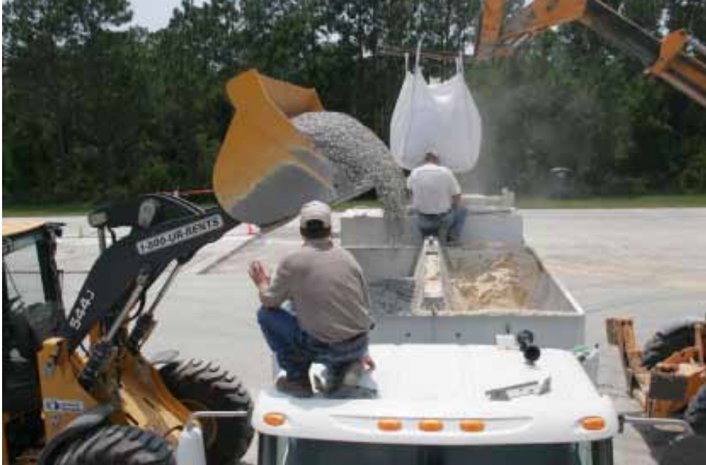
Figure 48. Refilling proportional mixer with stone and cement for Crater 6.
