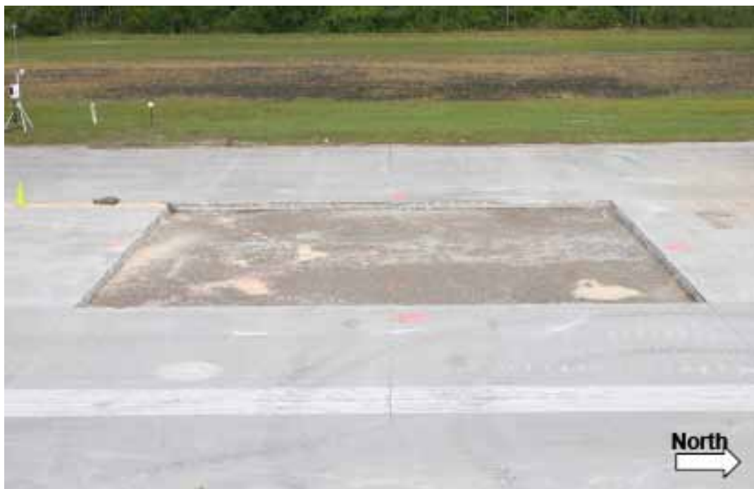
Figure 24. Crater 6 prior to cap placement.
