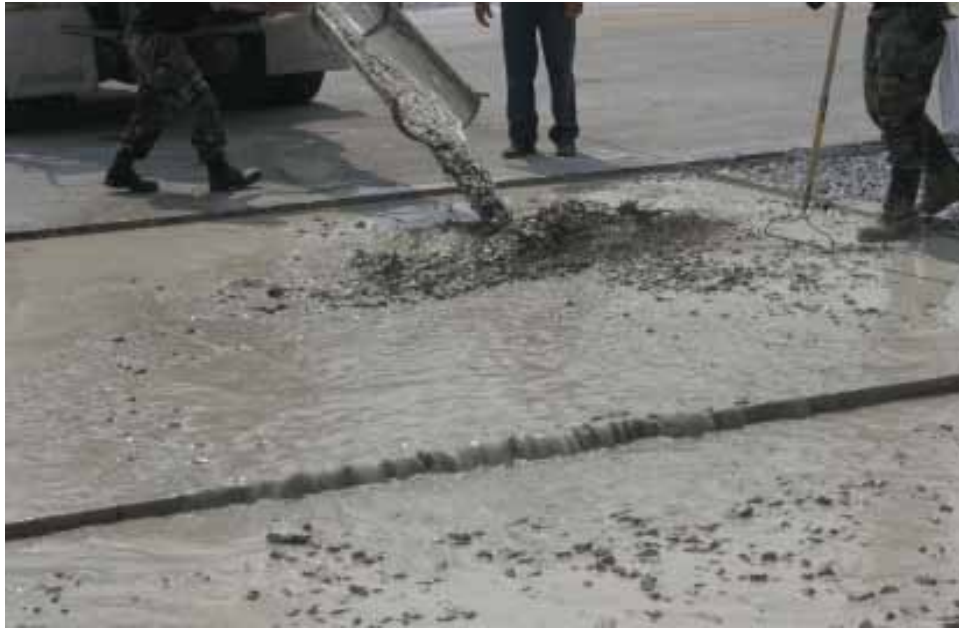
Figure 93. Aquacrete overflowing out of northeast quadrant of Crater 3.
