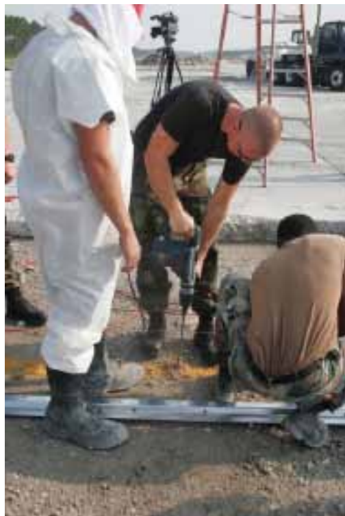
Figure 80. Drill used to make pilot hole to install form stake in Crater 4.
