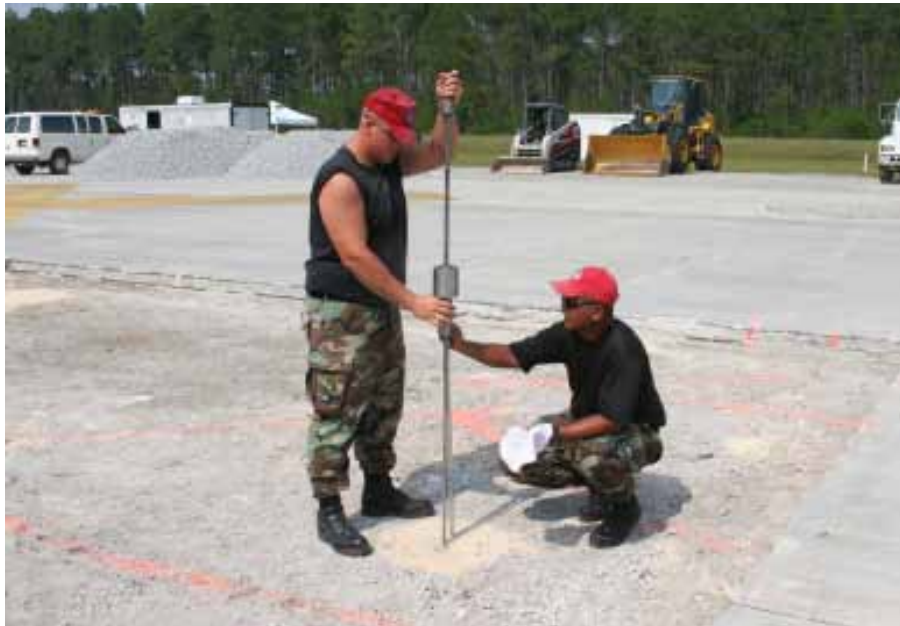
Figure 17. Soil strength testing with the DCP.
