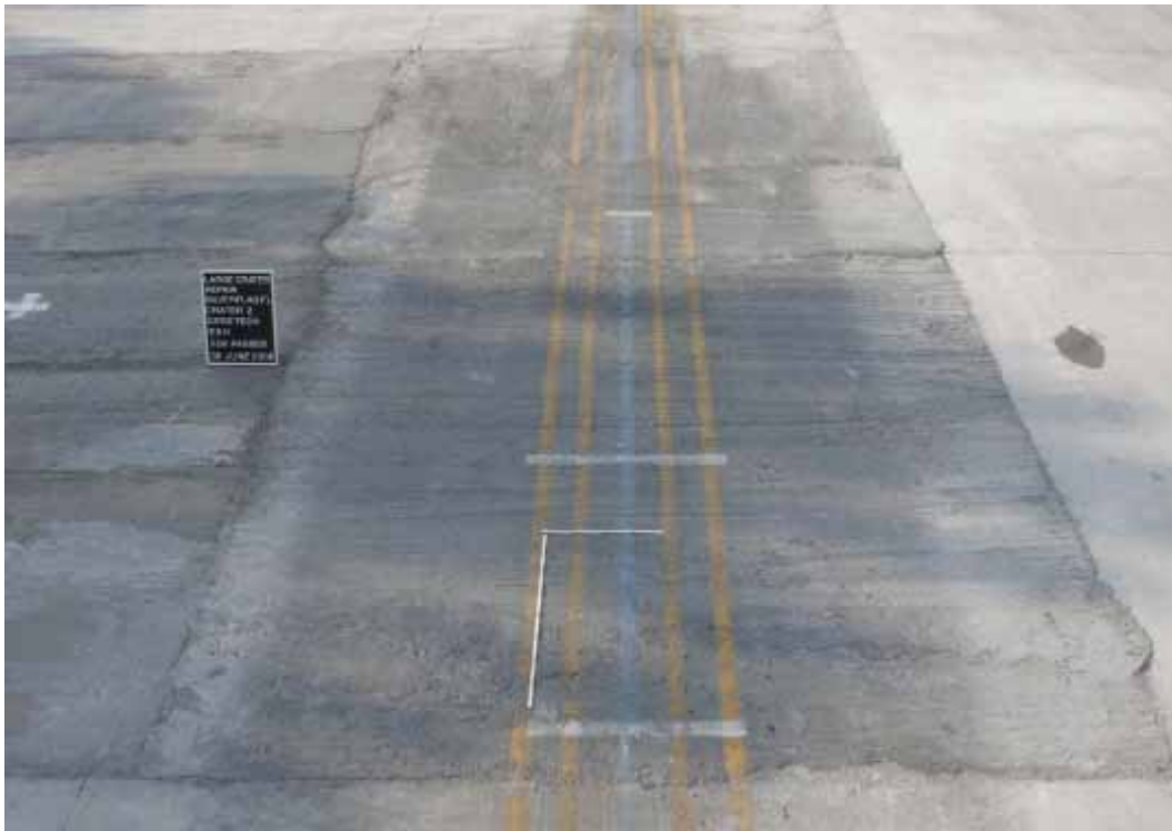
Figure 142. Crater 2 after 528 completed load cart passes.
