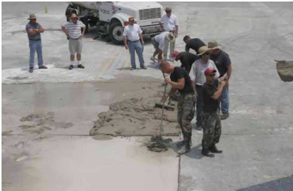
Figure 96. Gelled Aquacrete material could not be placed in Crater 3.
