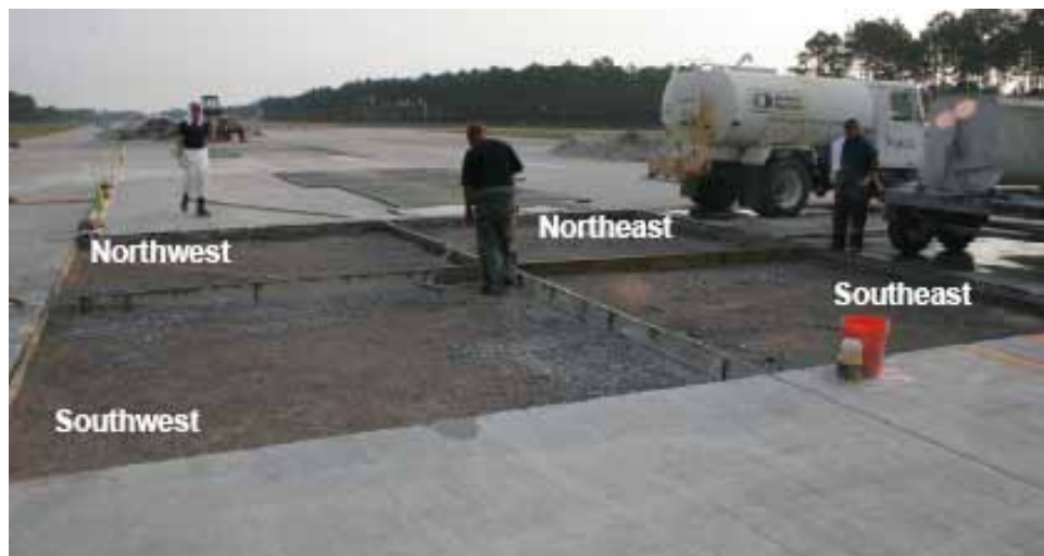
Figure 53. Formwork configuration in Crater 5.
