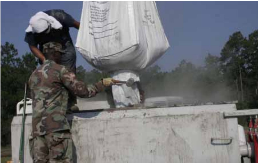
Figure 57. Striking the bottom of the supersack with a rubber mallet to improve material flow for Crater 5.
