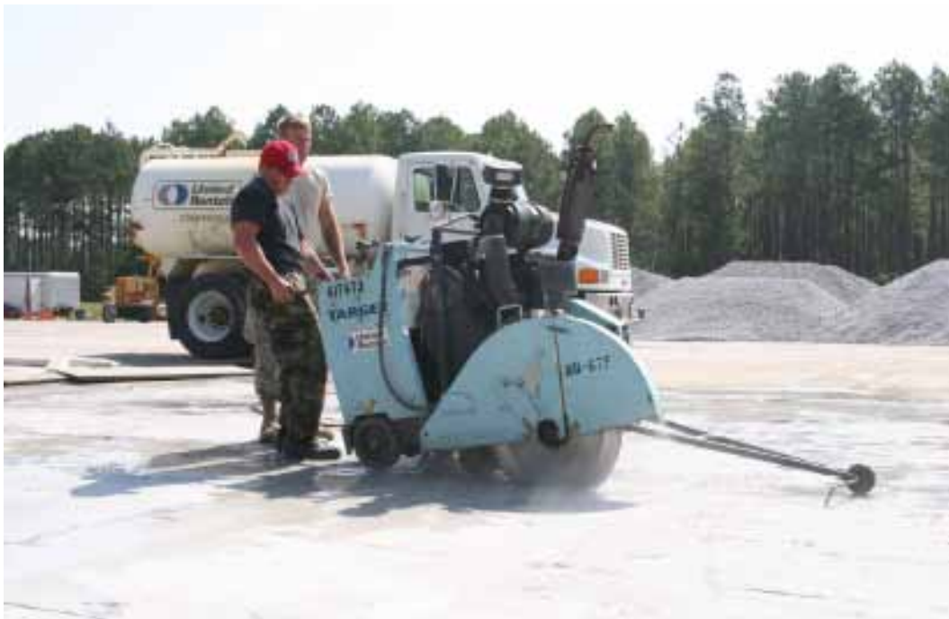
Figure 37. Saw cutting joints in Crater 1 stone and grout repair.
