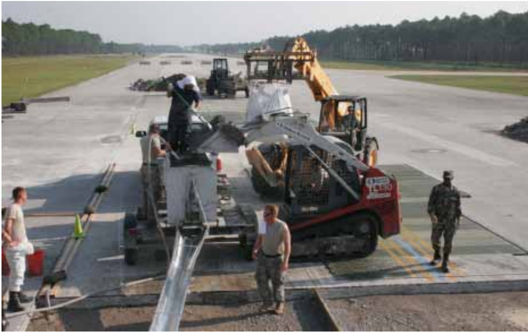
Figure 56. Mixing first batch for Crater 5 repair.
