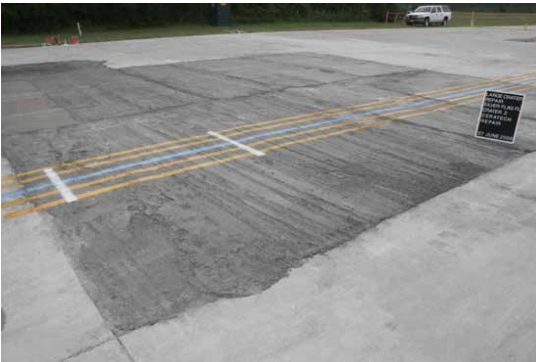
Figure 74. Final surface of the Pavemend EX-H repair for Crater 2.
