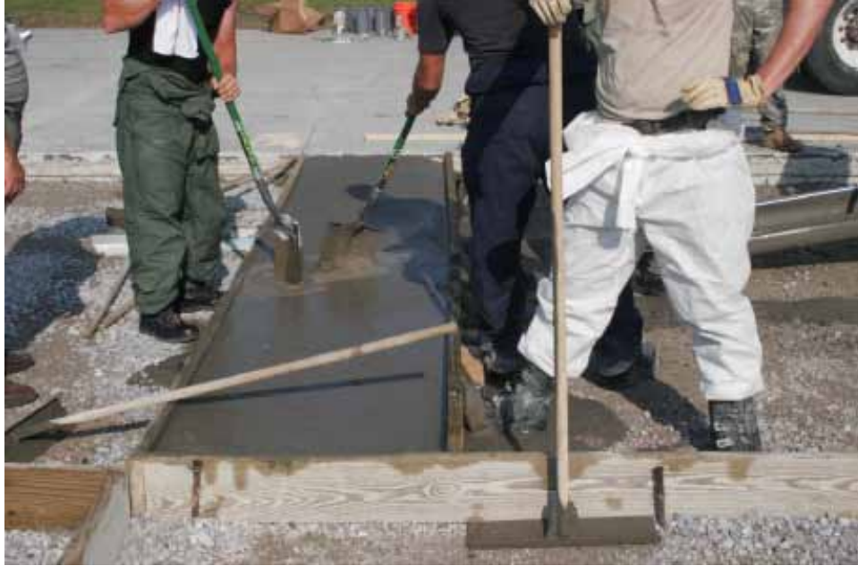
Figure 58. Holding the temporary formboard in place in Crater 5.
