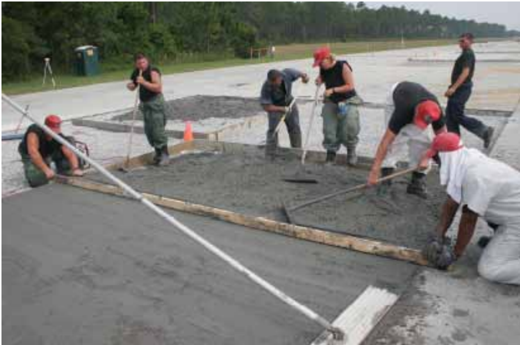
Figure 70. Screeding and floating the southeastern quadrant of Crater 2.
