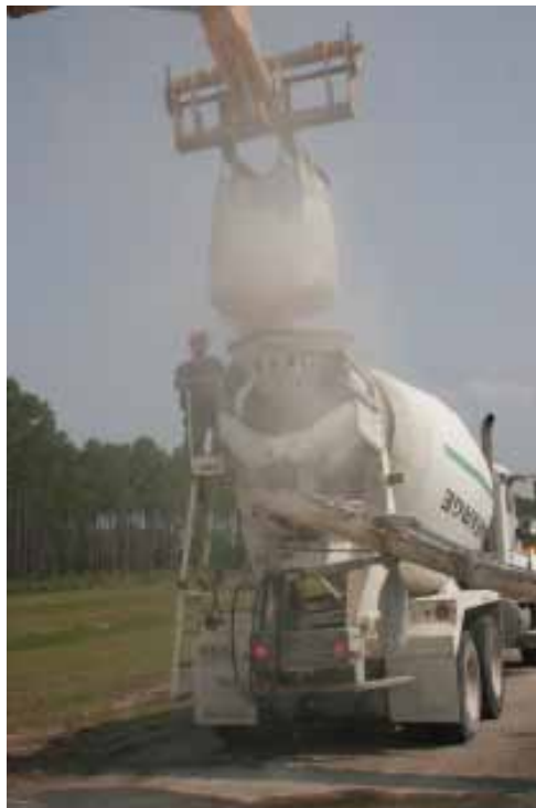
Figure 92. Adding Aquacrete to truck for Crater 3.
