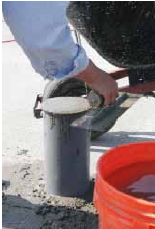
Figure 98. Casting strength cylinders during the full-scale field trial.
