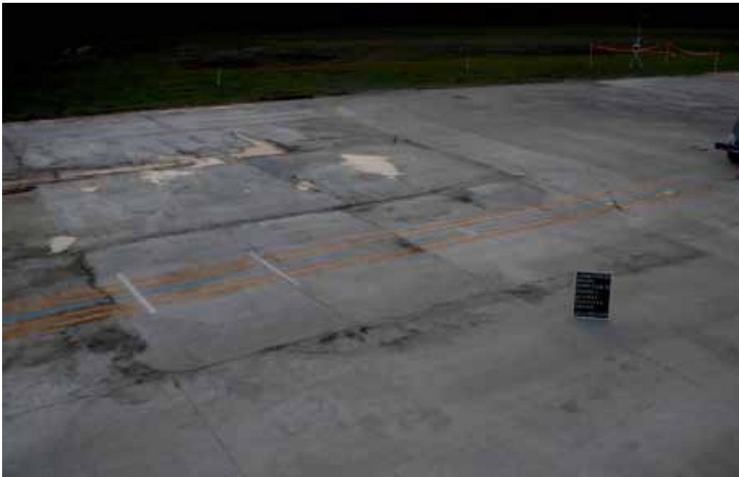
Figure 87. View of the completed repair in Crater 4.
