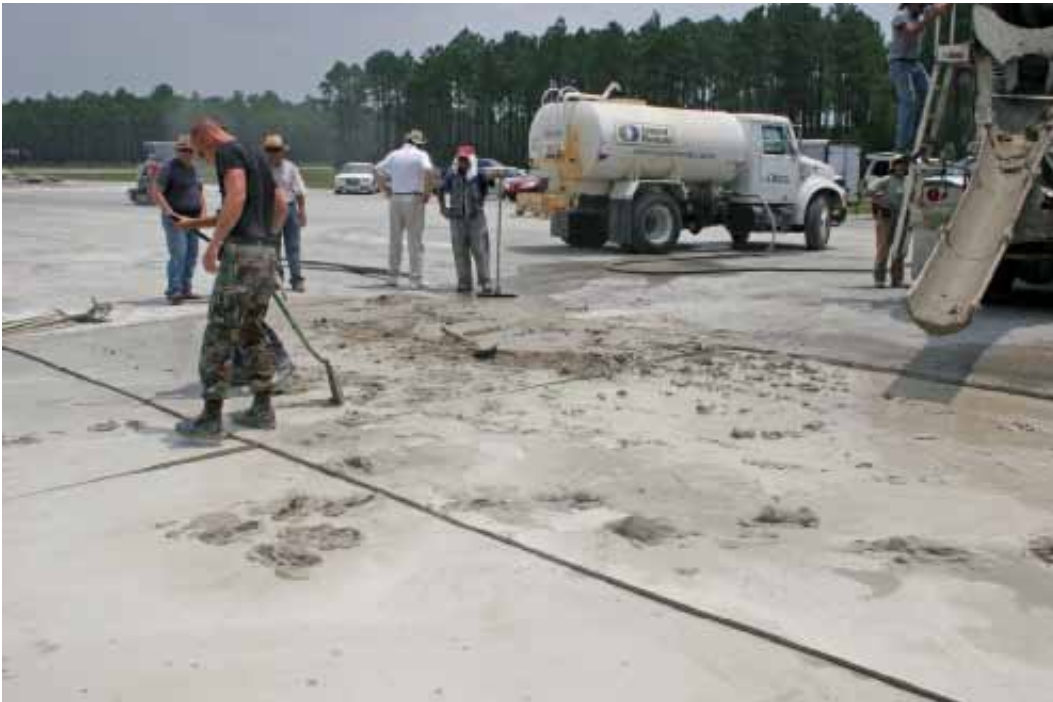
Figure 97. Final Crater 3 repair surface.
