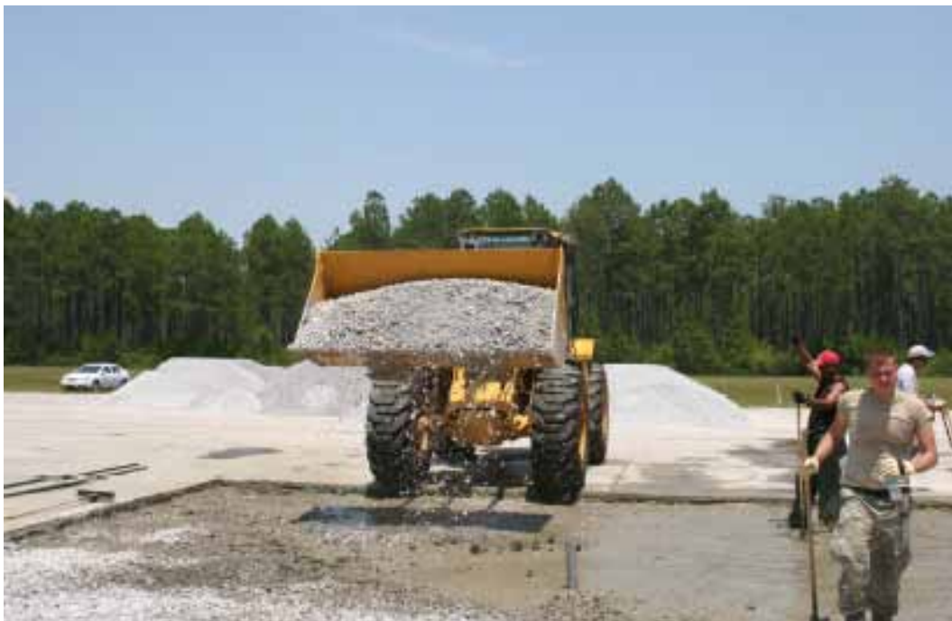
Figure 31. Adding stone to grout layer in Crater 1.
