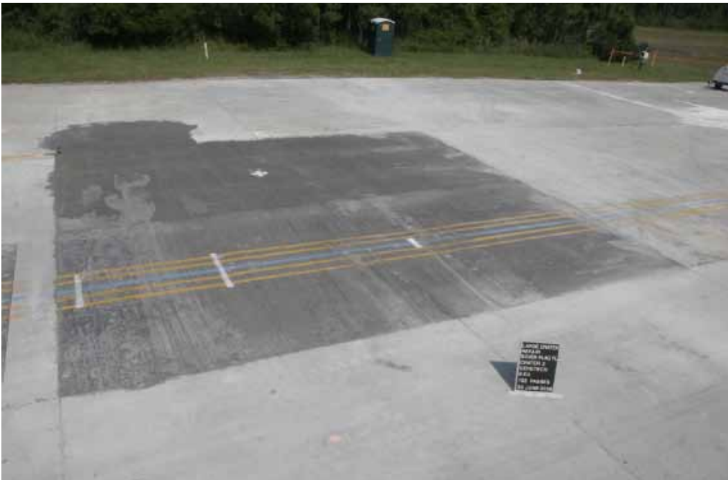
Figure 136. Crater 2, Pavement EX-H after 102 passes of load cart.
