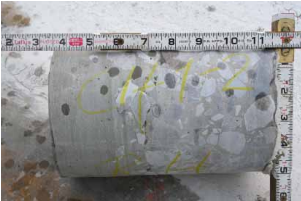
Figure 170. Core 2 from Crater 1 above pressure cell in traffic lane, stone and grout (control).
