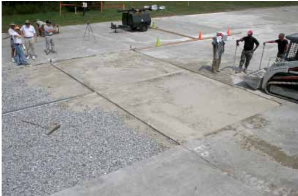
Figure 94. View of Crater 3 following first batch of Aquacrete.
