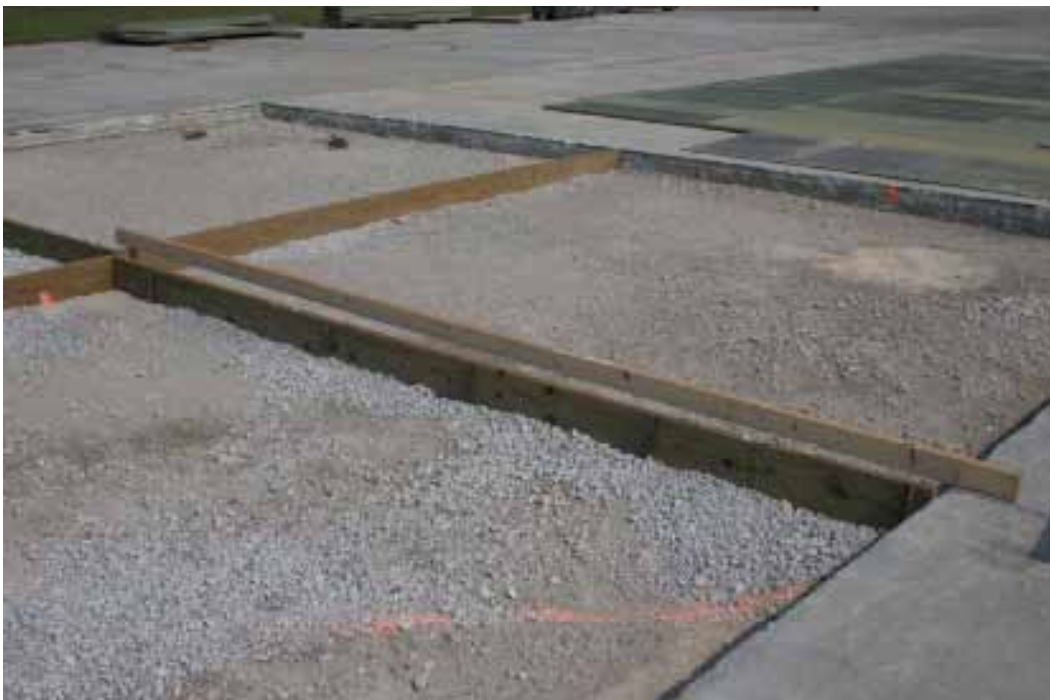
Figure 42. Formwork prepared for Crater 6.
