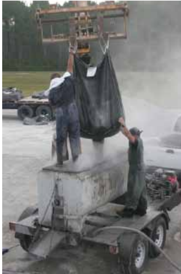
Figure 68. Adding Pavemend EX-H to the mixer for Batch 4 for Crater 2.
