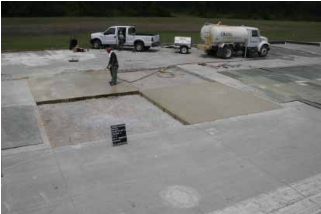
Figure 46. Water was applied to southwestern section, to aid curing, after completion of northeastern section of Crater 6.
