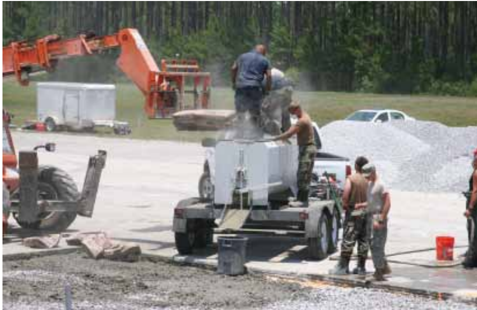
Figure 30. Crater 1 repair resumed following repair of hydraulic leak.
