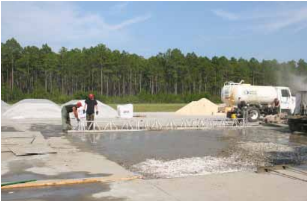
Figure 34. Setting up truss screed on east side of Crater 1.
