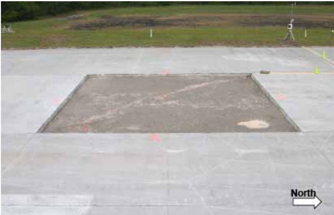
Figure 23. Crater 5 prior to cap placement.
