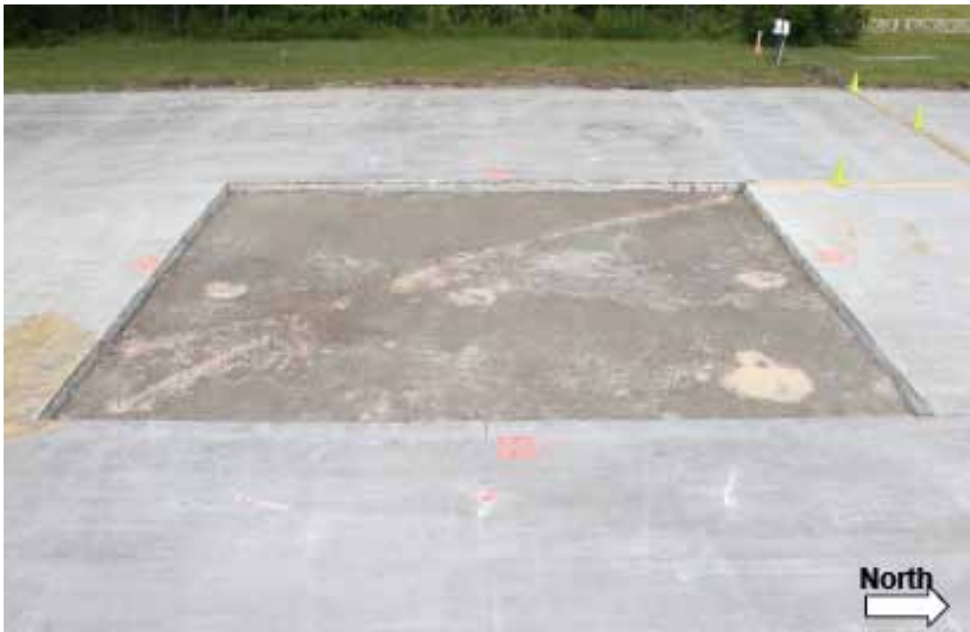
Figure 21. Crater 3 prior to cap placement.
