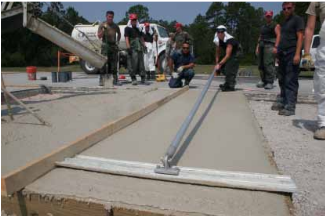
Figure 45. The surface of Crater 6 was screeded and finished.
