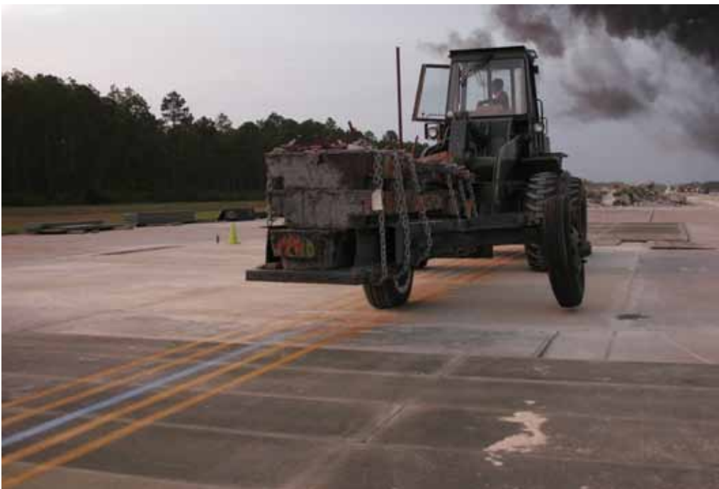
Figure 49. Crater 6, completed repair surface during trafficking.
