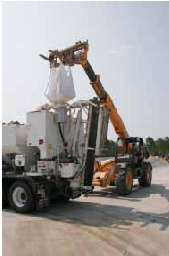
Figure 43. Filling the proportional mixer with Rapid Set DOT cement for Crater 6.
