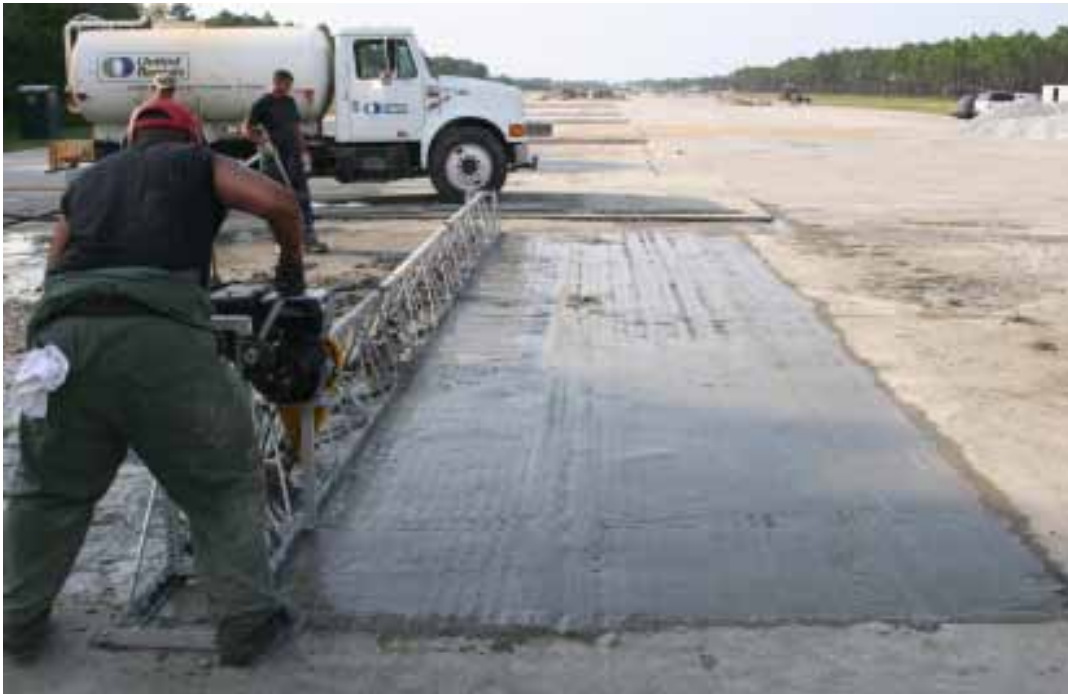
Figure 35. Crater 1, screeding the repair.
