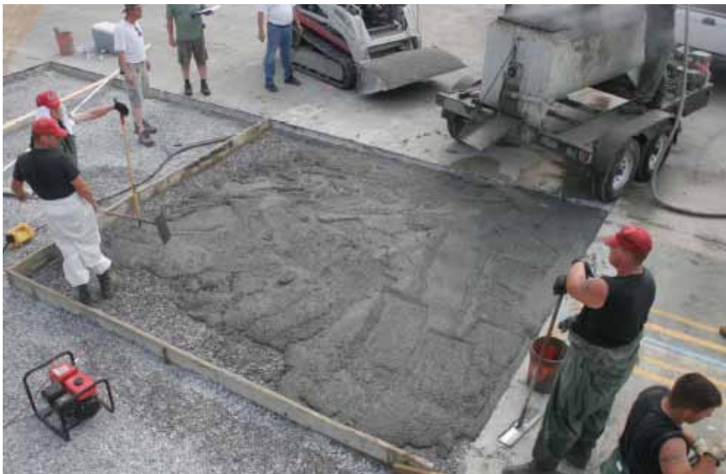
Figure 69. Southeastern quadrant of Crater 2 after placing two batches of material.
