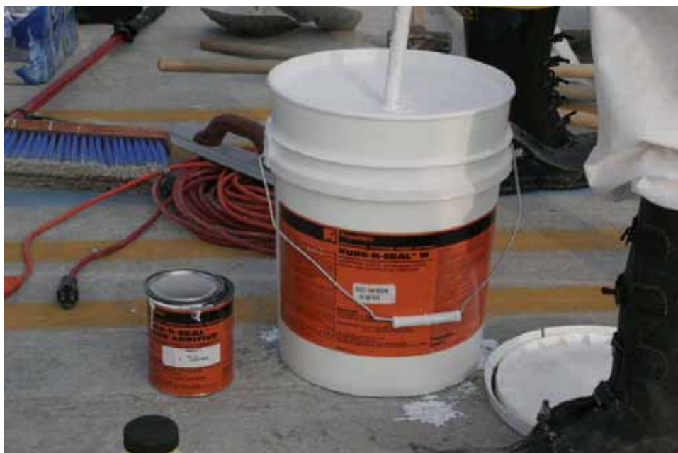
Figure 55. Preparation of curing compound used on Crater 5.
