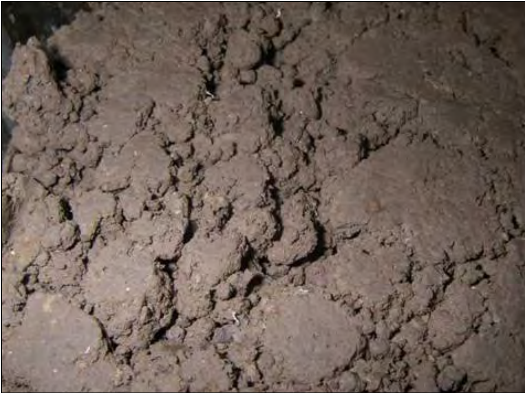
Figure 11. Surface of compacted soil layer after half the required hammer blows.
