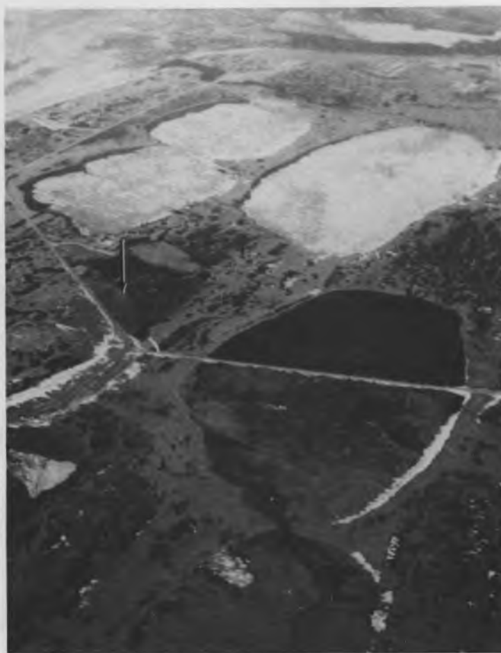
Figure 28. Flooding in a drained lake basin along a road in the Prudhoe Bay region. The photo was taken in early summer before the ice in the culverts thawed. By late summer the large semicircular impoundment drained, but the vegetation became noticeably greener in this area. Also note the other impoundments along the road leading into the background. The largest of these (arrow) does not drain all summer. (Photo by L. Klinger, 21 June 1982.)
