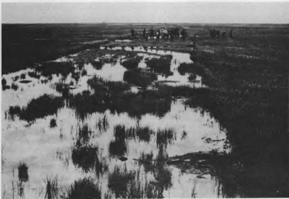
Figure 27. Early gravel road constructed in the late 1960s with insufficient gravel to prevent thermokarst. In places the road surface has subsided to the original ground level. (Photo by K.R. Everett, July 1983.)
