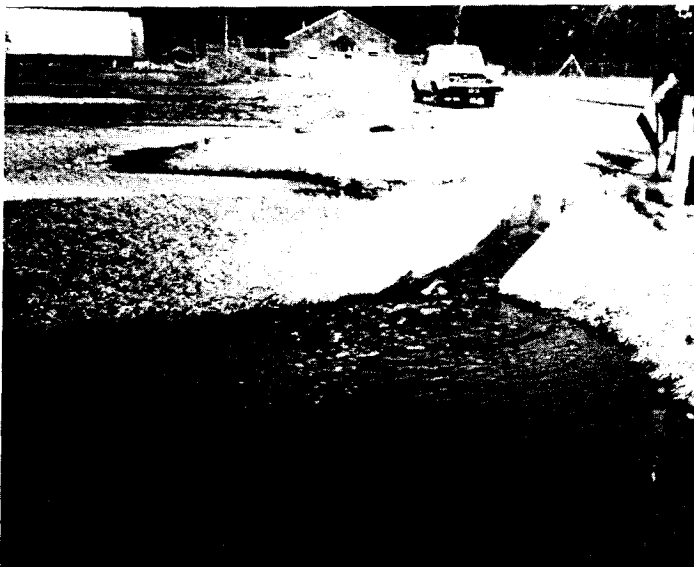
a. Sludge flowing into bed 4.
