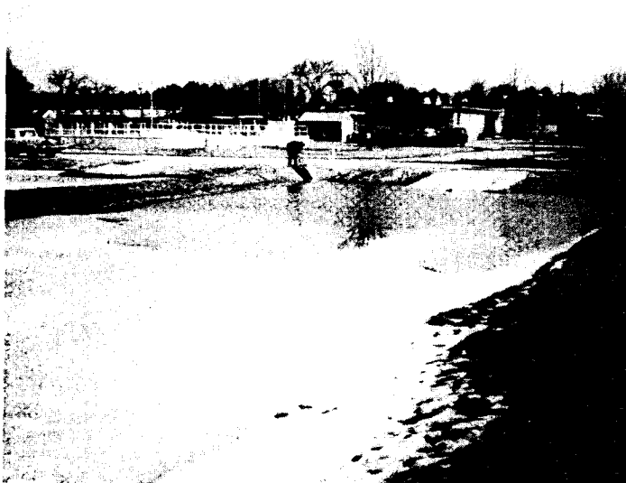
b. Sludge spreading over previously frozen layer.
