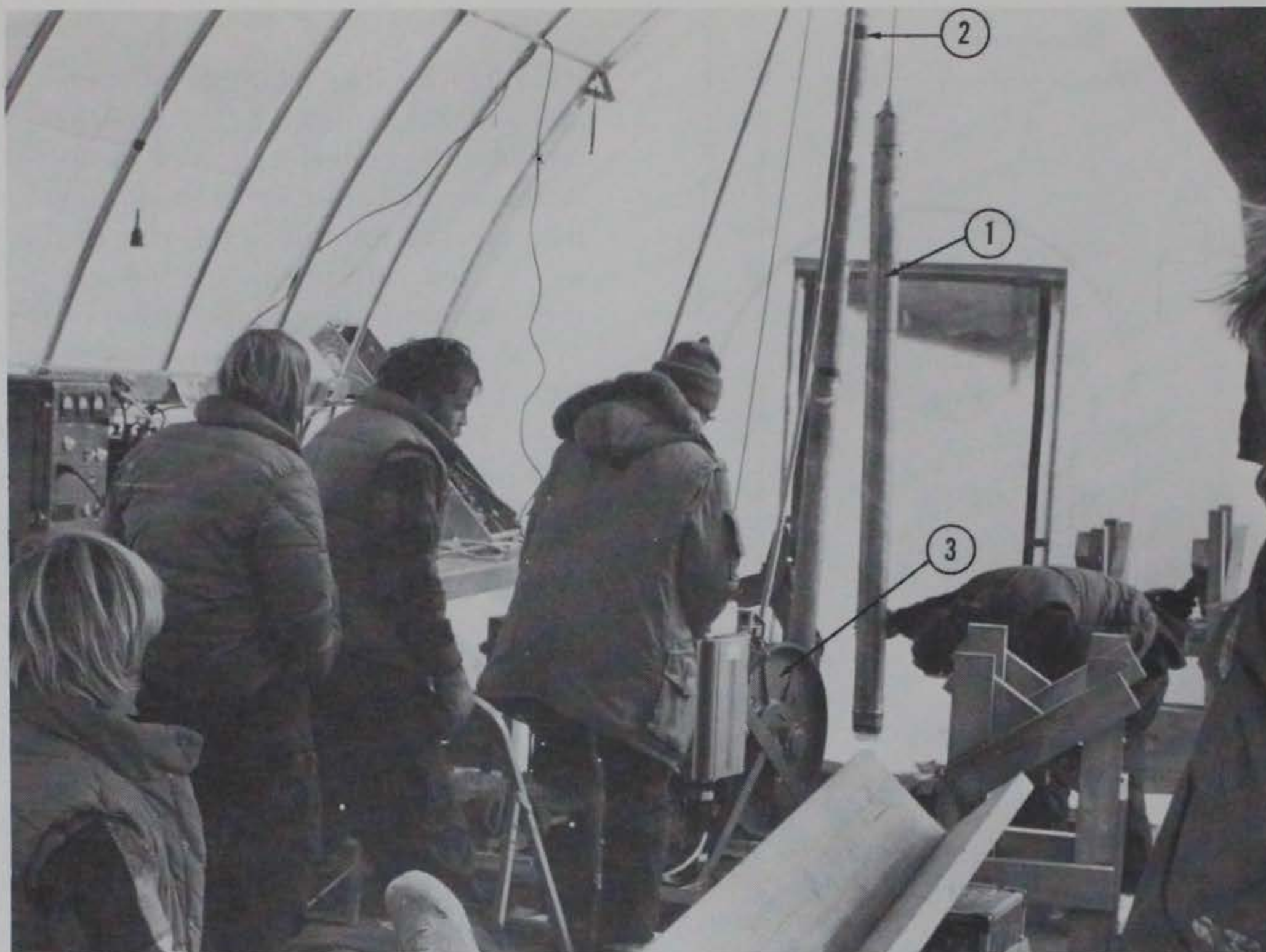
Figure 3. Drilling of antifreeze core hole at J-9 (1. drilling column; 2. mast; 3. winch.)
