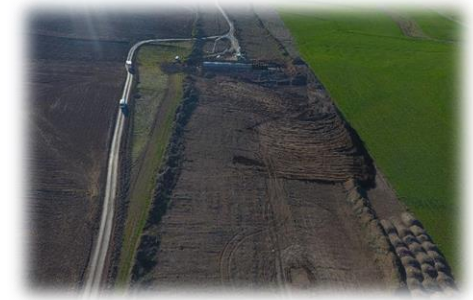
Site After Backfilling
