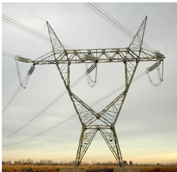
Figure 4.7 – Example and schematics of typical self-supporting suspension tower
