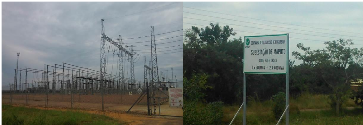
Photograph 6.5 – Aspects of the landscaping in the Maputo (Boane) substation
