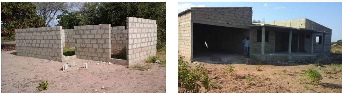
Photograph 6.37 – Houses under construction within the Project RoW
