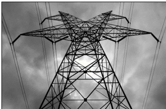
Figure 4.7 – Example and schematics of typical self-supporting suspension tower
