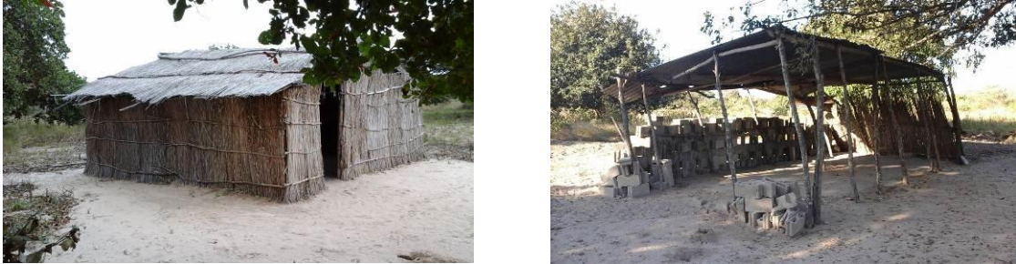
Photograph 6.31 – Zion churches located within the Project RoW (Moamba District)
