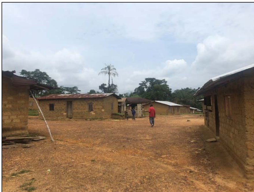
Figure 28: Residential structures in Gehwee town.
