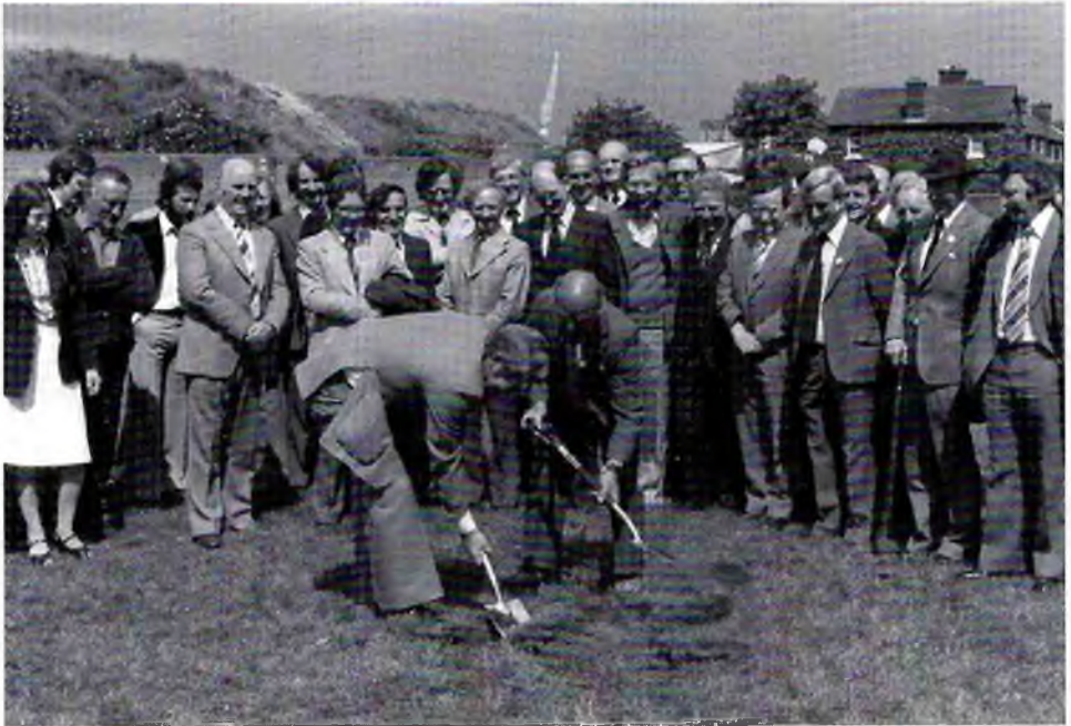
Paddy turning the sod for Sportsco facility with Jimmy D'Art, ESB Poolbeg, Dublin, 8 th June, 1977
