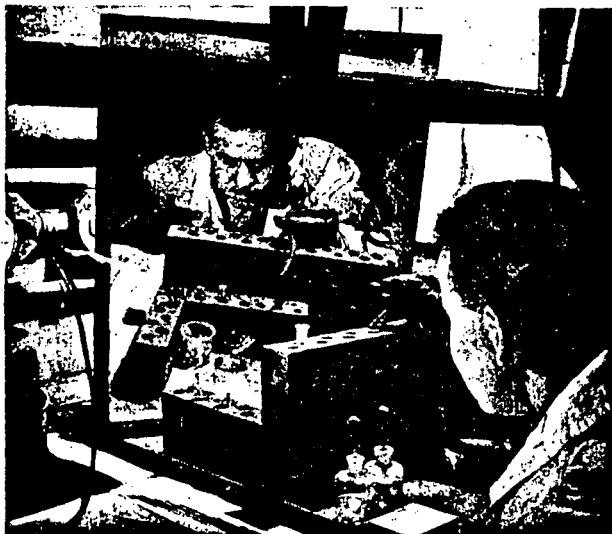
IN TRACER EXPERIMENT Chemist Stanley Thompson, watching his work in a mirror while protected by lead bricks, adds one solution to another which contains a radioactive element. A solid compound then precipitates, or settles, out of the solutions.
