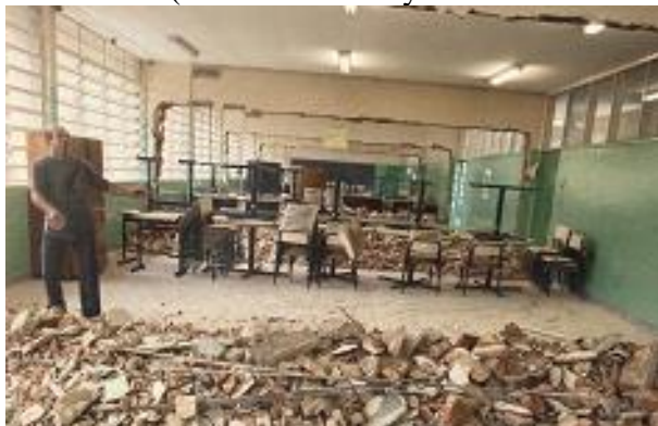
Historical picture depicting the former principal Braz Nogueira and the demolition of internal classroom walls. This photograph was captured from a mural on the history of the Bairro Educador (Educational Neighborhood) at the CEU Heliópolis complex.
