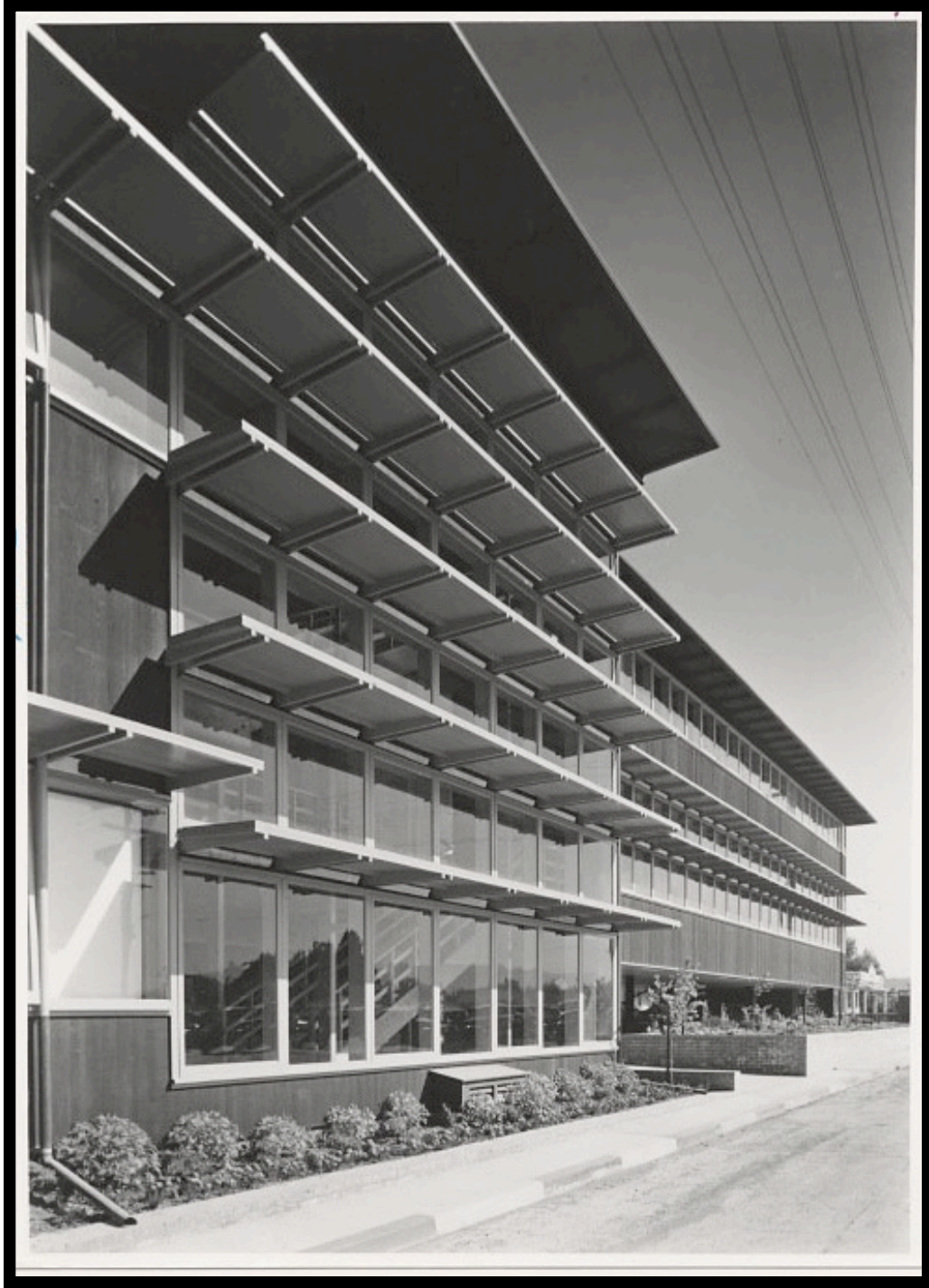
Figure 5.2: Wurster's offices for the Schuckl Canning Company in 1942 exemplify his regional modernist approach, this time in the corporate office setting. Redwood is blended with a toned-down modernist facade. William Wurster architect. Source: Roger Sturtevant, photographer, William W. Wurster/Wurster, Bernardi & Emmons Collection, 1922-1974, Environmental Design Archives. College of Environmental Design. University of California, Berkeley.
