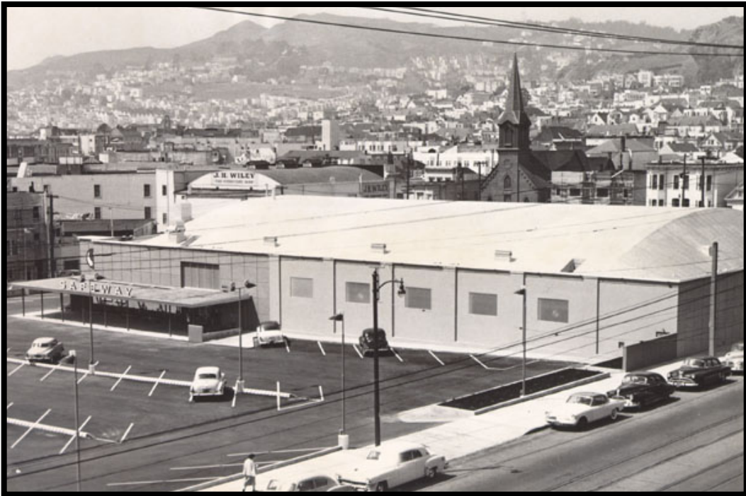
Figure 5.26, 5.27: Two examples of the industrial domed Safeways with more traditional fronts: Duboce and Market, San Francisco, 1954 and Walnut Creek California, 1955. Source: Safeway News ; San Francisco History Center, San Francisco Public Library.
