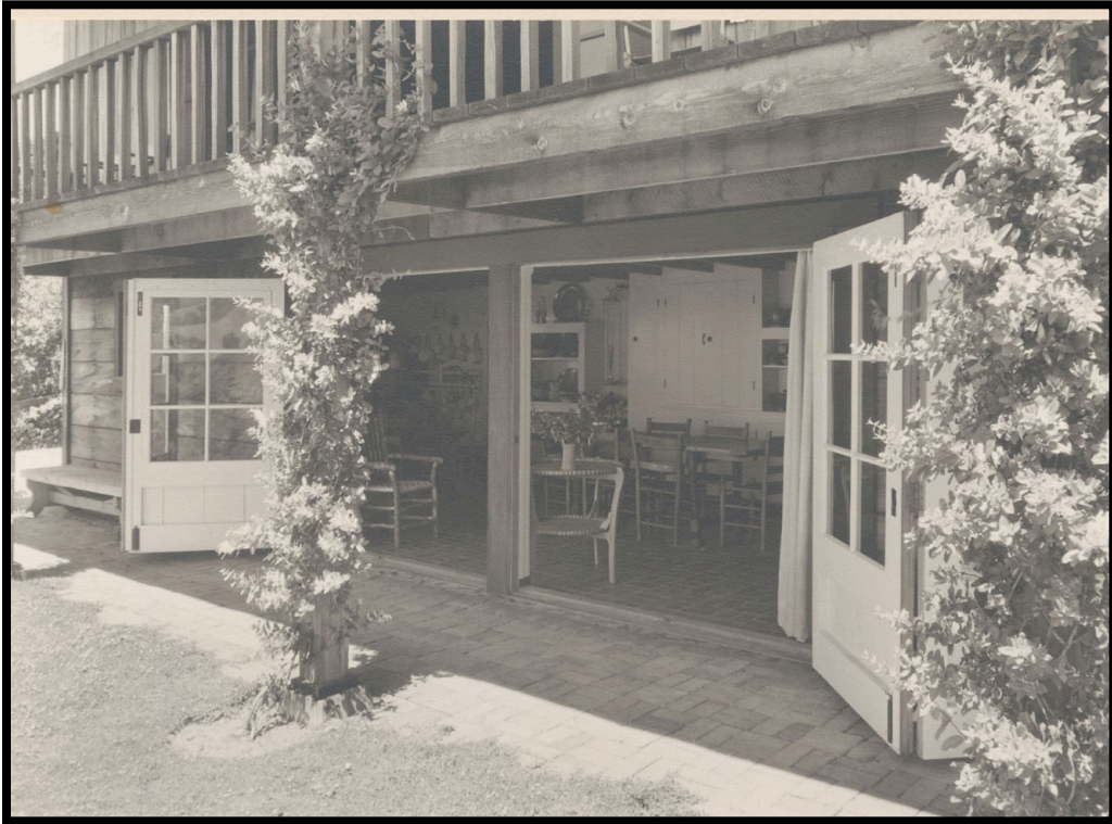
Figure 2.11: Indoor-outdoor relationship shown by the Carl L. Voss Residence, Big Sur, CA, William Wurster architect, 1931. Source: Roger Sturtevant, Photographer, William W. Wurster/Wurster, Bernardi & Emmons Collection, 1922-1974, Environmental Design Archives, University of California , Berkeley, California.
