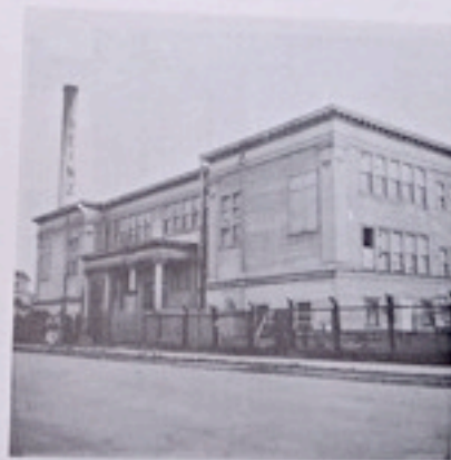
HEINZ STREET . . . . . STRUCTURALLY SOUND, THEREFORE NOT A BLIGHT? HOW CAN YOU GET PEOPLE TO FIX UP THEIR HOMES WHEN AN UGLY DILAPIDATED SIGHT SUCH AS THIS IS RIGHT OUTSIDE THE FRONT DOOR?
