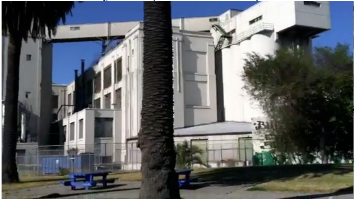
Fig. 7 Park Adjacent to Industrial Facility
