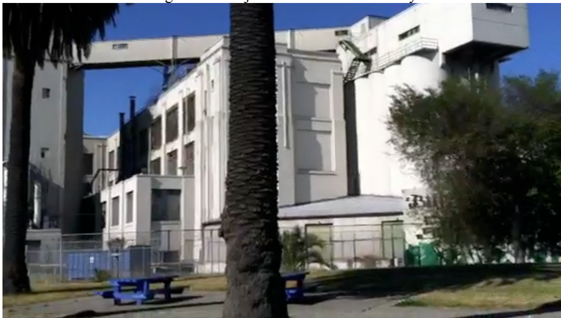
Fig. 7 Park Adjacent to Industrial Facility
