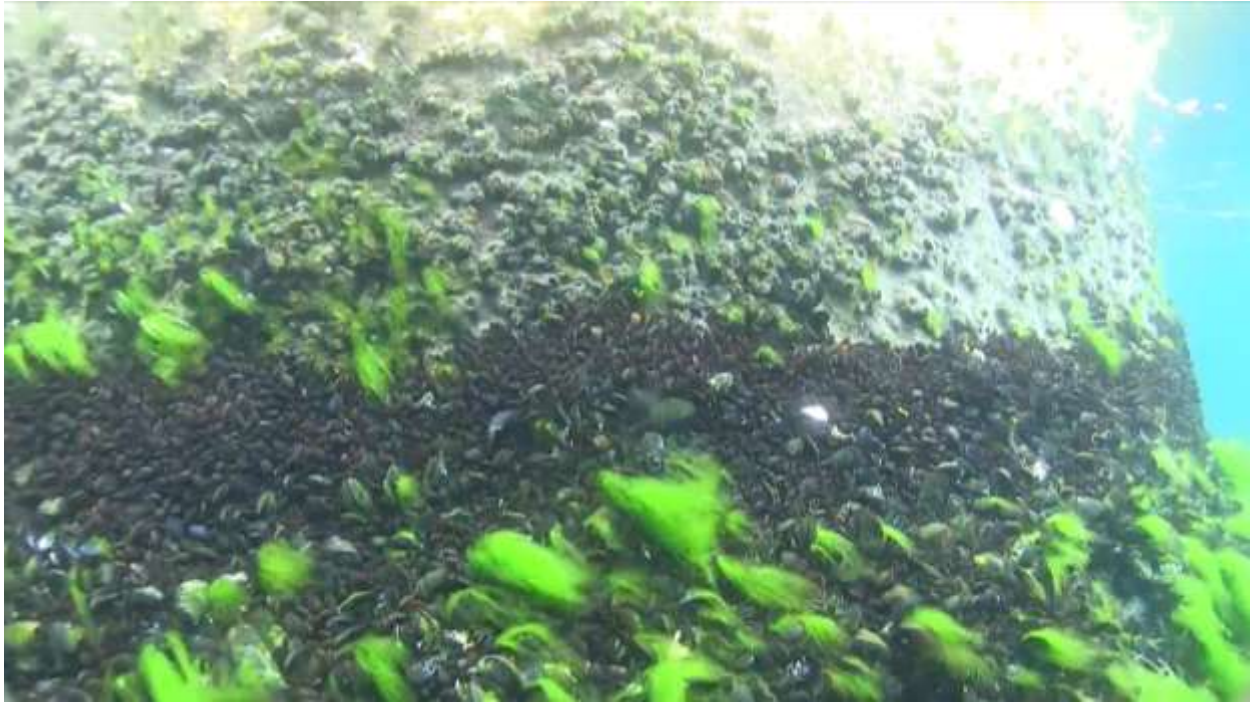
Figure L-3-1. Intertidal zone of the BIWF jacket foundation showing barnacle ( Balanus sp.), mussel ( Mytilus edulis ) and green algae.
