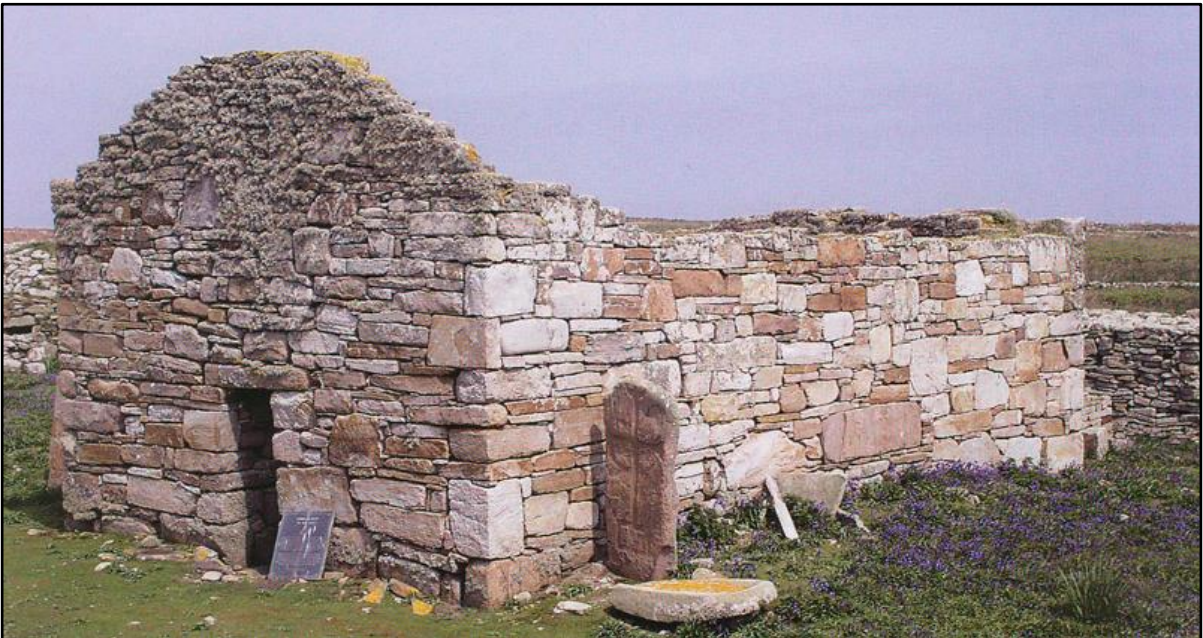
Figure 4.20: Templemolaise, Inishmurray. (Reproduced from O'Sullivan and Ó Carragáin, Inishmurray)
