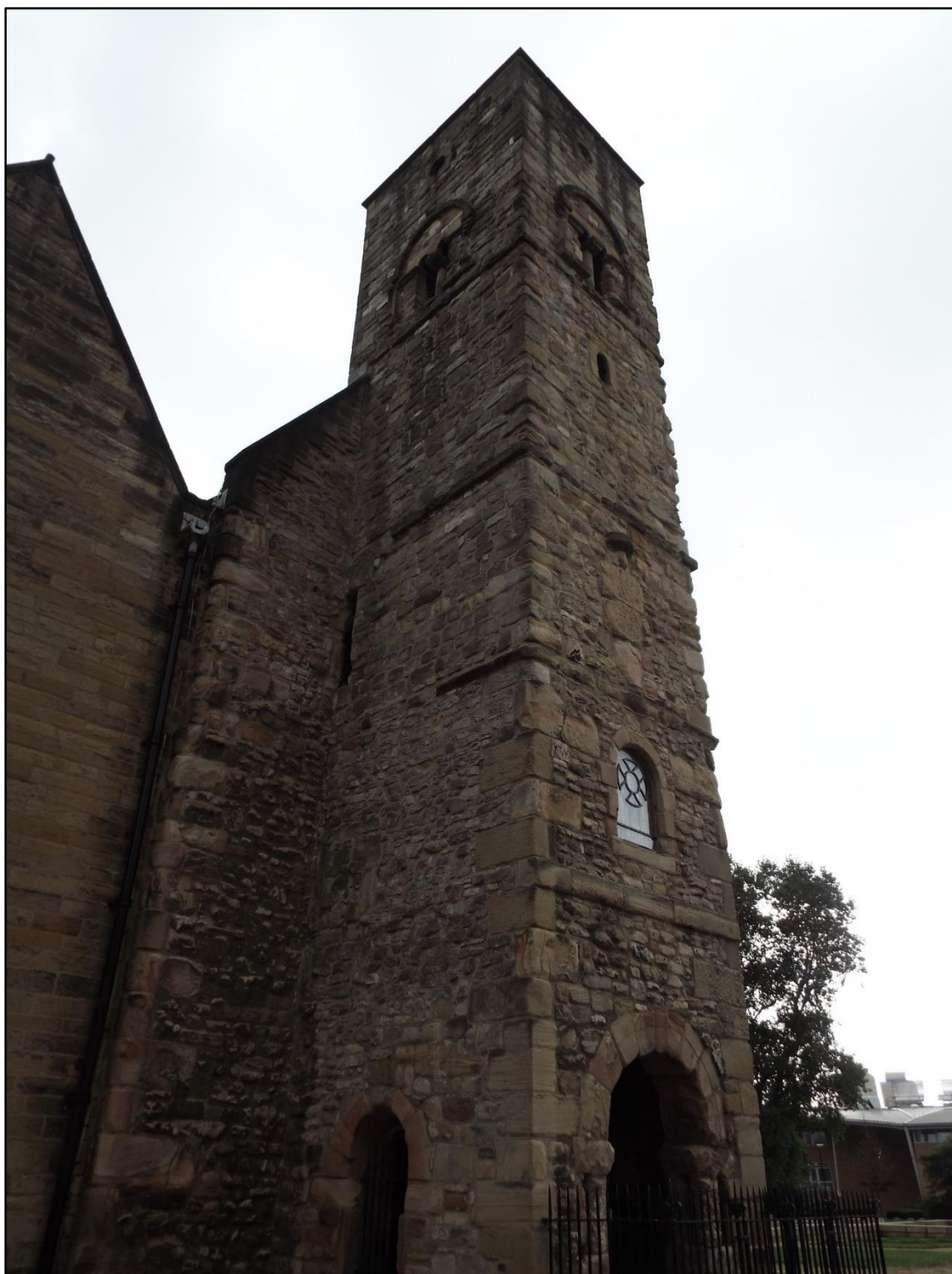
Figure 6.38: The western tower of St Peter's Church, Weymouth. The fabric above the third set of stripwork is of a noticeably different construction, indicating that a much later tower was built on a seventh- or eighth-century porch which featured a relief of a human figure, now greatly weathered. (Photo by Ross McIntire)
