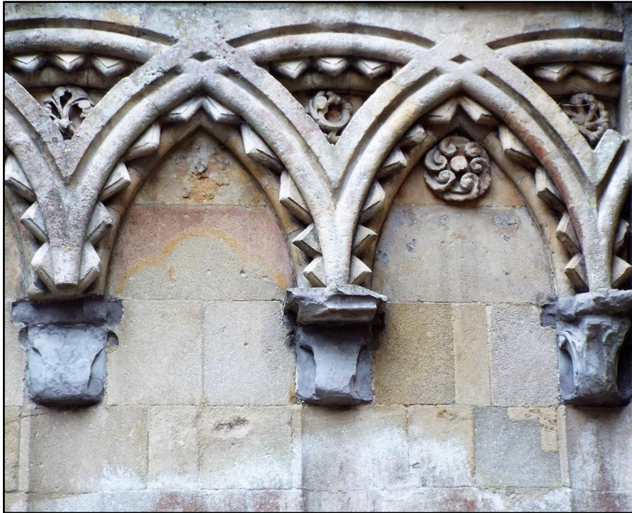
Figure 7.6: Detail, Lady Chapel blind arcading, south interior wall. (photo by Ross McIntire)
