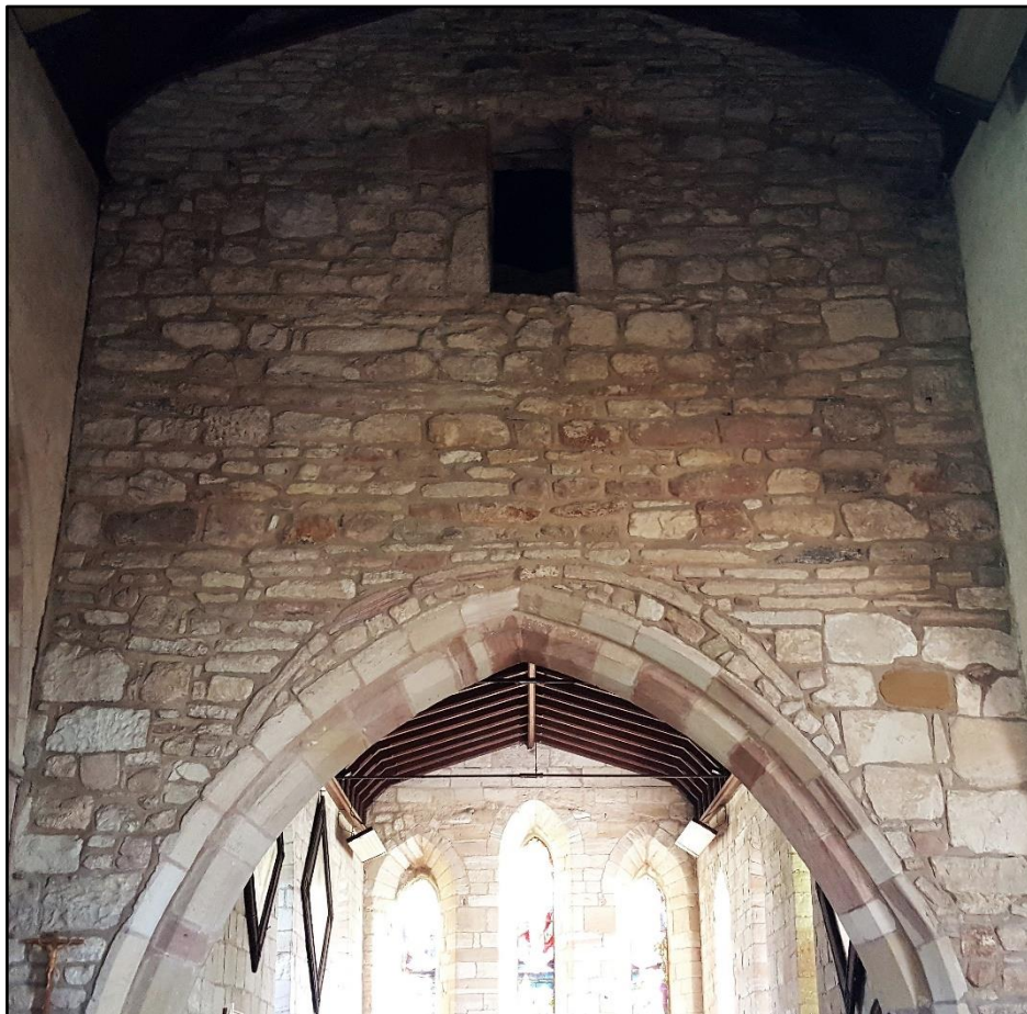
Figure 6.13: The west face of the chancel arch, St Mary's Church, Lindisfarne. The scarring from a previous rounded open can be seen above the 13thc pointed arch. (Photo by Ross McIntire)
