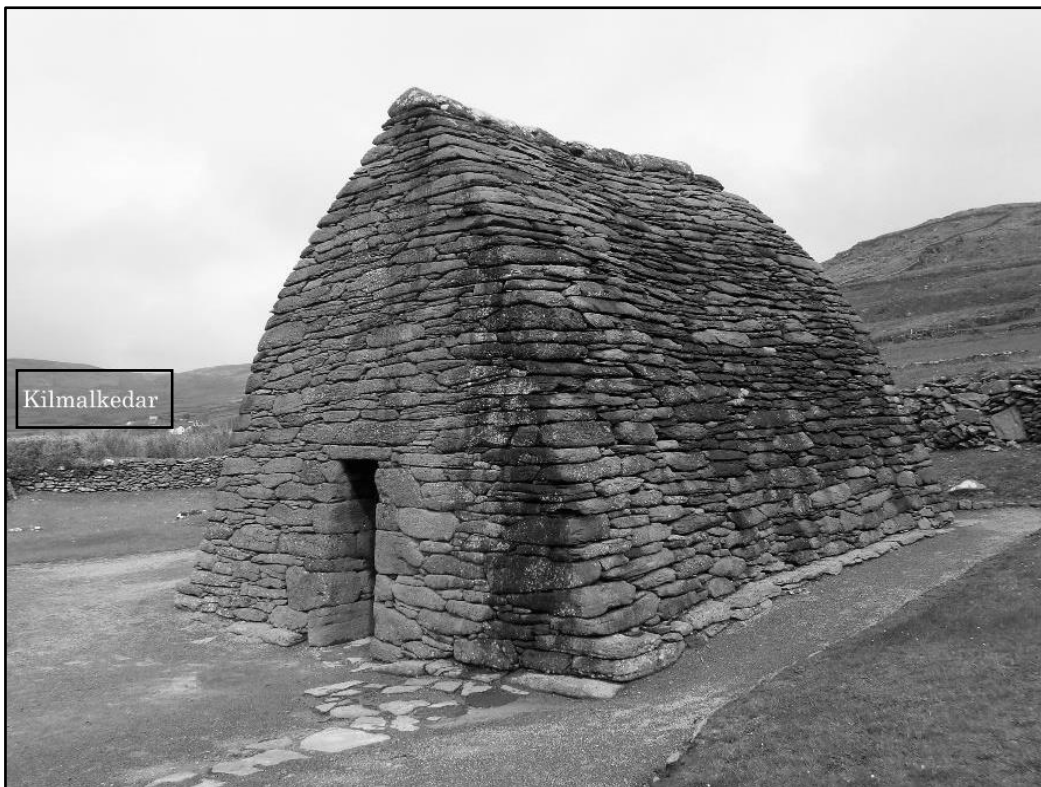
Figure 4.31: Gallarus Oratory, a corbelled building dated to anywhere between the 7 to 11c., looking northeast. Beyond the enclosure the cemetery of Kilmalkedar is visible in the distance. (Photo by Ross McIntire)
