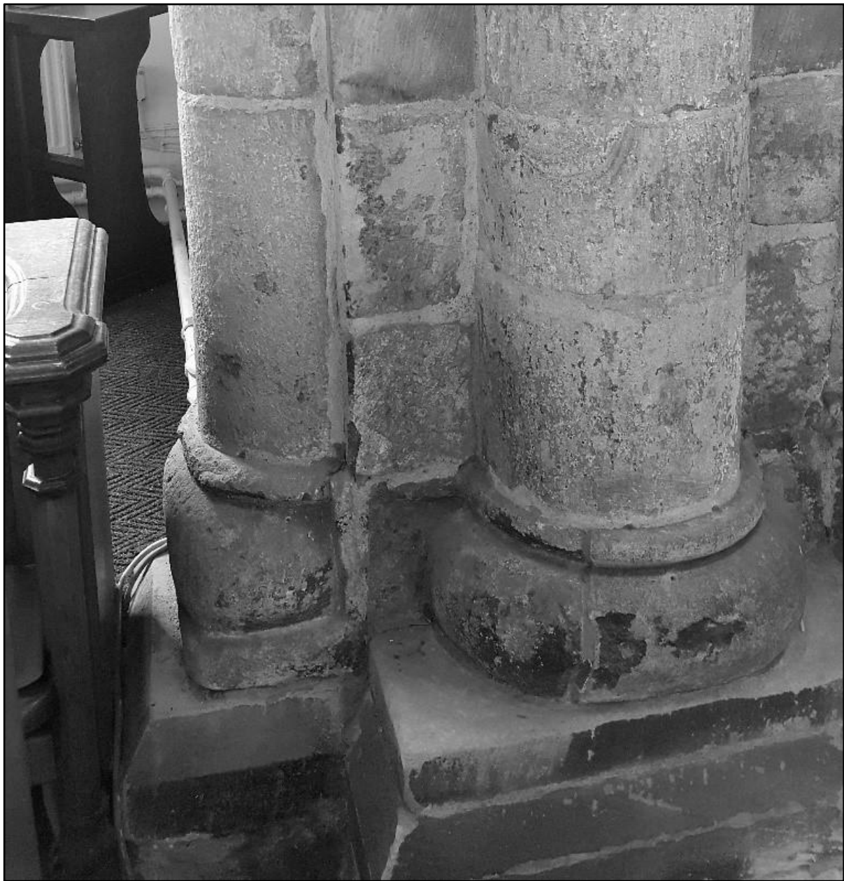
Figure 6.39: Southeast pier of the lost chancel arch, possibly eleventh century. (Photo by Ross McIntire)
