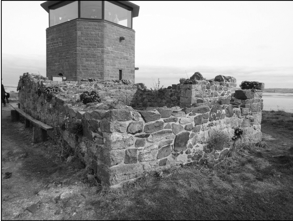
Figure 6.17: The 'Chapel of the Lamp' on the Heugh. The standing ruins to the east of the modern lighthouse are a post-medieval construction, but incorporated pieces of medieval architectural fragments suggested the presence of an earlier building. (Photo by Ross McIntire)
