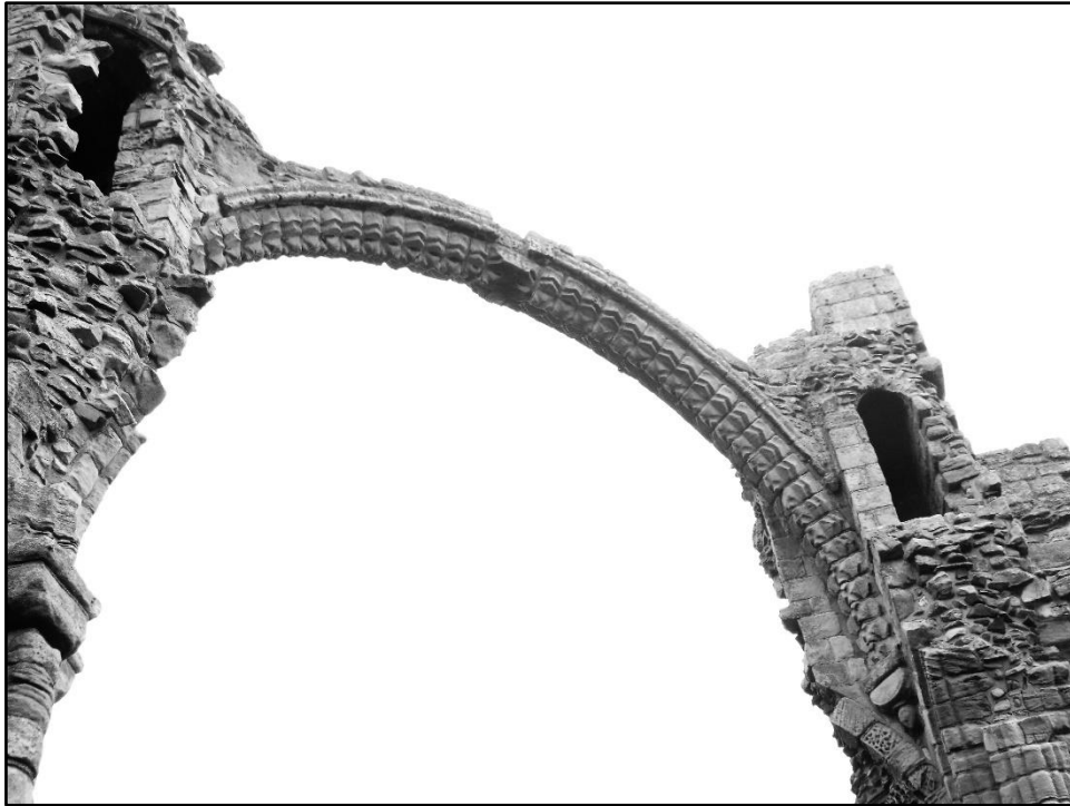
Figure 6.6: The 'hanging rib' between the north-west and south-east piers of the crossing tower, c.1150. (Photo by Ross McIntire)
