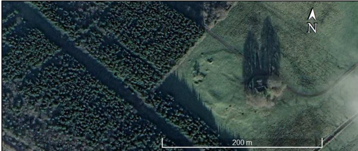
Figure 4.26: Monaincha (Co. Tipperary). While the outline of the original island and later fishponds remain to the west of the monastic church, there is no trace of either the other buildings on the main island or the second island depicted by Ledwich in either modern aerial photos or those number taken in 1966, prior to the forestation of the adjacent land. (Google Earth)
