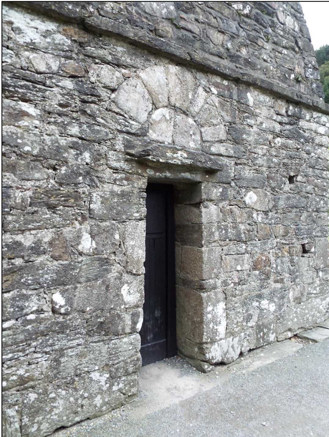
Figure 4.10: The head of a doorway reused in the western entrance to St Kevin's Church. Ó Carragáin argues that this is evidence of a previous stone building on the site, which makes it unique (with the exception of the cathedral) and strengthens the case for it as Kevin's shrine church. (Photo by Ross McIntire)
