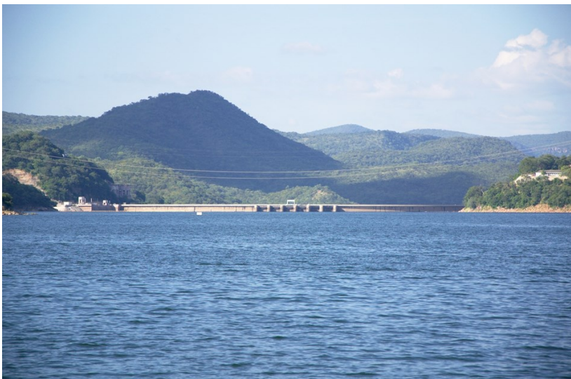
Kariba Dam located along the Zambezi River at the border between Zambia and Zimbabwe.
