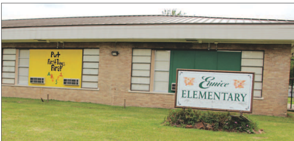
Repairs to a classroom building at Eunice Elementary are complete. (Photo by Myra Miller)
