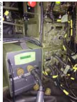
Photo: SFC Energy
