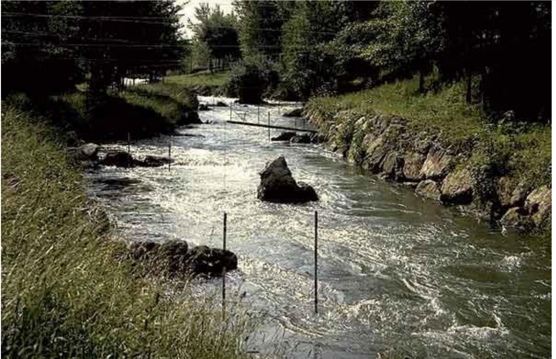
Bypass, Gave de Pau (France) to overcome a 5.5 m high dam (Ravichandran & Semwa, 2016)
