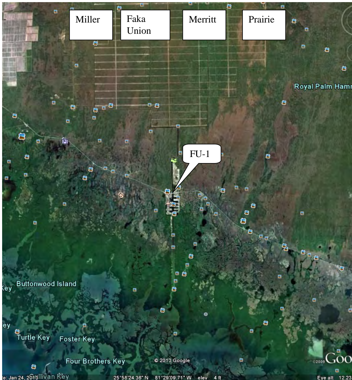
Figure A7-1-10. Picayune Strand Restoration Project area showing drainage canals (top of image) and Faka Union outlet structure (FU-1).
