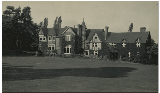
Ivy House, c.1950.
